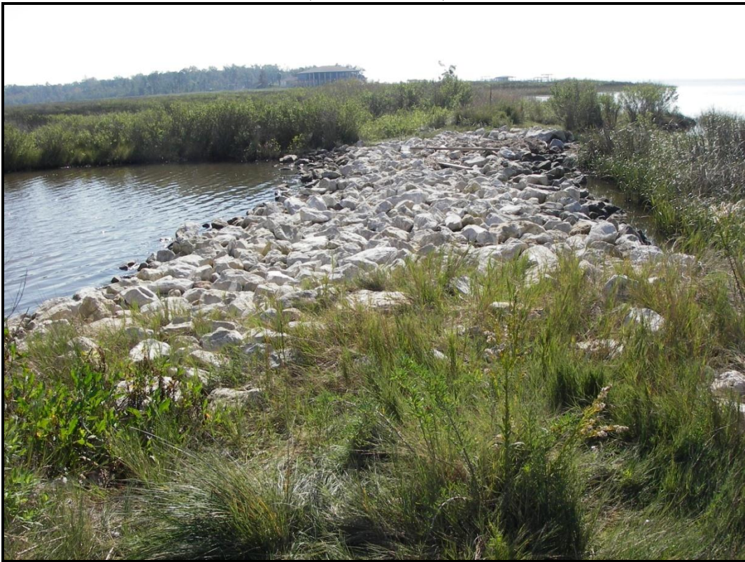
Photo No. 6, Structure No. 8, rock plug showing accretion occurring on lake side.
