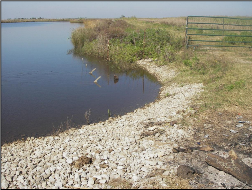
Photo No.3 , Structure No.1, outlet side.
