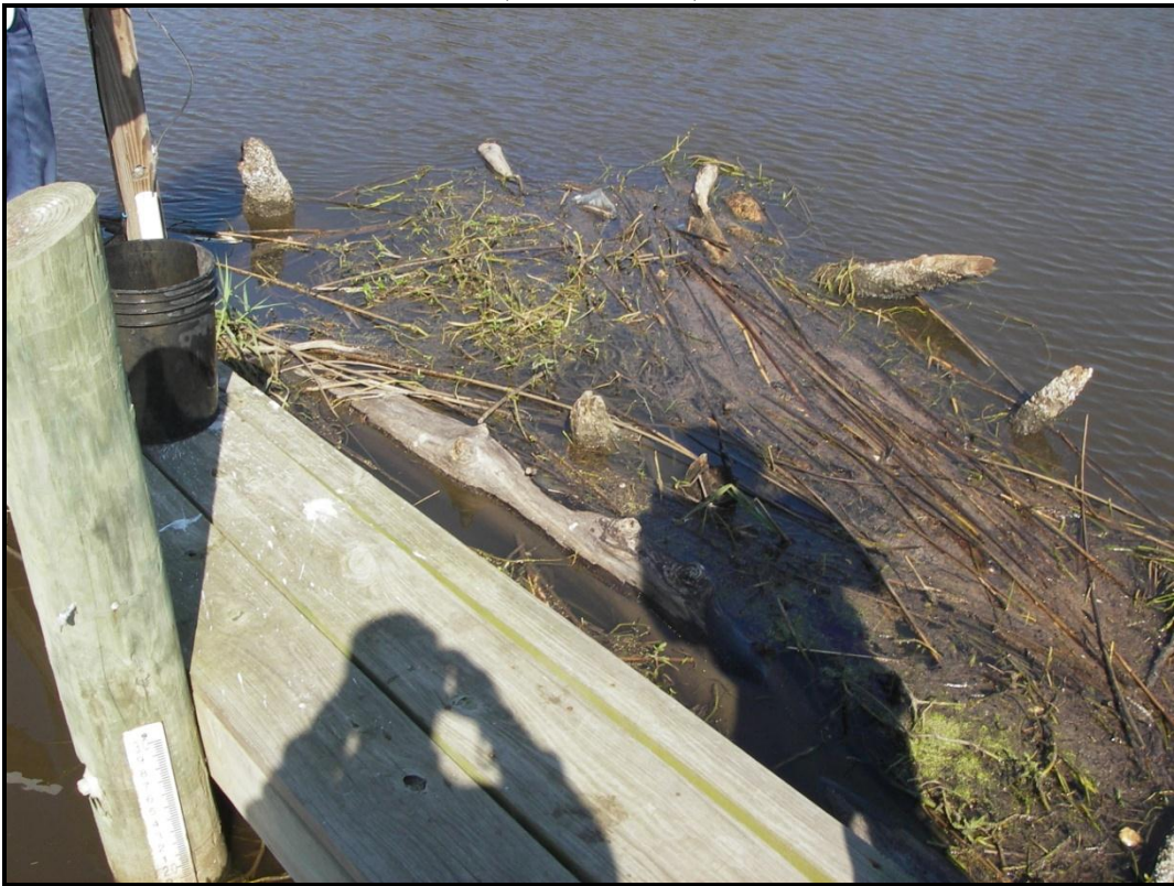
Photo No. 2, Structure No.1, trash along fence.
