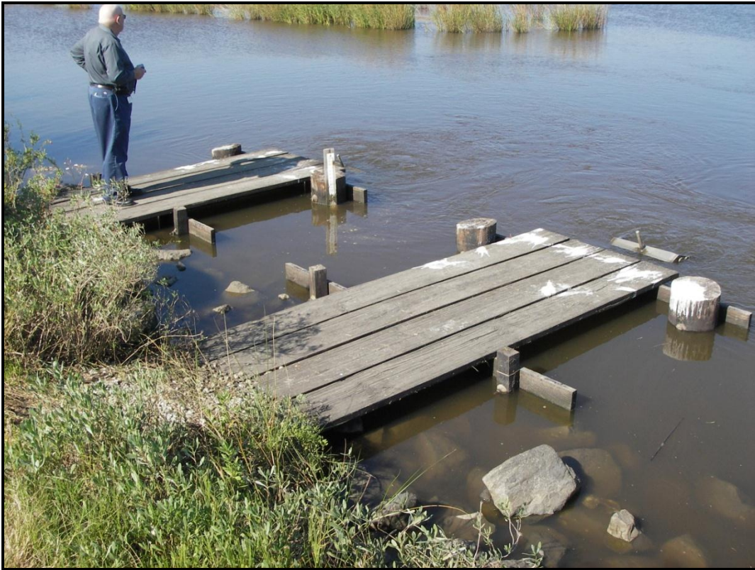
Photo No. 5, Structure No. 12, outlet side.
