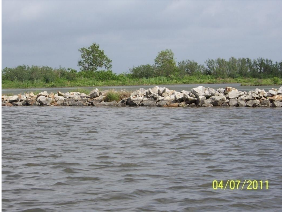
Photo 9: Bayou DeCade Rock Dike and breach closure constructed in 2003, looking north
