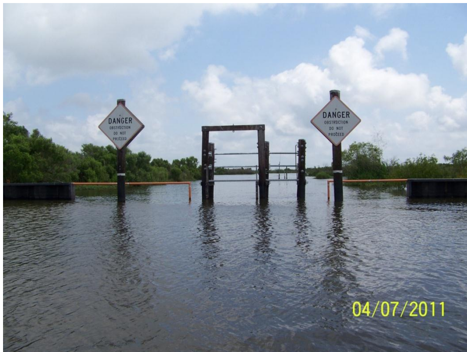
Photo 68: Structure 14 fixed crest weir with variable crest section, looking east
