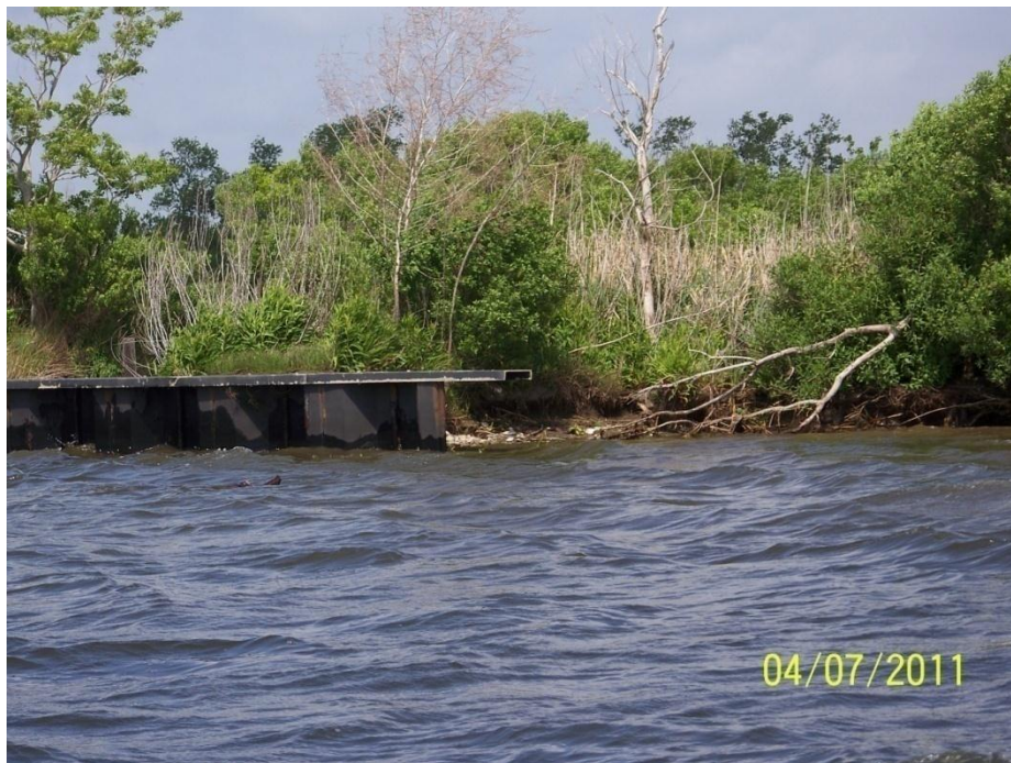
Photo 26: Tie-in erosion on northeast side of Structure 21 causing exposed bulkhead
