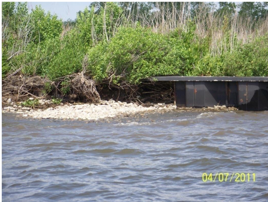
Photo 28: Tie-in erosion on southwest side of Structure 21 causing exposed bulkhead
