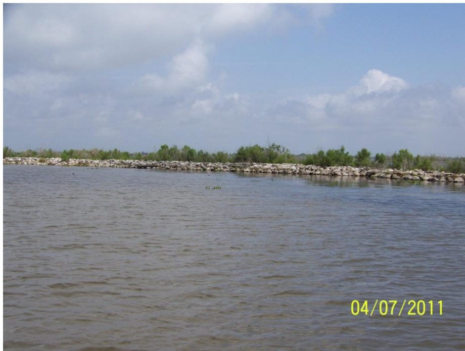
Photo 52: Embankment with rock along Bayou DeCade north shoreline located between Structure 6 and 7
