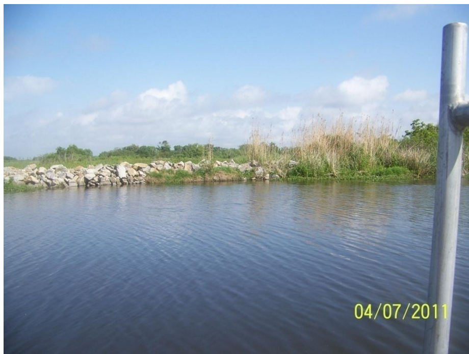
Photo 1: Armored breach repair located in oil field access off Superior Canal, looking northeast
