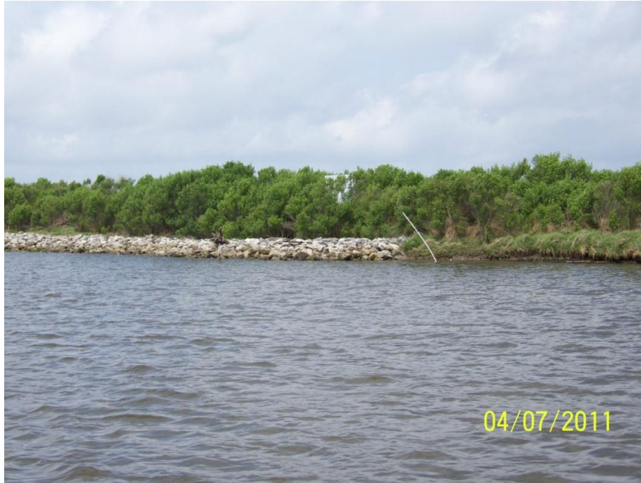
Photo 57: Transition to earthen embankment with rock along north bank of Bayou Decade
