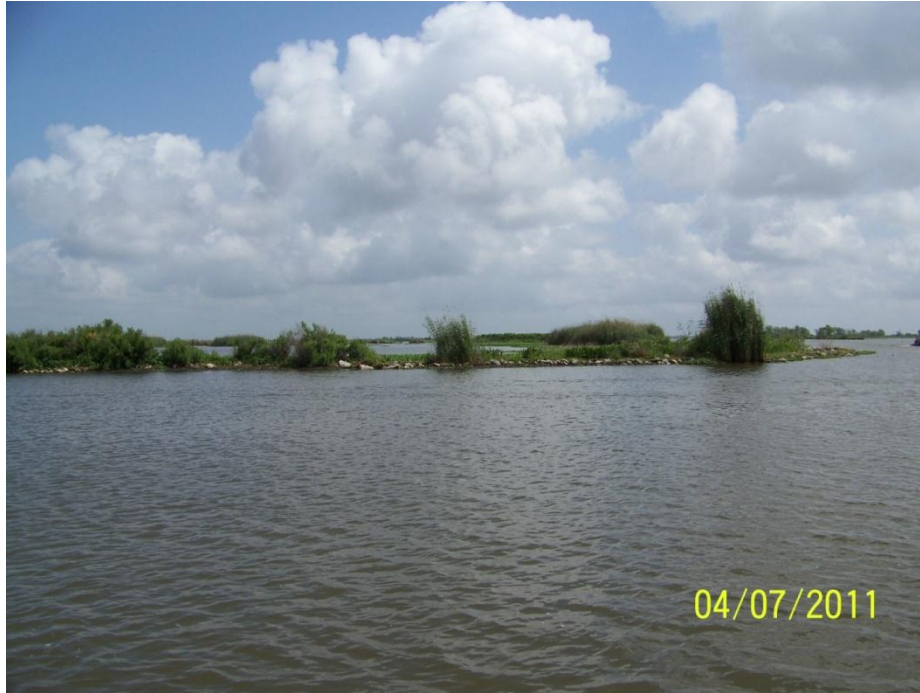
Photo 51: Low area of rock dike along Bayou DeCade north shoreline, located between Structure 6 and 7
