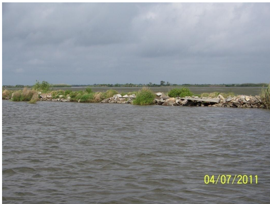
Photo 5: Bayou DeCade Rock Dike and breach closure constructed in 2003, looking north
