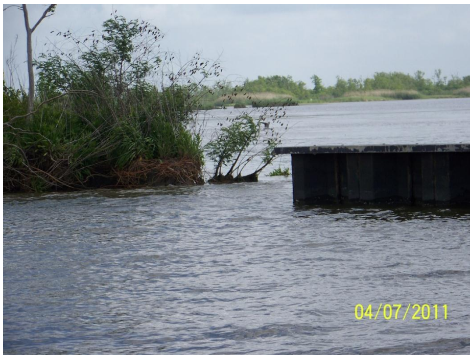
Photo 22: Structure 23 Tie-In Breach on north side of structure, looking east
