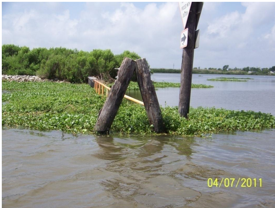
Photo 46: Steel sheetpile weir and timber bumper guards on the west side of the barge bay of Structure No. 6
