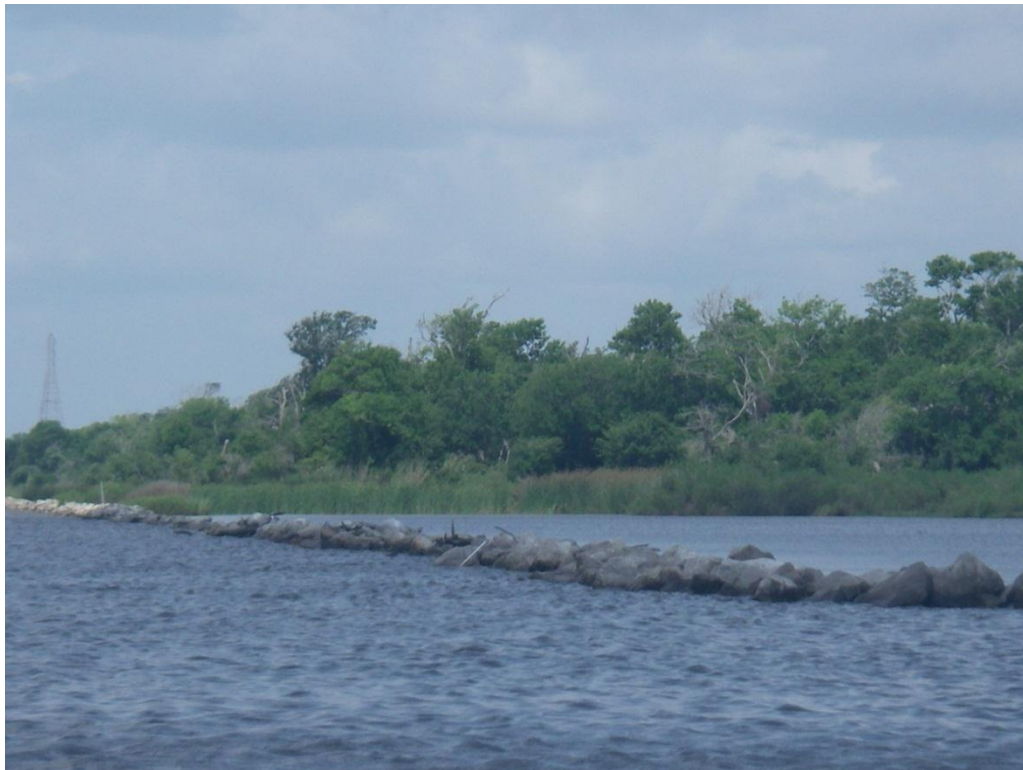
Photo No.2, Accretion behind Rock Dike
