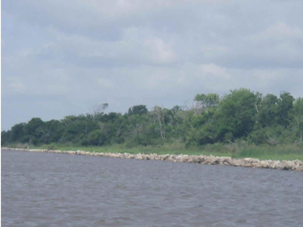
Photo No.3, Vegetation behind Rock Dike
