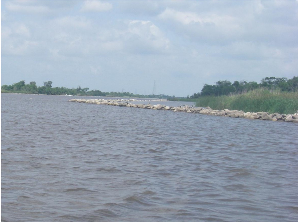
Photo No.1, Typical Rock Dike
