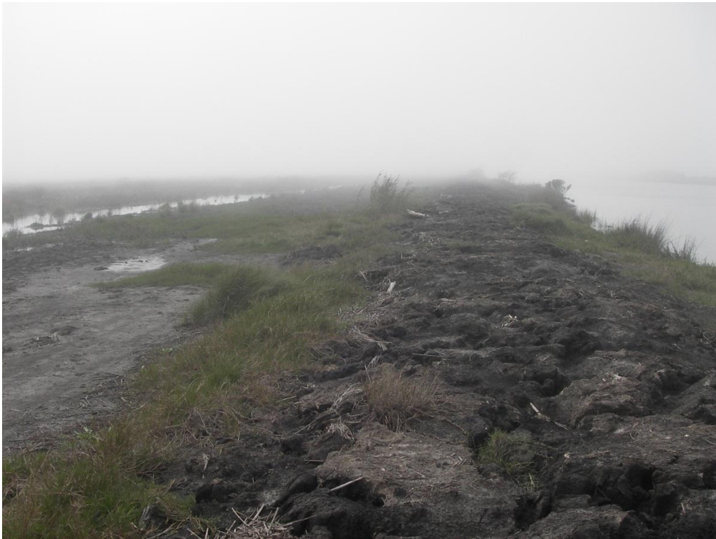
Photo No.2, Containment Dike along Pipeline Canal
