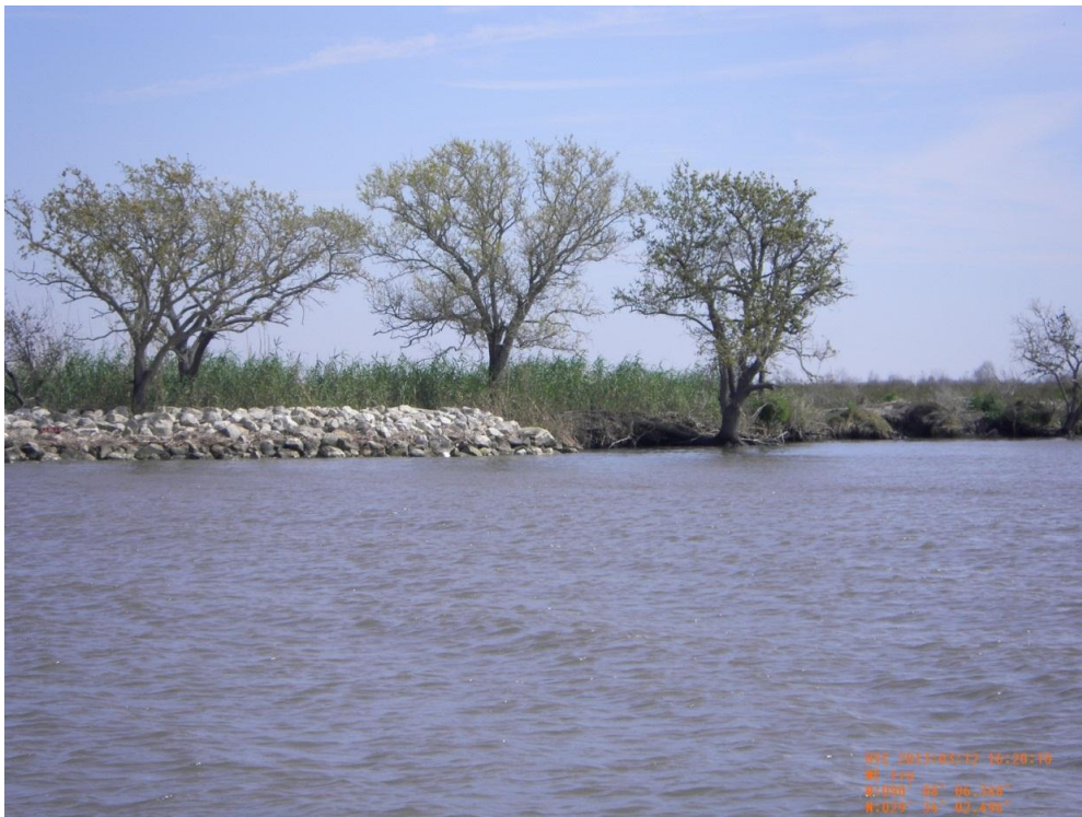
Photo 24: View of the CU#4 rock tie-in on the east side of Harvey Cutoff canal
