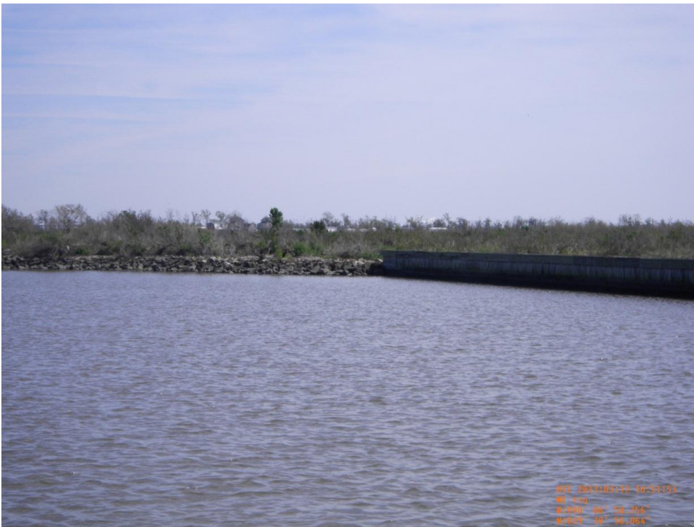
Photo 44: View of intersection of CU#6 rock dike and pipeline timber bulkhead looking east
