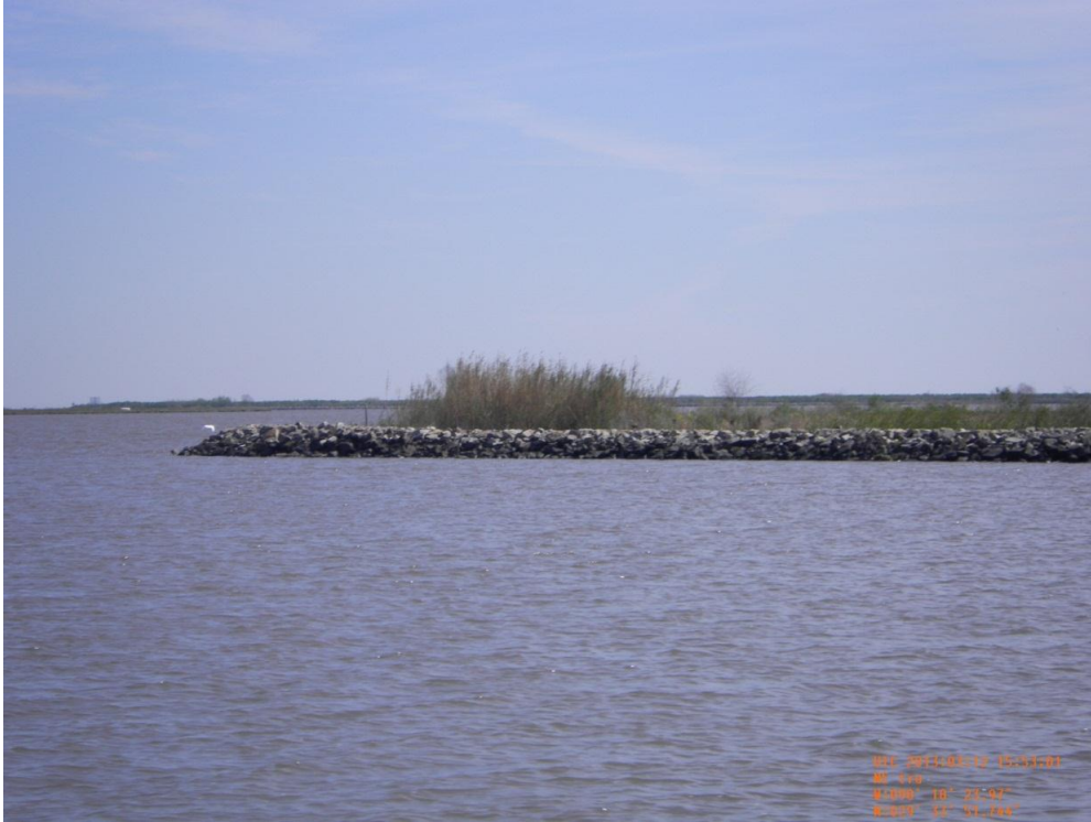
Photo 13: View of the CU#3 rock dike along the southern end of Bayou Perot
