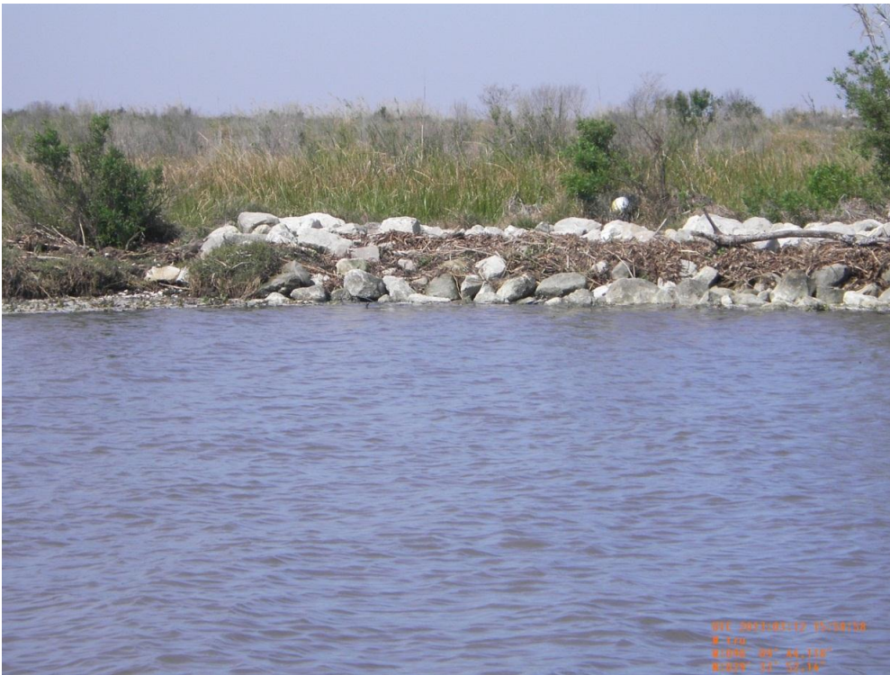
Photo 18: View of CU#4 rock tie-in on south side of oilfield canal
