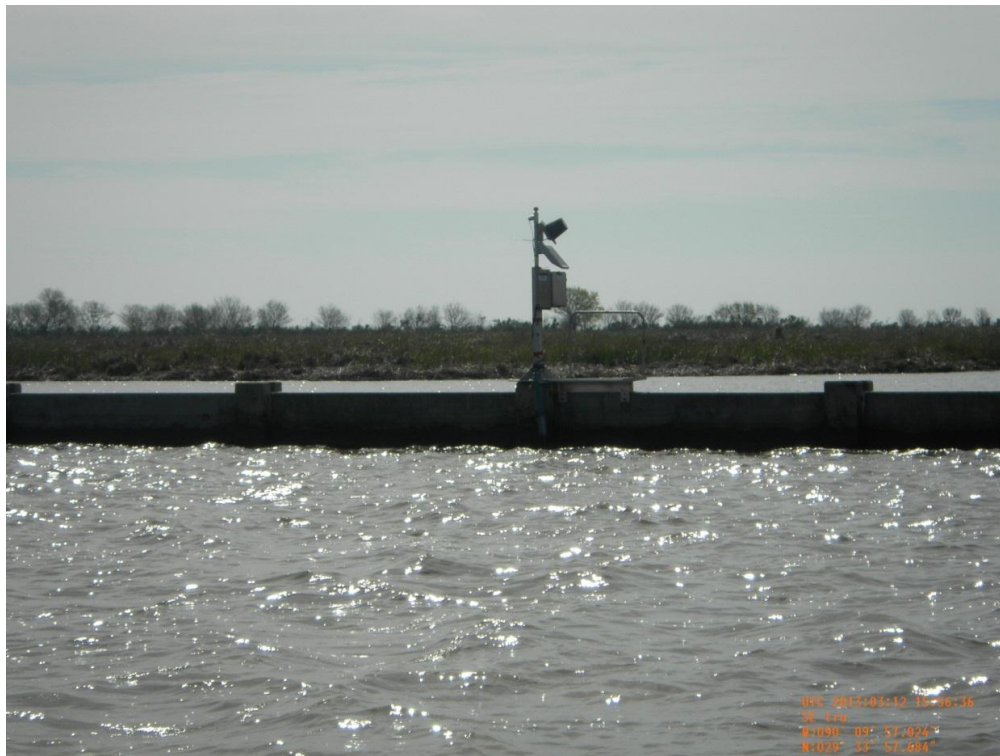
Photo 16: View of data station illicitly installed on the CU#4 concrete wall
