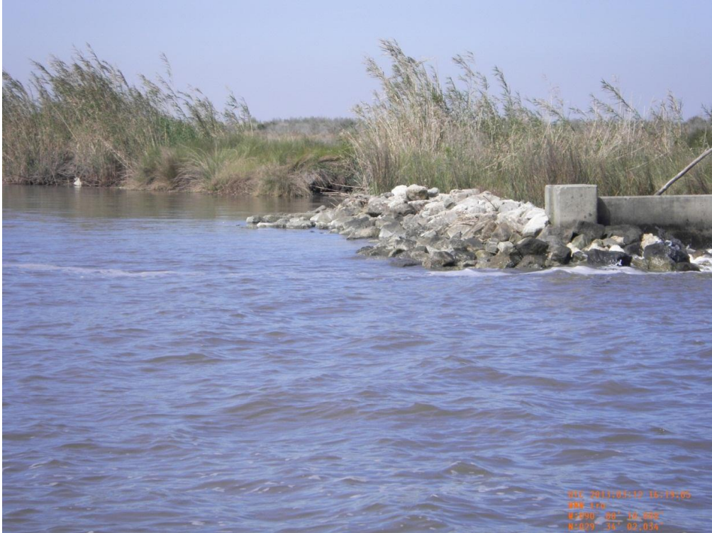
Photo 23: View of the CU#4 rock tie-in on the west side of Harvey Cutoff canal
