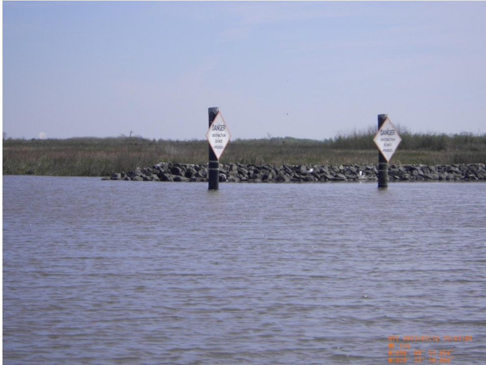
Photo 11: View of a rock dike opening and warning signs along CU#3
