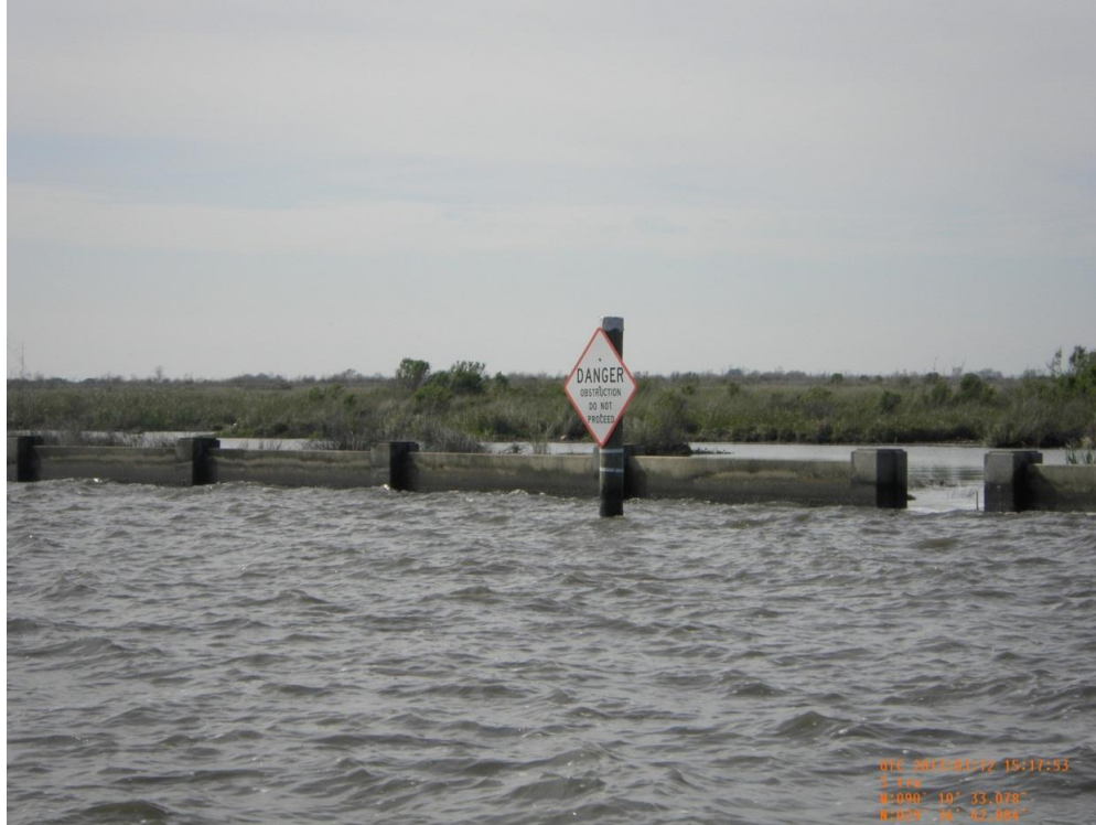
Photo 35: View of concrete wall and warning sign along CU#5
