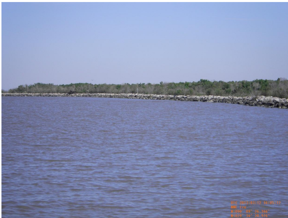
Photo 2: View of CU#2 rock dike along the southern end of Bayou Perot looking east
