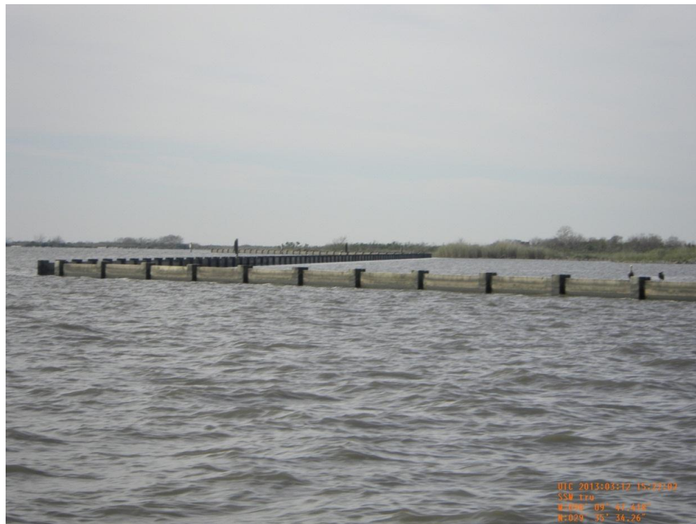
Photo 36: View of concrete wall of CU#5 along Bayou Perot looking south
