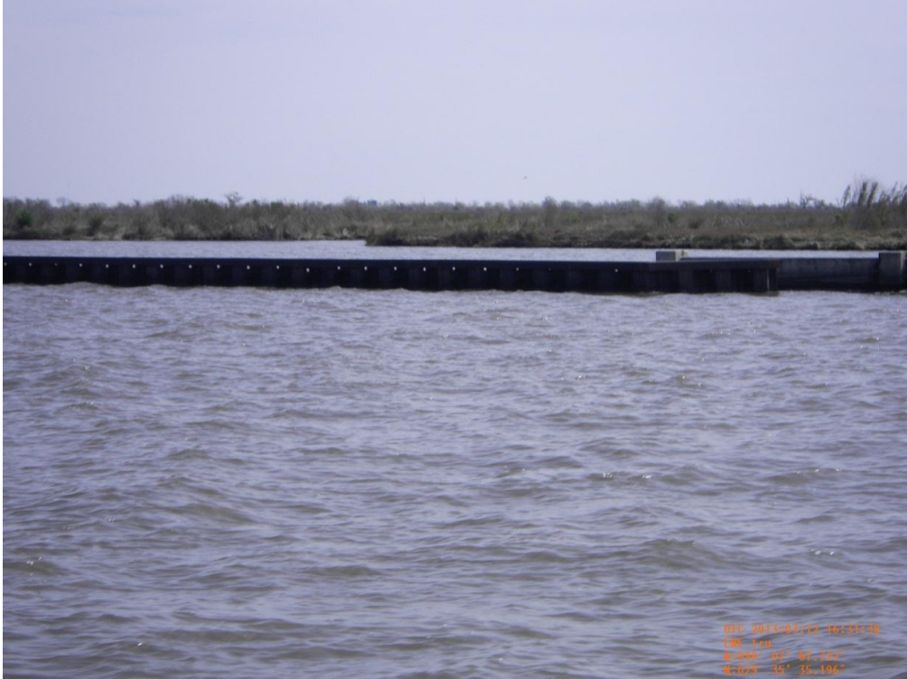
Photo 29: View of steel bulkhead placed to close gap left in CU#4 concrete wall
