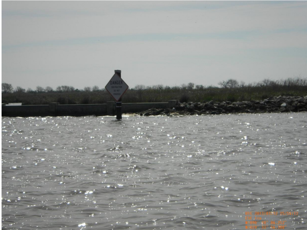
Photo 15: View of rock revetment tie-in on the western end of CU#4
