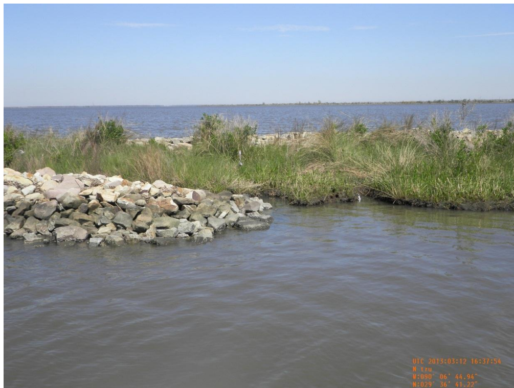
Photo 38: View of CU#6 rock embankment tie-in on north side of oilfield canal
