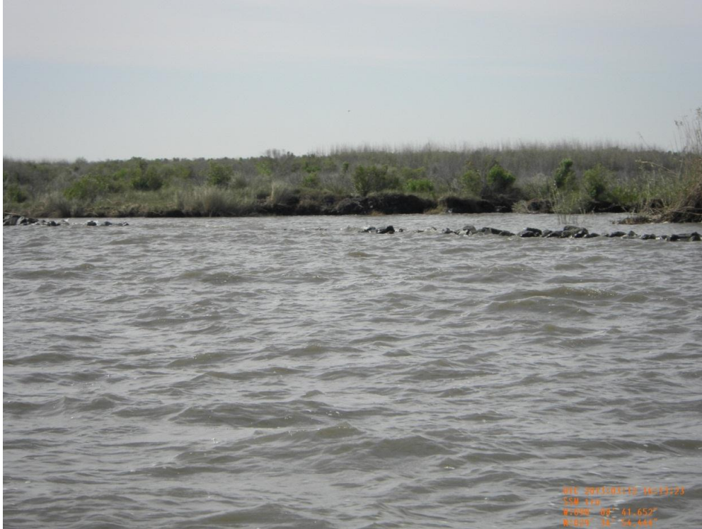
Photo 7: View of a low section along the CU#2 rock dike near the Harvey Cutoff canal
