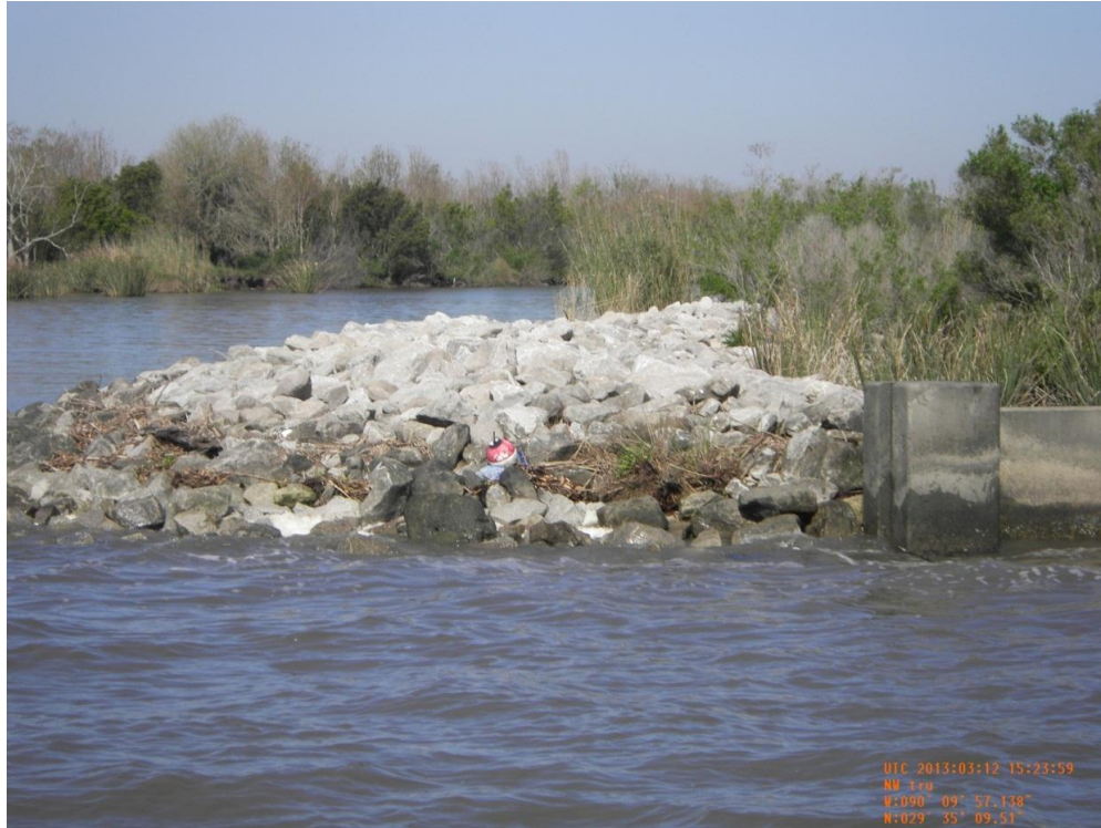
Photo 37: View of rock revetment embankment tie-in on the south end of CU#5
