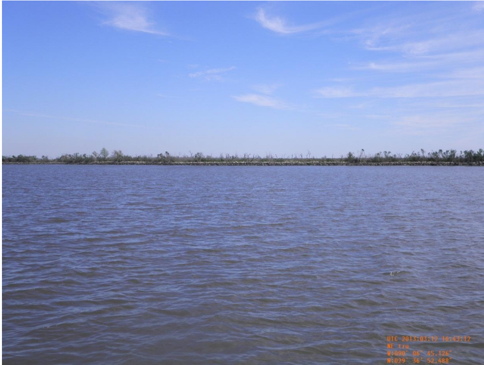
Photo 39: View of CU#6 rock dike along the eastern side of Bayou Rigolettes
