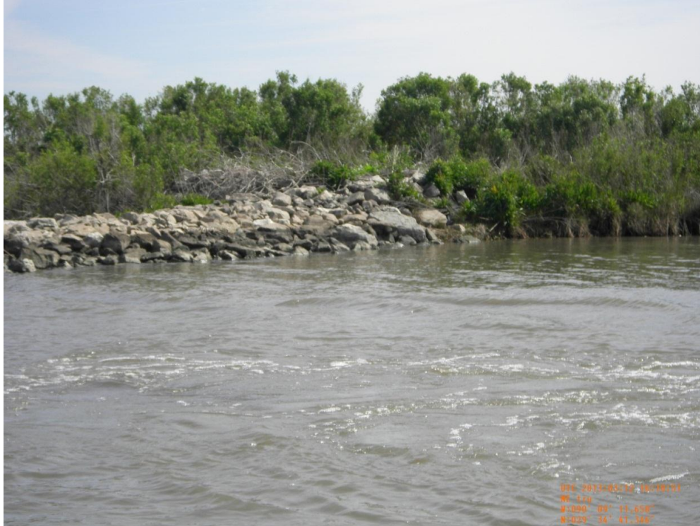
Photo 5: View of CU#2 embankment tie-in on east side of oilfield canal
