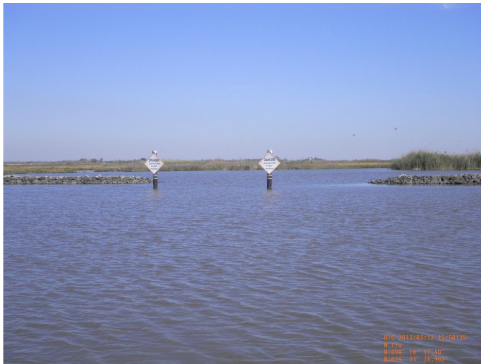
Photo 12: View of a rock dike opening and warning signs along CU#3
