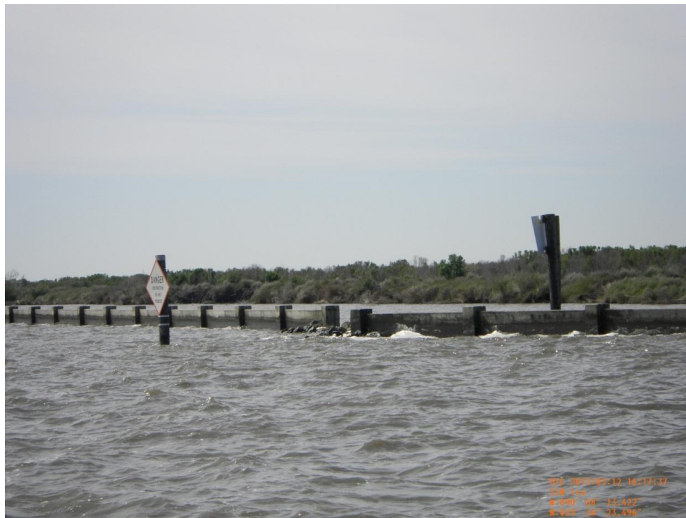
Photo 22: View of the CU#4 concrete wall near the Harvey Cutoff canal
