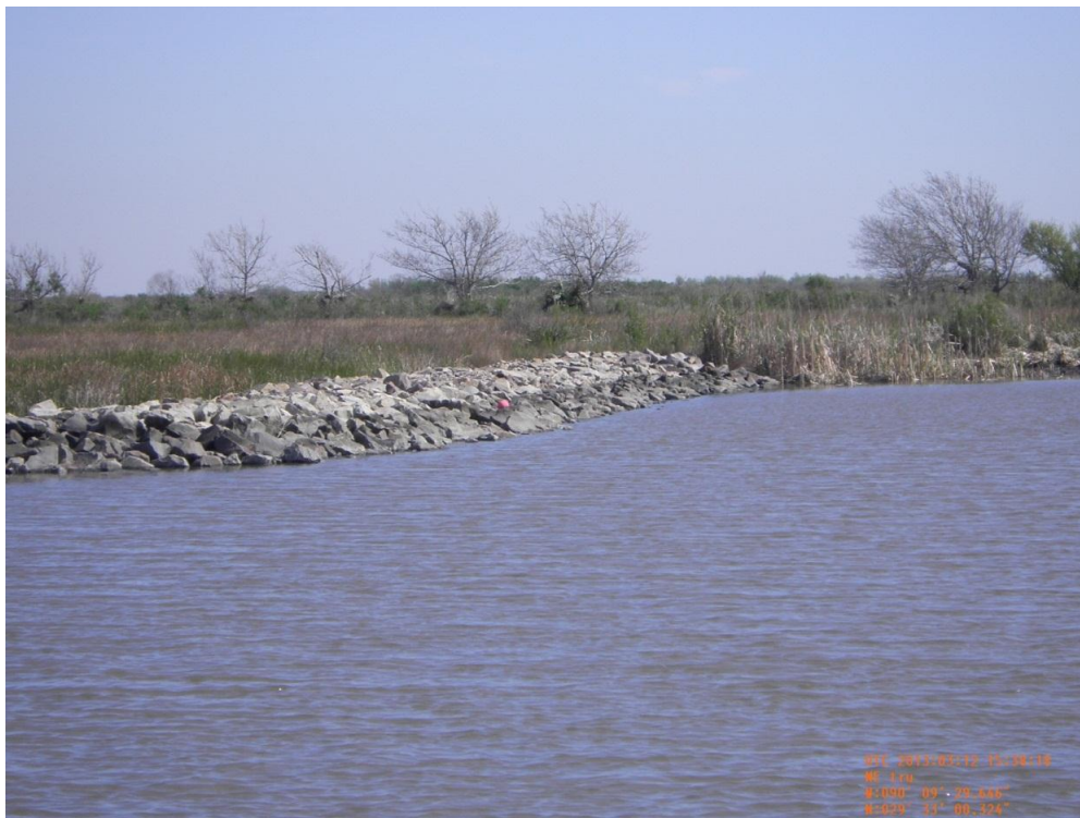
Photo 8: View of the southern embankment tie-in of CU#3 along the eastern edge of Little Lake
