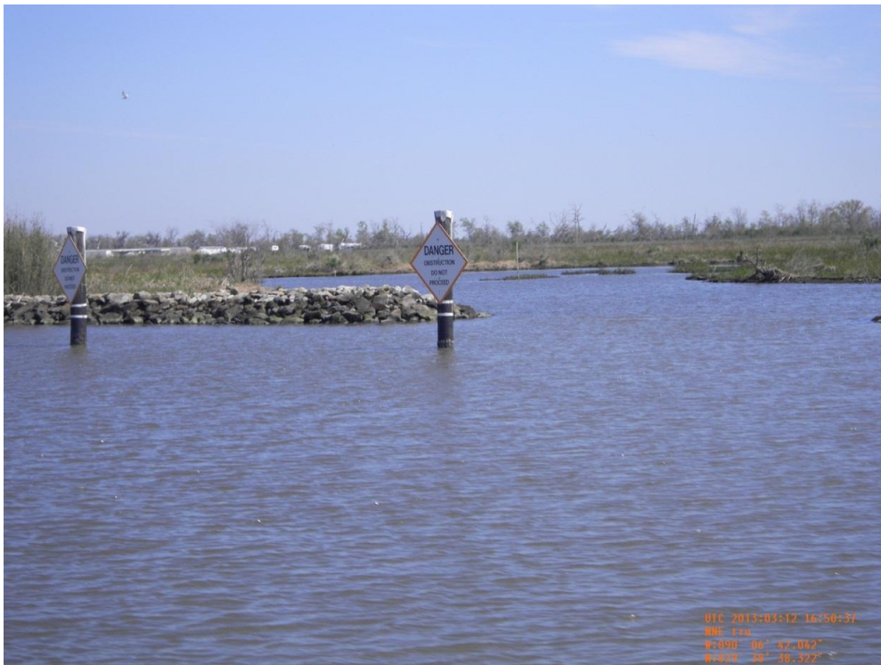
Photo 42: View of warning signs and CU#6 rock dike along eastern side of Bayou Rigolettes
