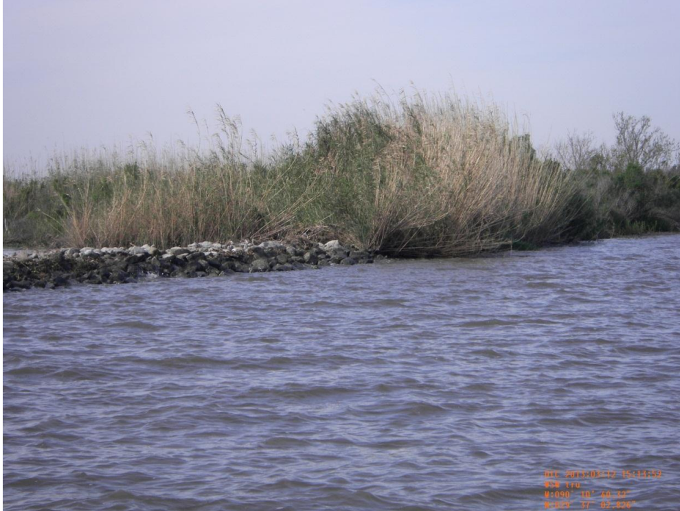
Photo 33: View of rock revetment embankment tie-in on the north end of CU#5
