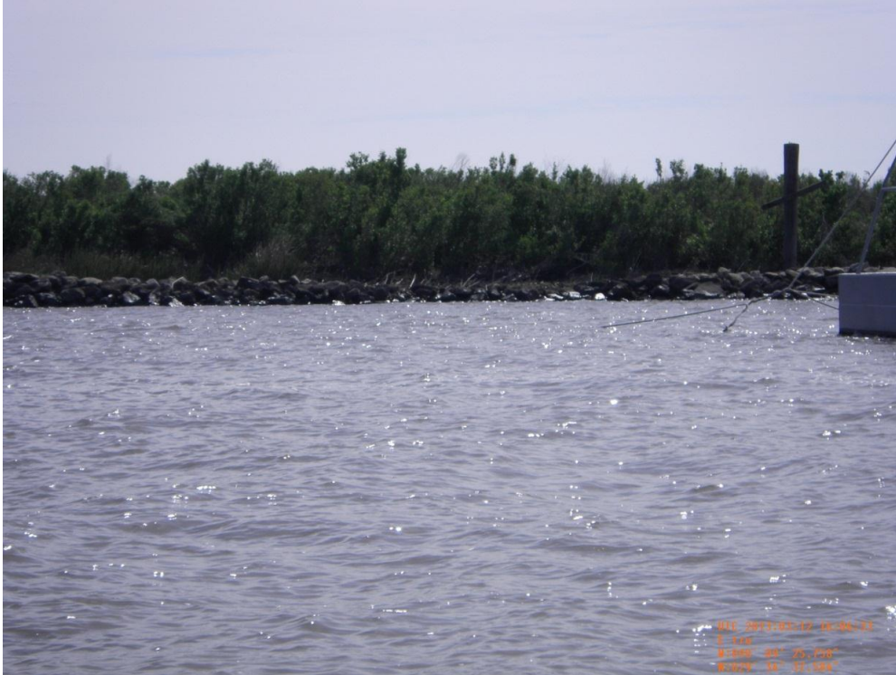
Photo 3: View of a low section of the CU#2 rock dike along the southern end of Bayou Perot
