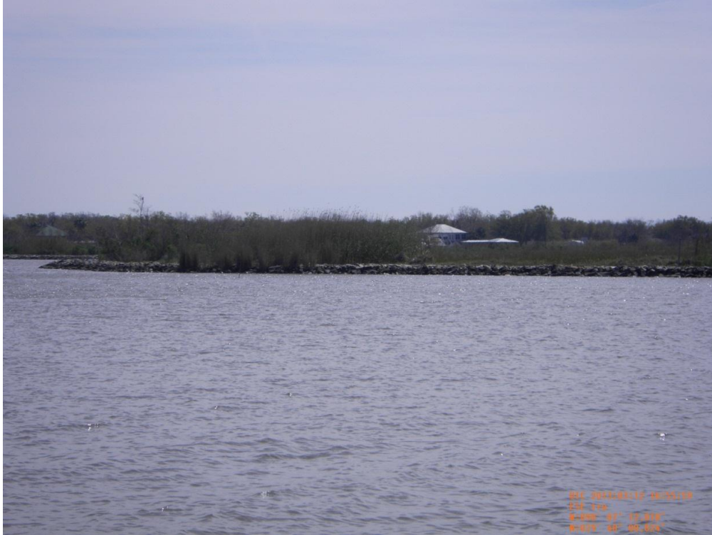
Photo 47: View of CU#6 rock dike from Bayou Rigolettes looking east
