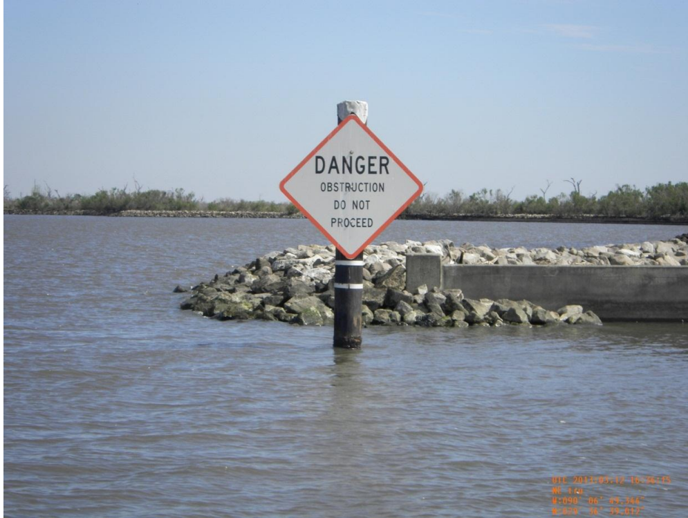
Photo 31: View of warning sign and CU#4 concrete wall transition to rock revetment tie-in
