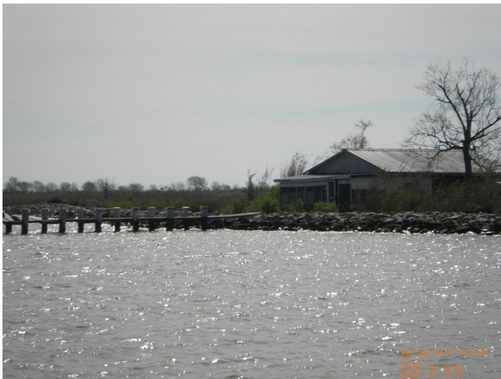
Photo 14: View of the CU#3 rock dike along the southern end of Bayou Perot
