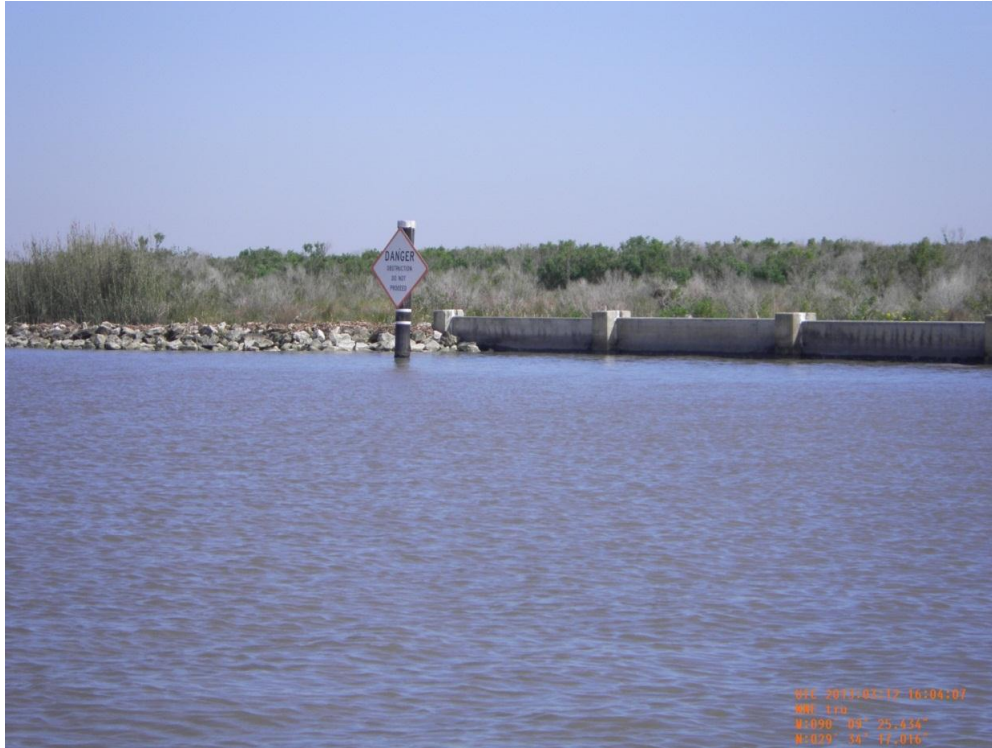
Photo 1: View of transition from CU#4 concrete wall to CU#2 rock dike
