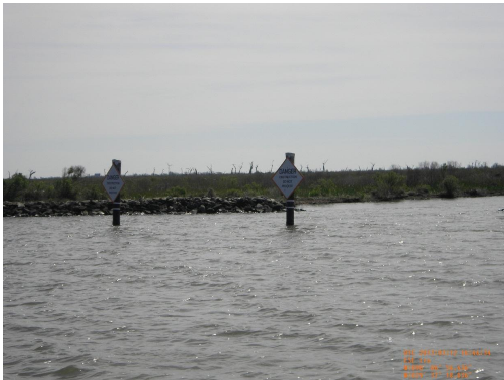
Photo 40: View of warning signs and CU#6 rock dike along eastern side of Bayou Rigolettes
