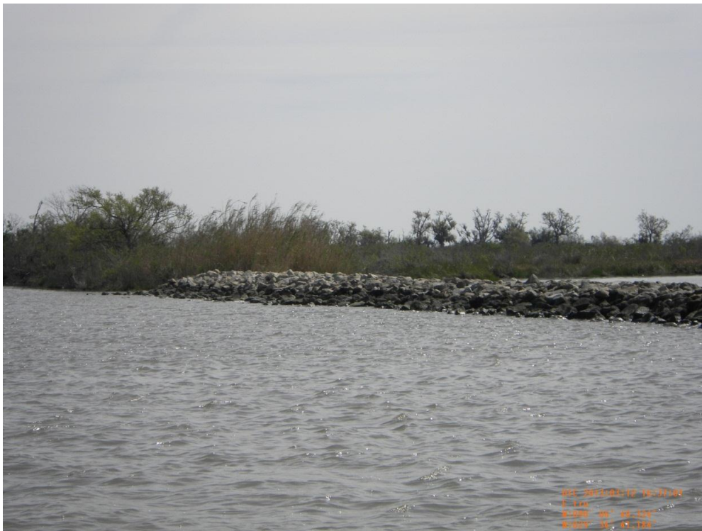
Photo 32: View of CU#4 rock embankment tie-in on south side of oilfield canal
