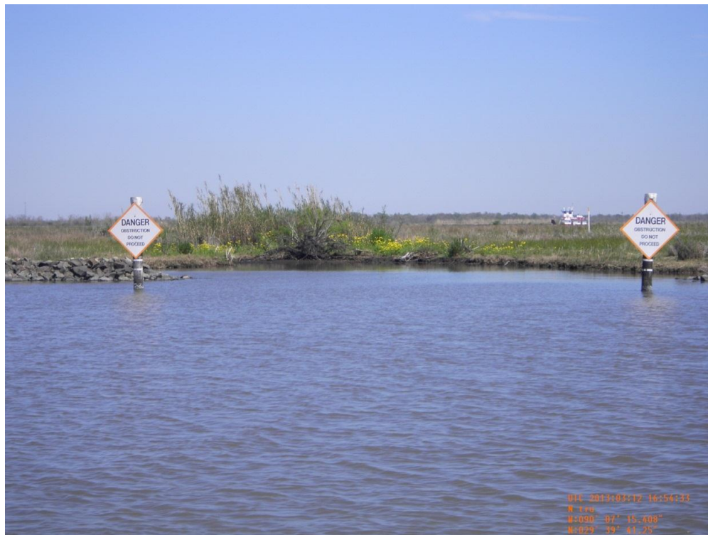
Photo 46: View of warning signs and CU#6 rock dike along eastern side of Bayou Rigolettes
