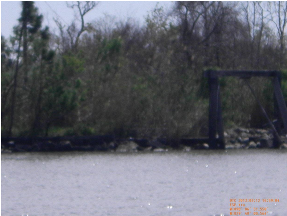
Photo 48: View of northern CU#6 rock dike embankment tie-in near Laffite
