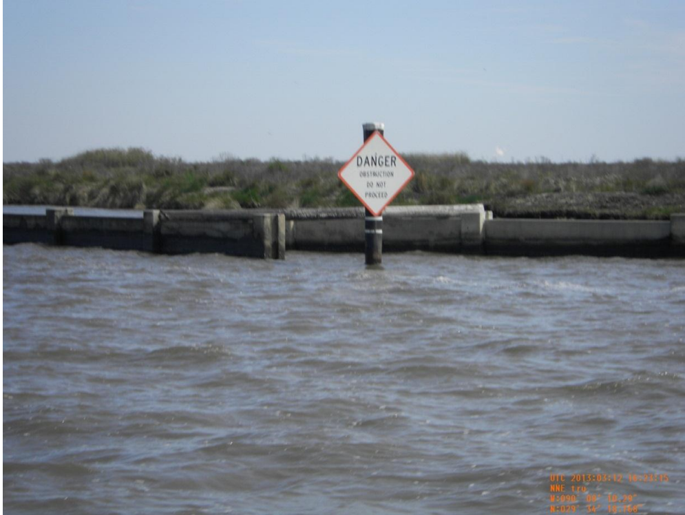
Photo 27: View of timber piling resting on top of the CU#4 concrete wall near Harvey Cutoff canal
