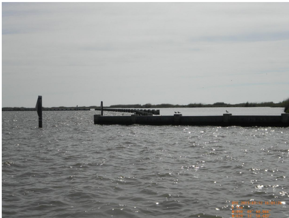
Photo 20: View of CU#4 concrete wall along southern end of Bayou Perot looking east
