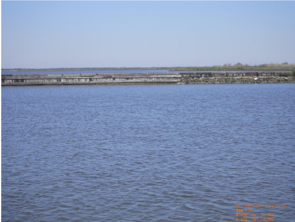
Photo 43: View of intersection of CU#6 rock dike and pipeline timber bulkhead looking north
