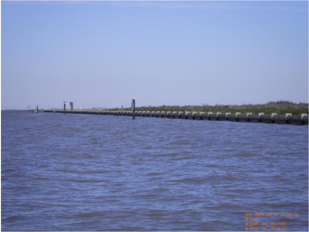
Photo 26: View of the CU#4 concrete wall along the east side of Harvey Cutoff canal
