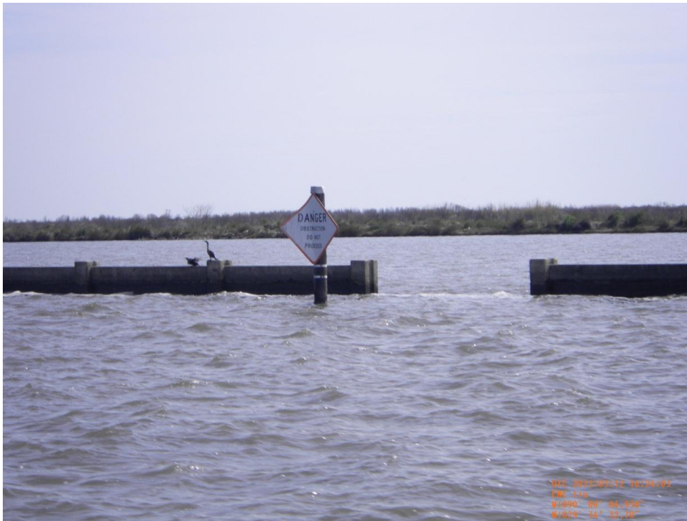
Photo 28: View of a bent warning sign along CU#4 concrete wall near Harvey Cutoff canal
