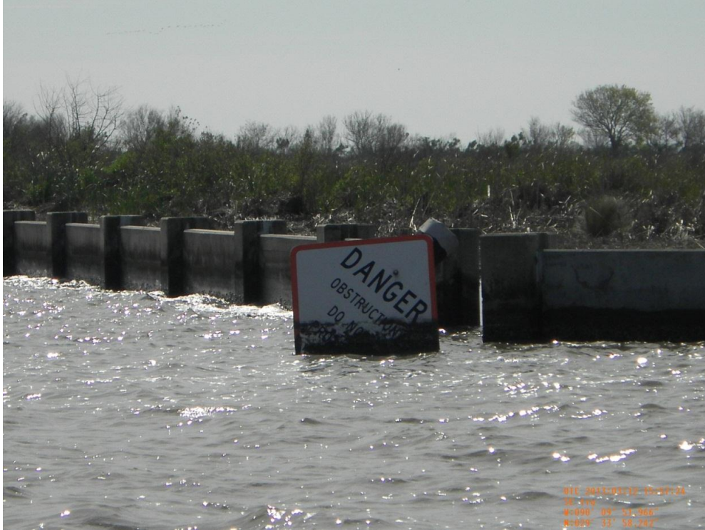
Photo 17: View of damaged warning sign along CU#4 concrete wall near an oilfield canal
