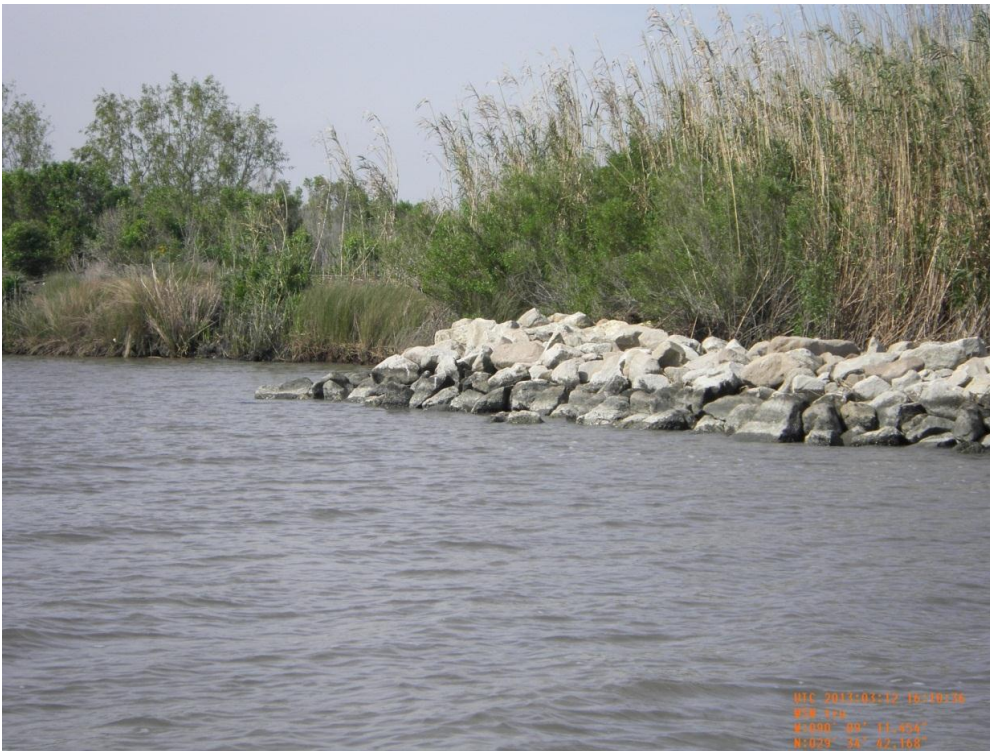
Photo 4: View of CU#2 embankment tie-in on west side of oilfield canal
