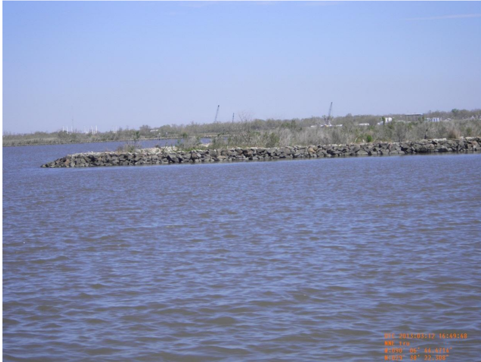
Photo 41: View of CU#6 rock dike from Bayou Rigolettes looking northeast
