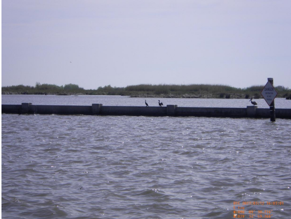
Photo 21: View of CU#4 concrete wall along southern end of Bayou Perot looking south
