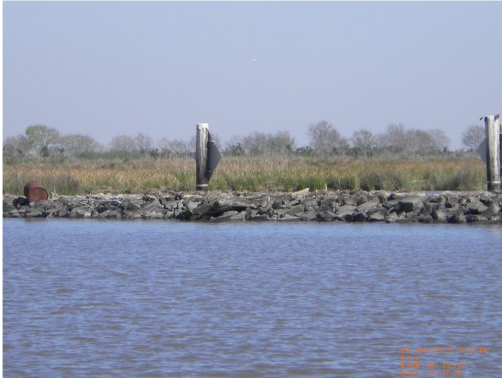
Photo 9: View of CU#3 rock dike and warning signs on the eastern edge of Little Lake
