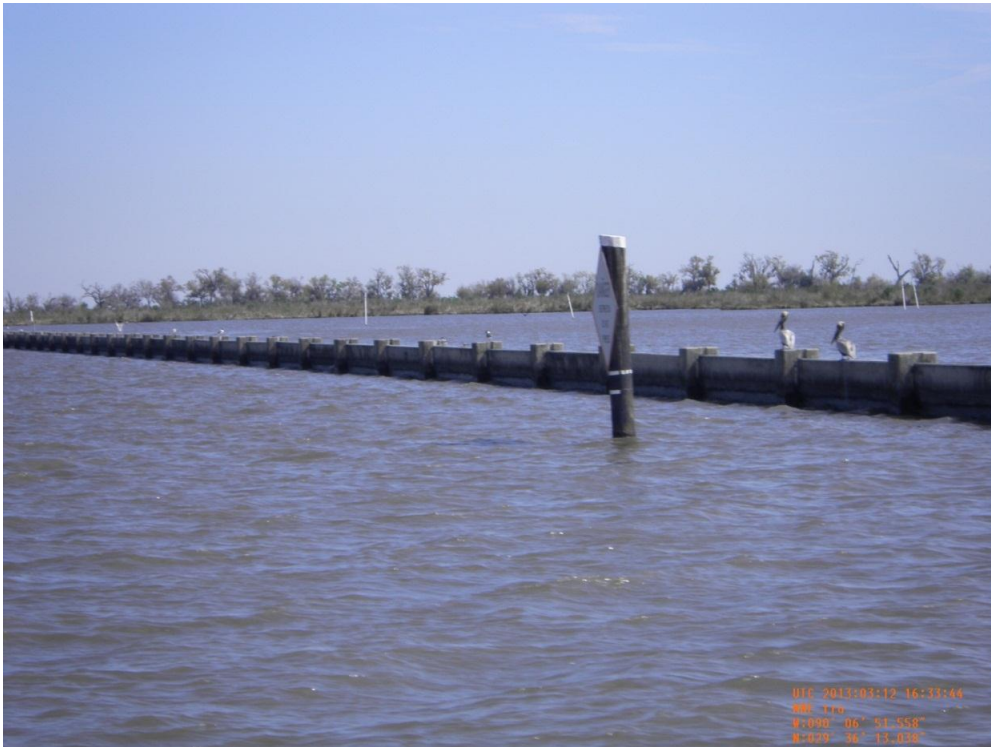
Photo 30: View of CU#4 concrete wall along the eastern side of Bayou Rigolettes
