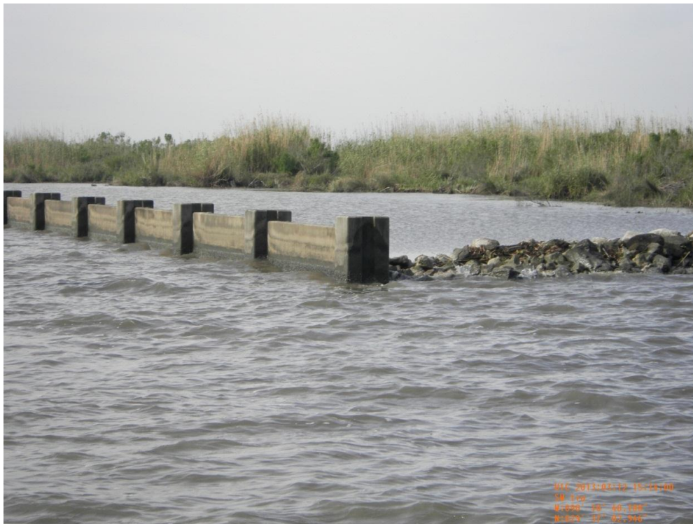
Photo 34: View of transition between rock revetment and concrete wall on north end of CU#5
