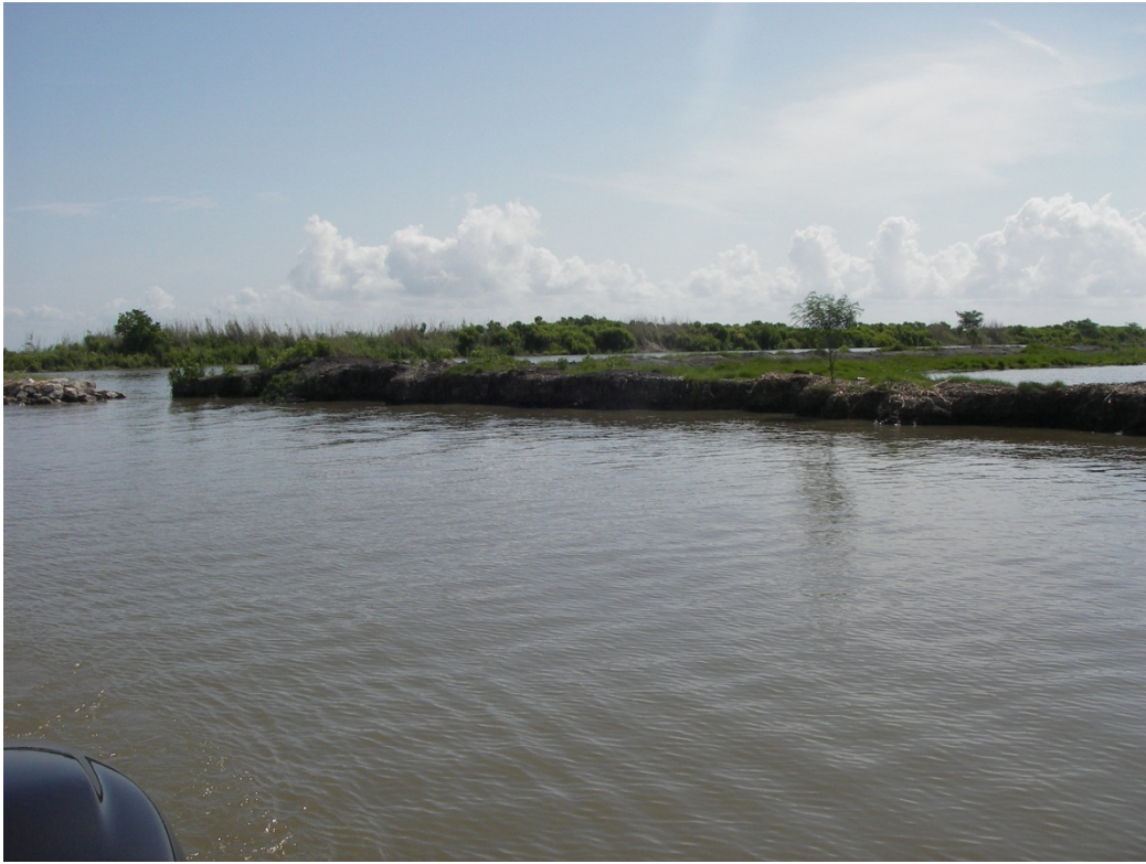
Photo No. 3, Containment Dike along North-South Canal near Rock Plug
