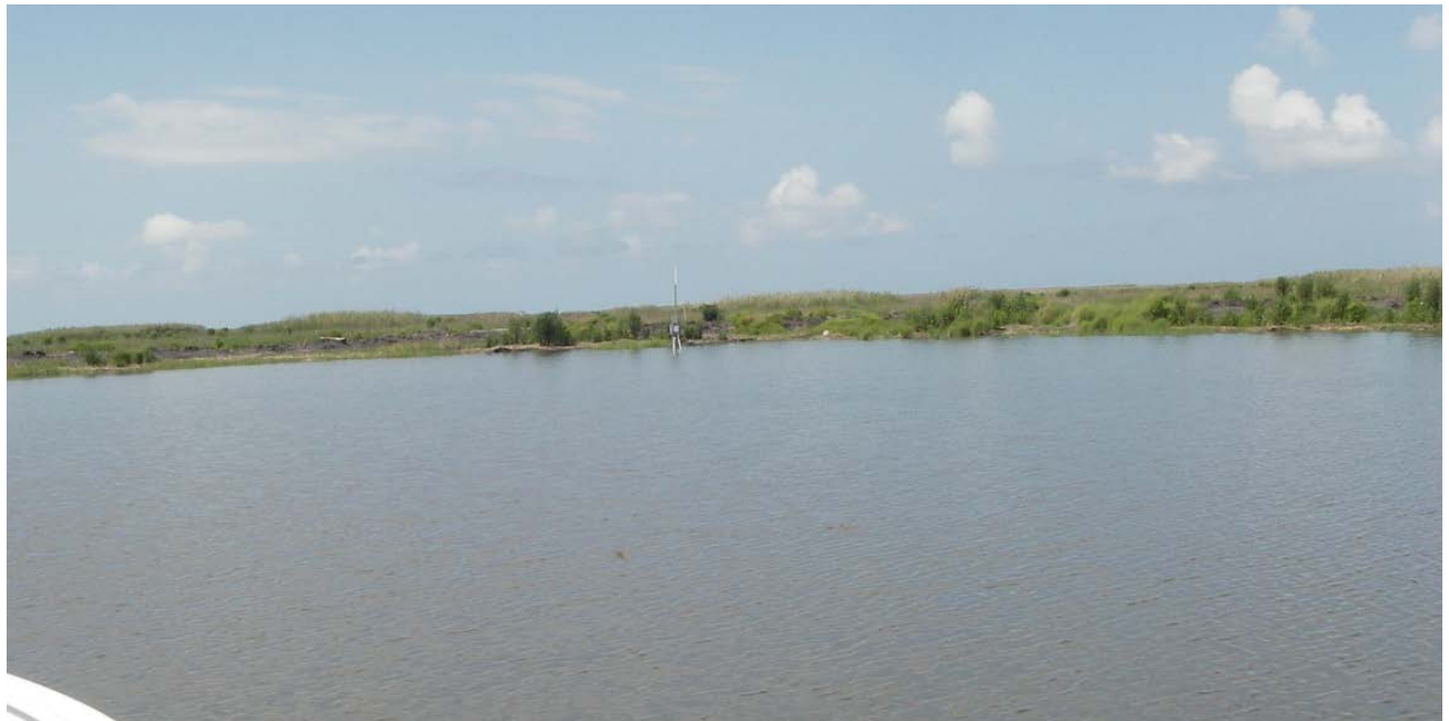
Photo No. 6 , Earthen Plug at End of North-South Pipeline Canal
