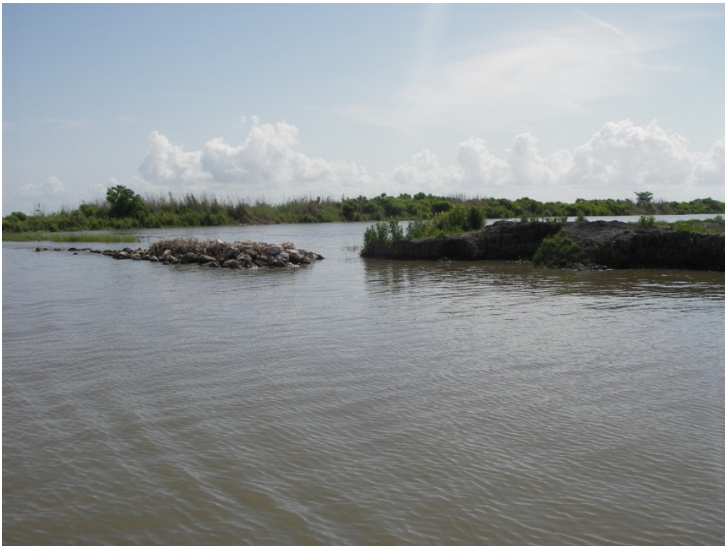
Photo No.2, Containment Dike along North-South Canal at Rock Plug
