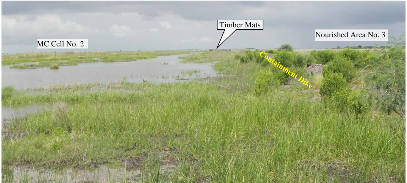
Photo No. 5 , Marsh Creation Cell No. 2, Borrow Channel, Containment Dike, Timber Mats, and Nourished Area No. 3 (Looking West)
