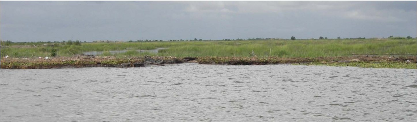
Photo No. 9 , Containment Dike along Gulfward Shoreline at NE Corner of MC Cell No. 1 (Original Breach near Southern Section of Intended Armor Area)
