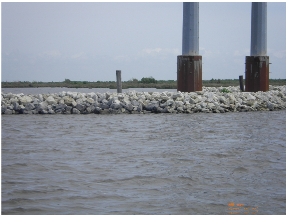
Photo 34: View of the Lake Rim rock dike refurbishment from Breton Canal, looking northwest
