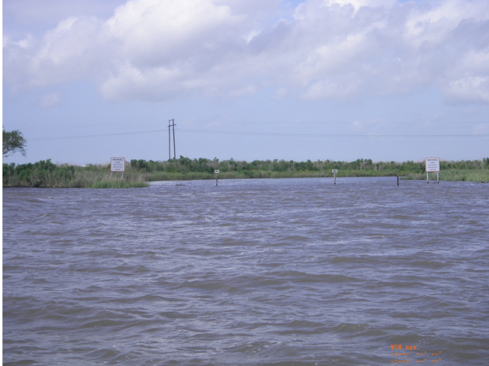
Photo 53: Overall View of Structure 7 fixed crest rock weir with boat bay, looking west
