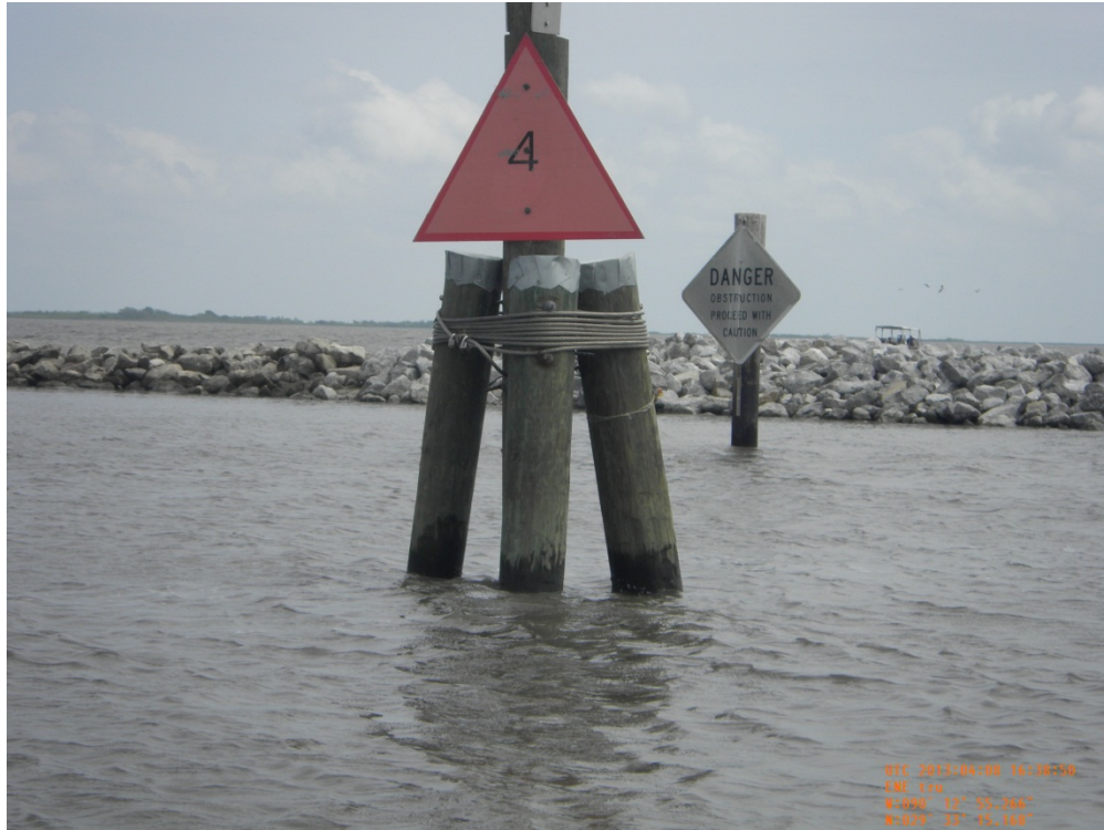
Photo 63: View of newly installed timber pile cluster and sign on northwest side of Structure 14
