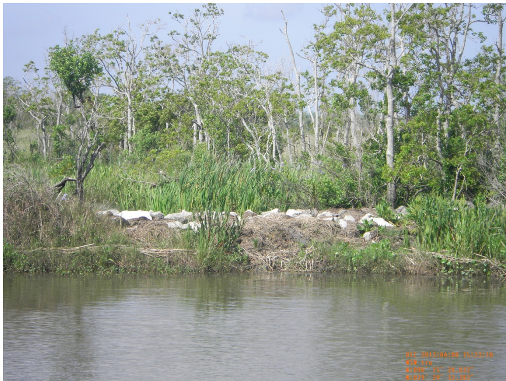
Photo 18: Close up view of the embankment tie-in on the southeast side of Structure 90
