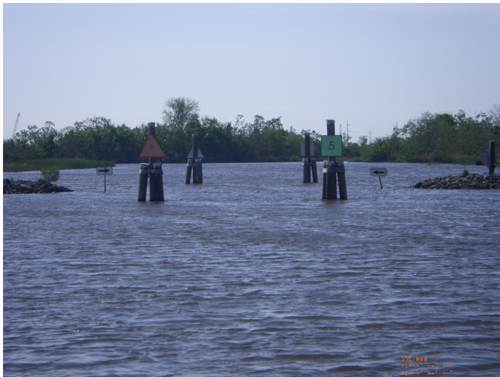
Photo 4: Overall view of Structure 1 rock riprap weir, looking southwest
