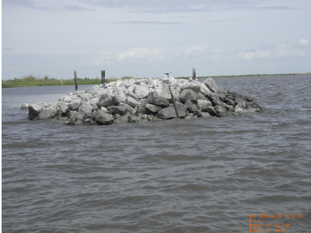
Photo 61: View along the rock recap on the northern side of Structure 14 from the barge bay, looking north
