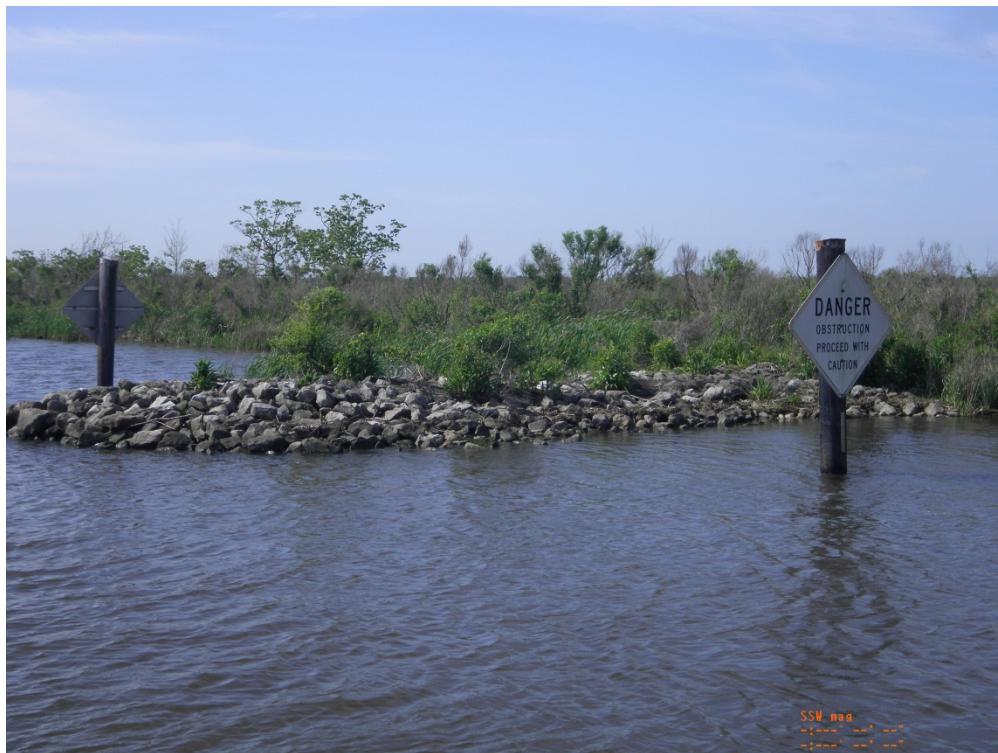
Photo 6: Close up view of the embankment tie-ins on the west side of Structure 1
