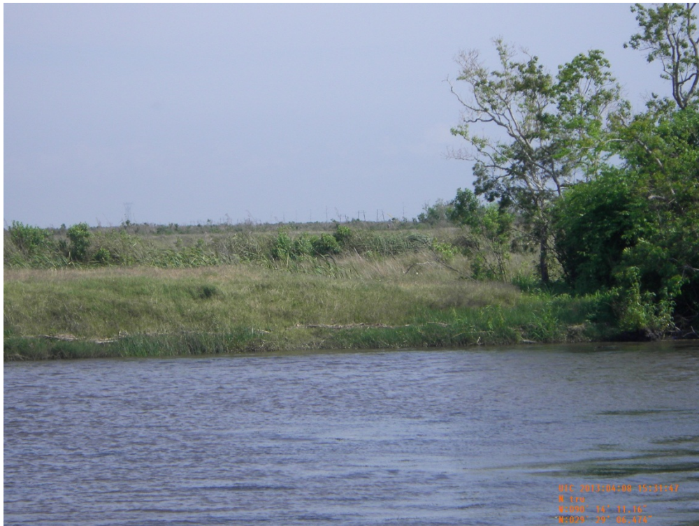
Photo 22: View of Breach Closure No. 2 which was part of the 2012 Maintenance Project
