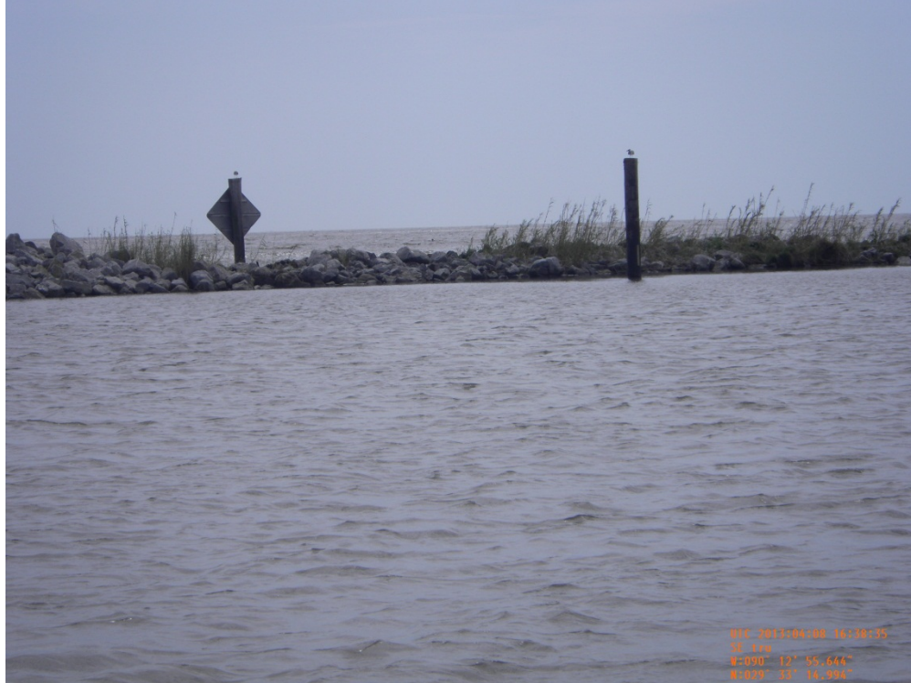
Photo 65: View along the southern side of Structure 14 from Clovelly Canal, looking southeast
