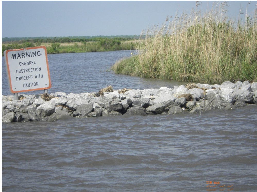
Photo 43: View of warning sign and rock recap on the northern side of Structure 2
