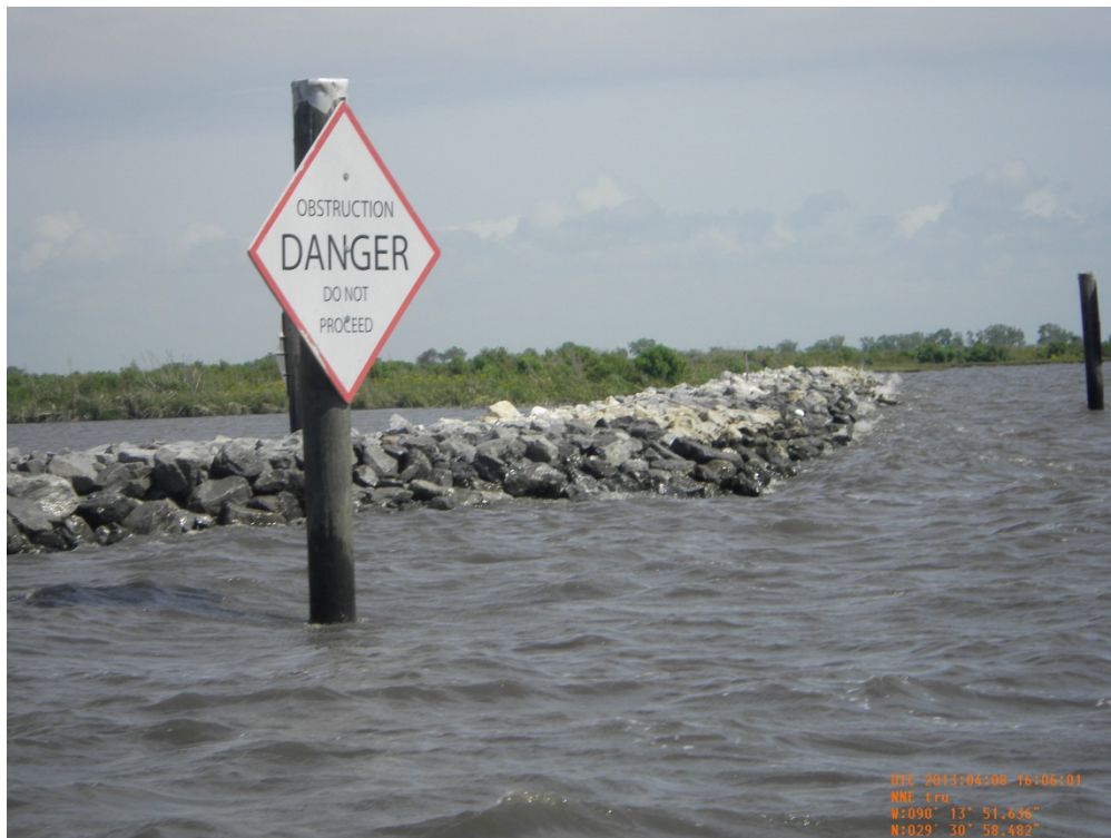
Photo 50: View of new warning sign and transition from Rock Dike Extension to Structure 4A&4B
