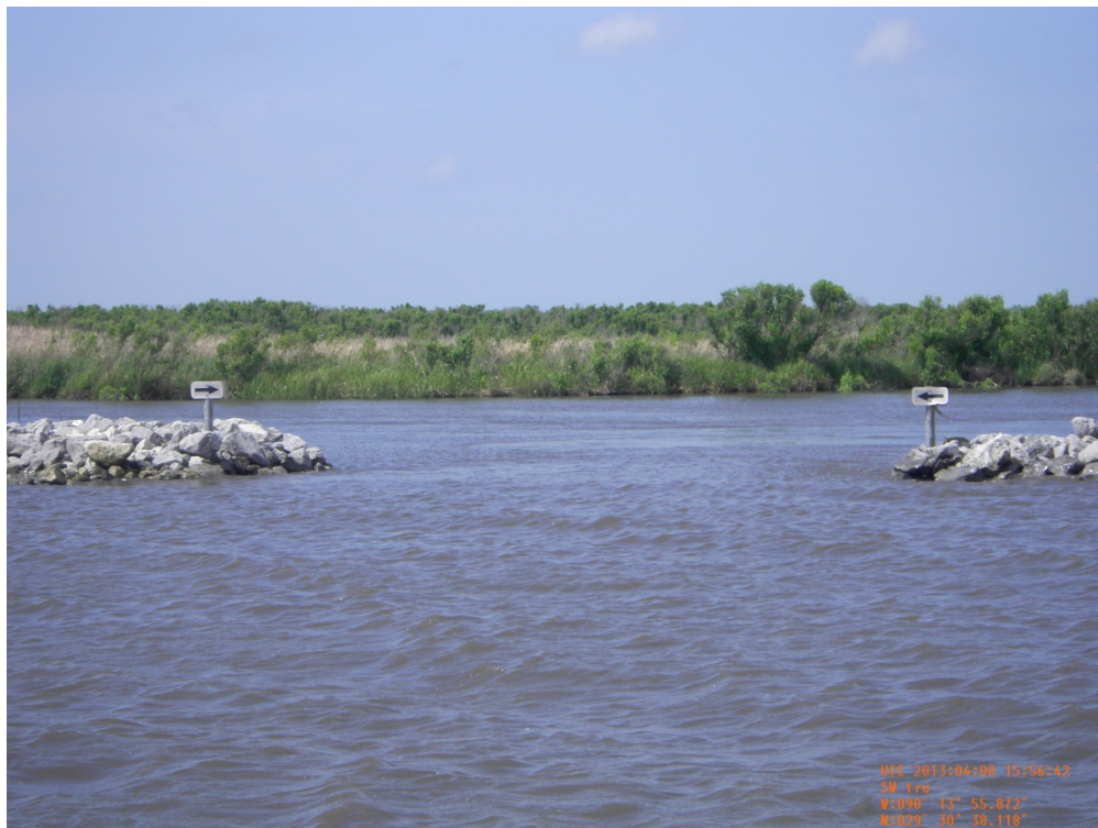
Photo 40: Overall view of Structure 2 fixed crest rock weir with boat bay, looking southwest
