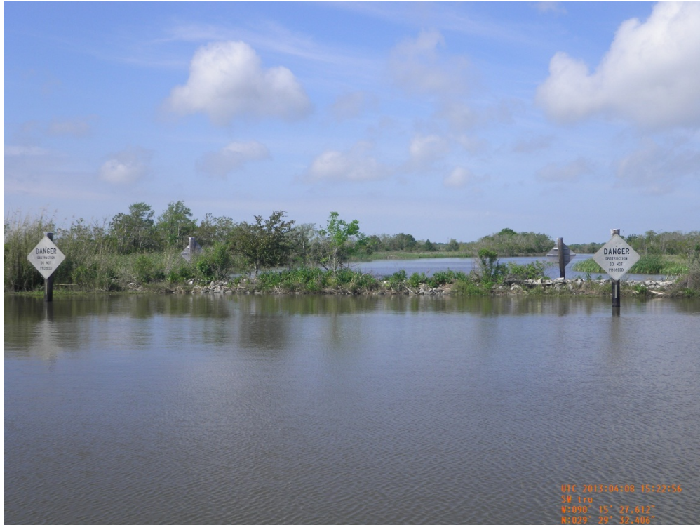
Photo 17: Overall view of Structure 90 rock plug, looking southwest
