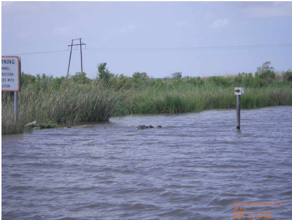
Photo 54: View of the warning sign and embankment tie-in on the southern end of Structure 7
