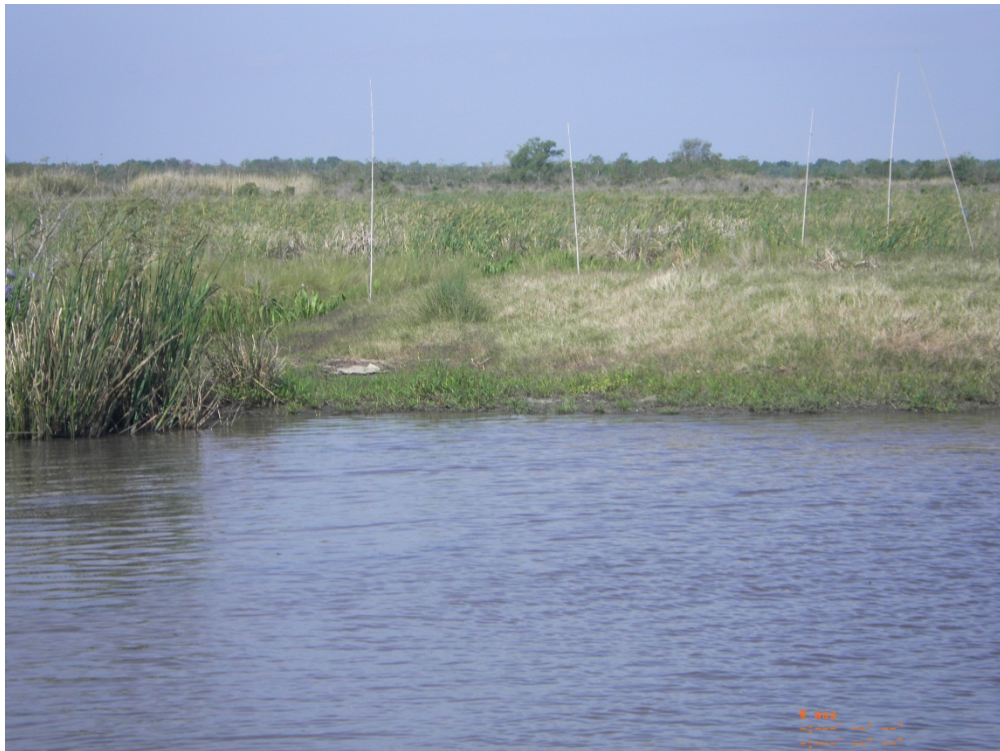
Photo 10: View of Breach Closure No. 5 which was part of the 2012 Maintenance Project
