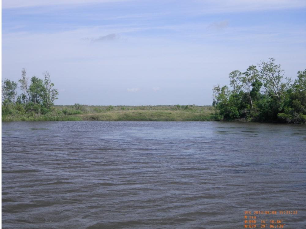
Photo 21: View of Breach Closure No. 2 which was part of the 2012 Maintenance Project
