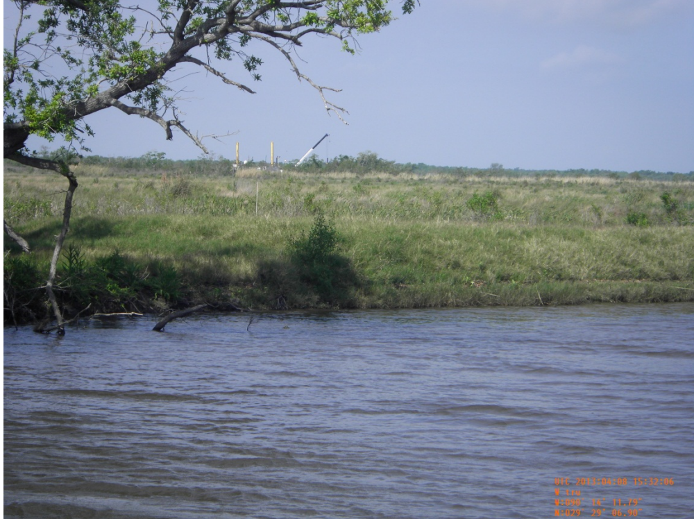
Photo 25: View of Breach Closure No. 3 which was part of the 2012 Maintenance Project
