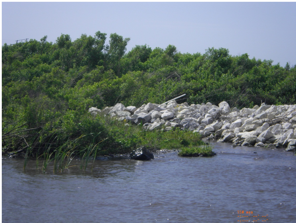
Photo 42: View of the embankment tie-in on the southern side of Structure 2
