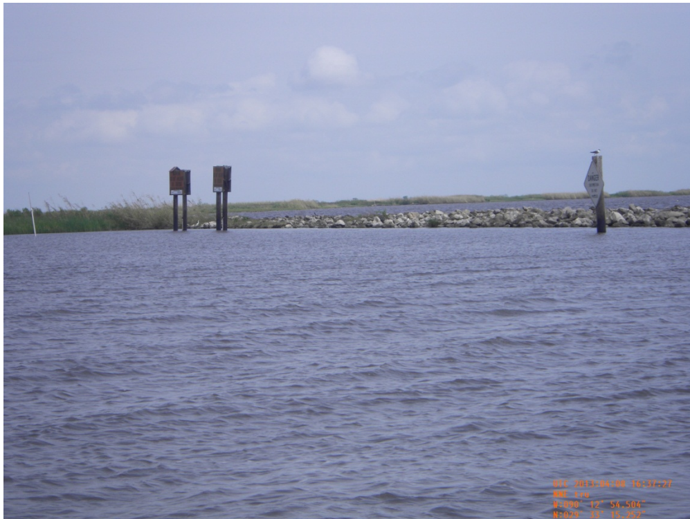
Photo 62: View along the northern side of Structure 14 from Clovelly Canal, looking northeast
