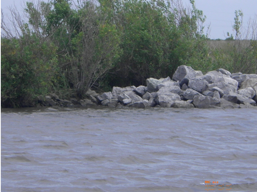
Photo 31: View of the southernmost end of the Lake Rim rock dike refurbishment in Breton Canal
