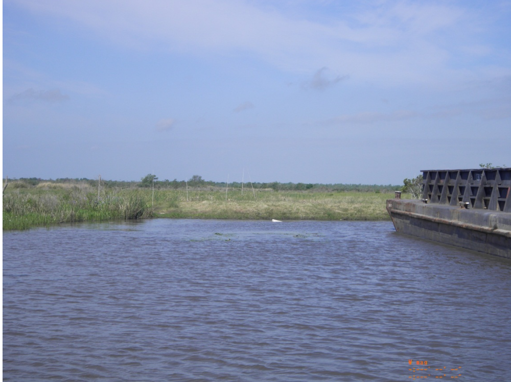
Photo 9: View of Breach Closure No. 5 which was part of the 2012 Maintenance Project
