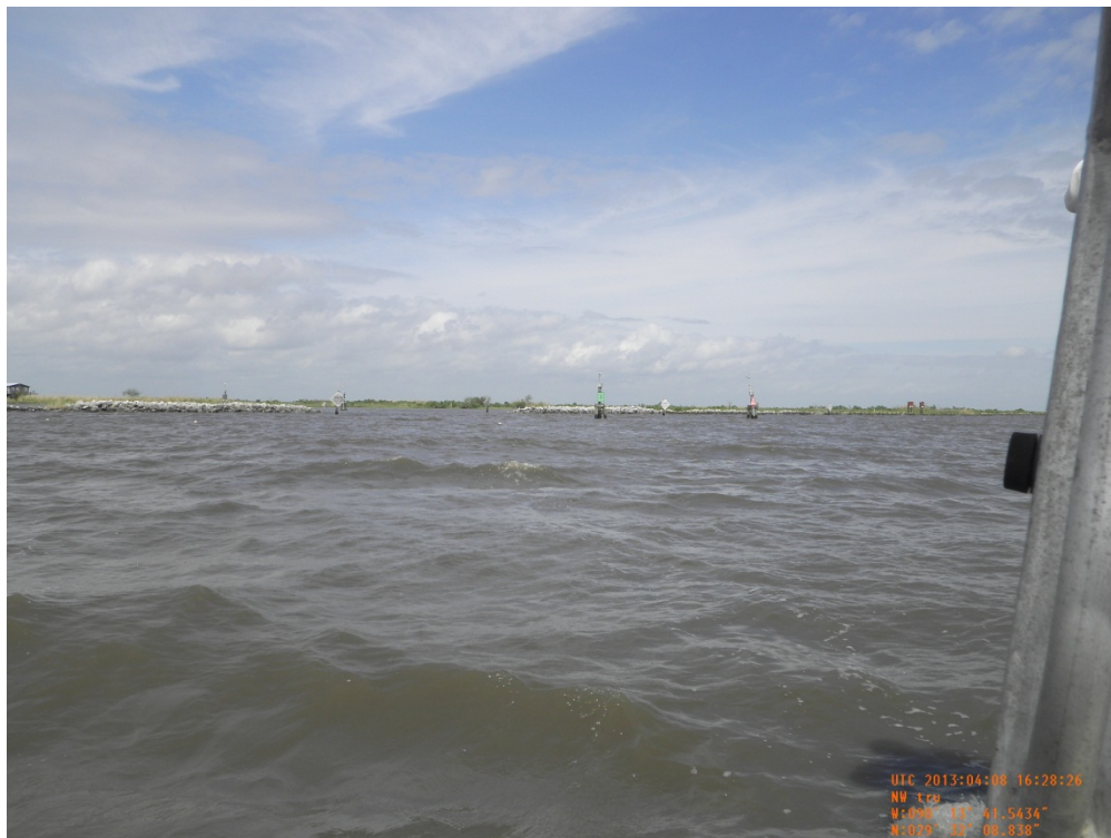
Photo 58: Overall view of Structure 14 fixed crest rock weir with barge bay from Little Lake looking west
