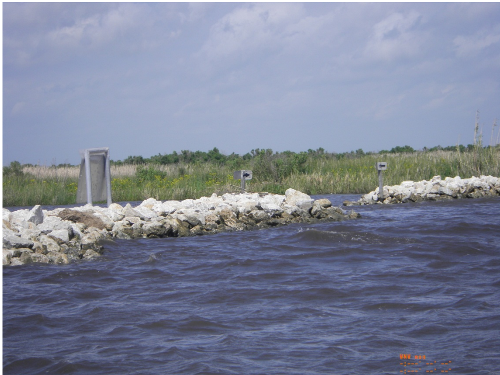
Photo 46: View along the rock recap of Structure 4, looking northwest
