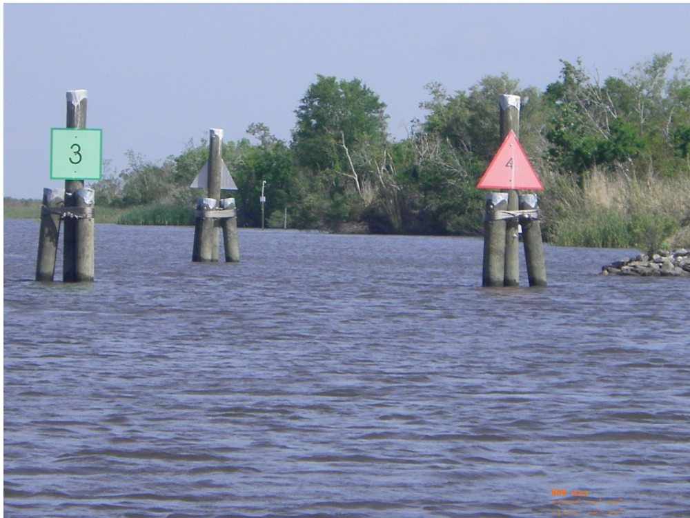
Photo 8: View of the newly installed timber pile clusters and signs on the south side of Structure 1
