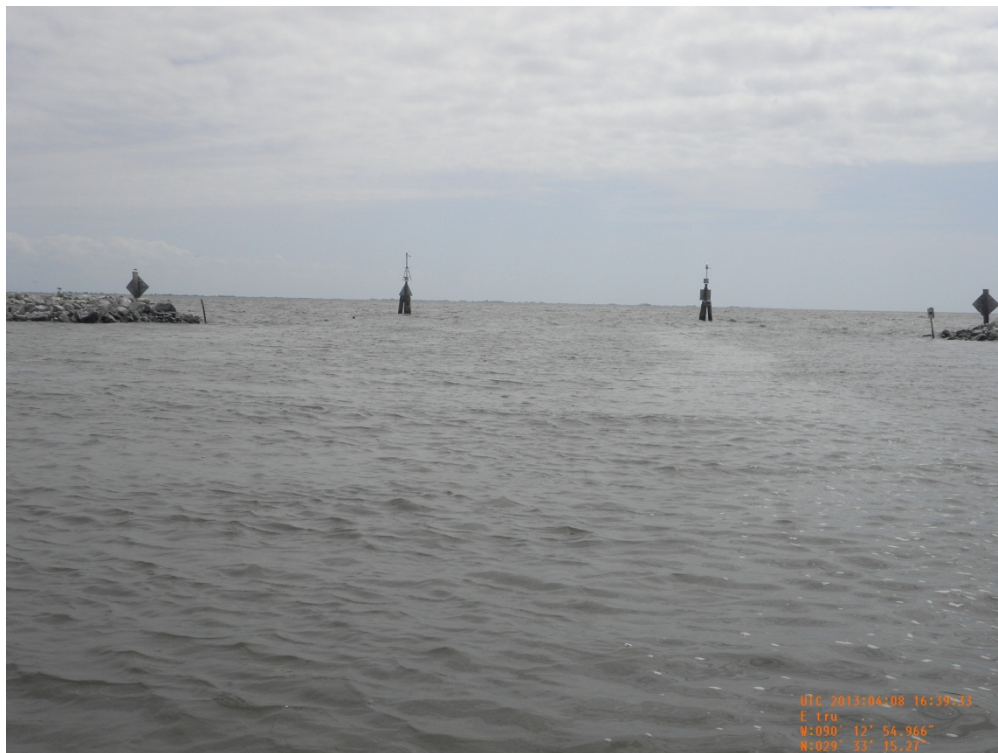
Photo 66: Overall view of Structure 14 fixed crest rock weir with barge bay from Clovelly Canal looking east
