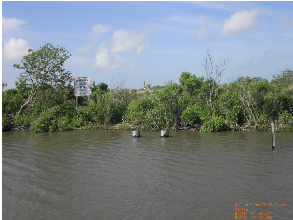
Photo 13: Overall view of Structure 91 rock plug with culvert and flap gate, looking south
