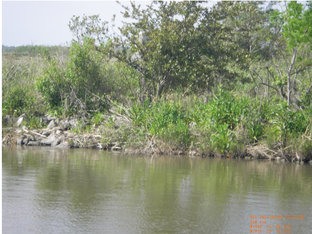
Photo 19: Close up view of the embankment tie-in on the northwest side of Structure 90
