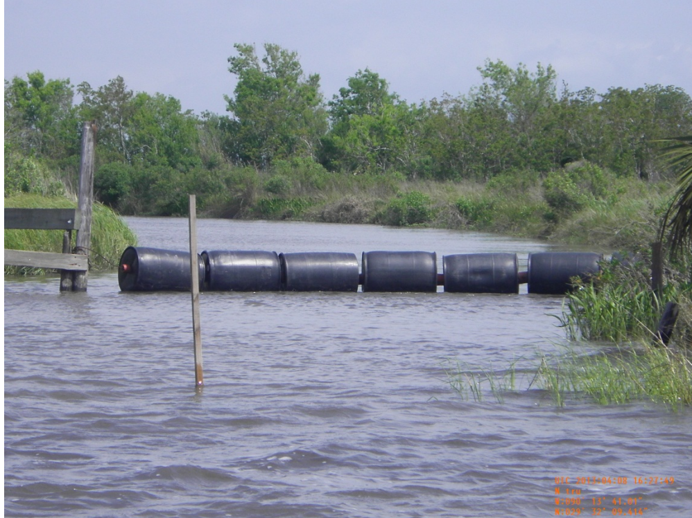
Photo 57: View of Structure 8 rock riprap channel plug, looking north
