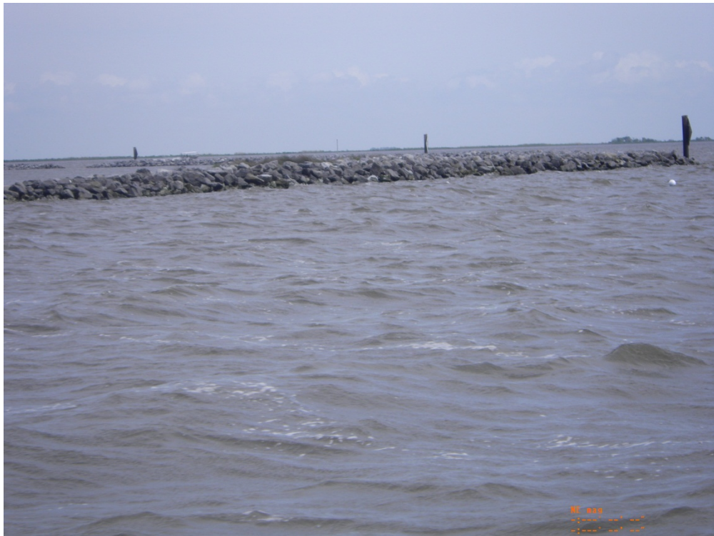
Photo 36: View of the Lake Rim rock dike refurbishment from Breton Canal, looking north
