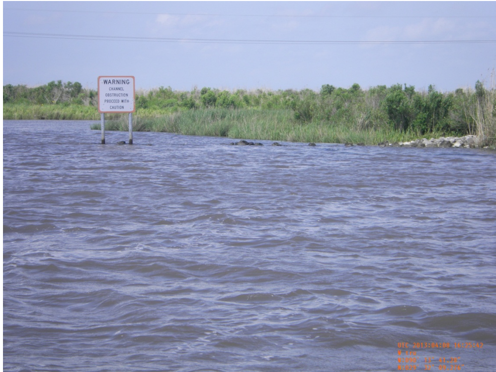
Photo 55: View of the warning sign and embankment tie-in on the northern end of Structure 7
