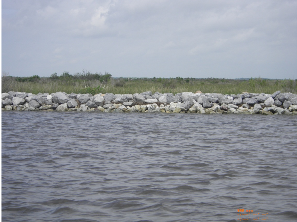
Photo 33: View of the Lake Rim rock dike refurbishment from Breton Canal, looking northwest
