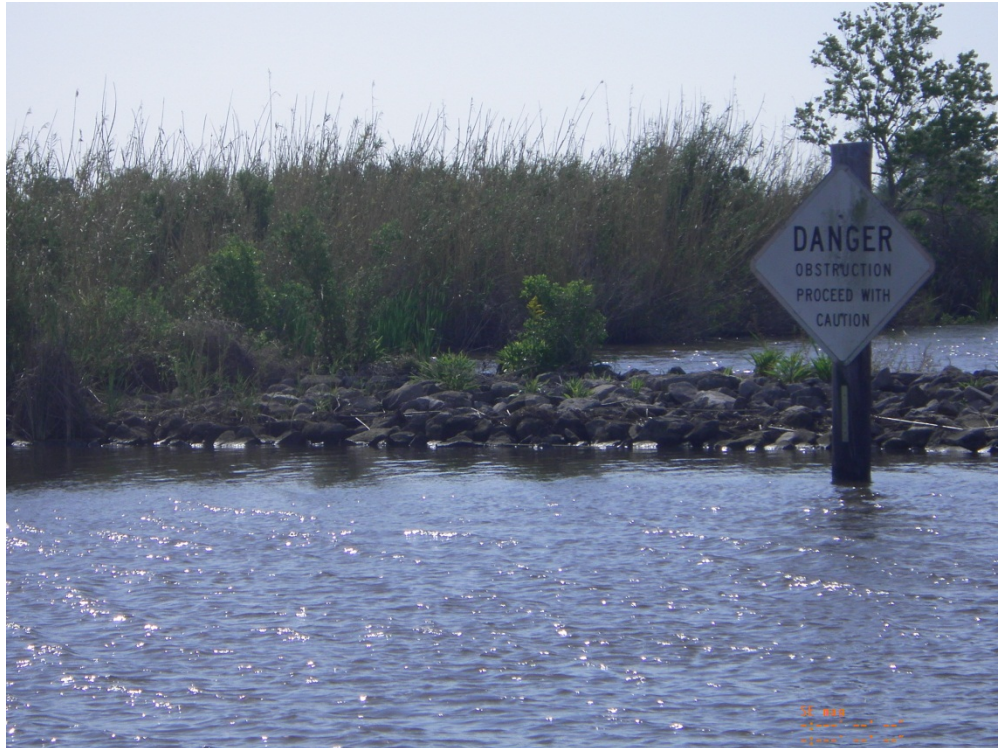
Photo 5: Close up view of the embankment tie-ins on the east side of Structure 1
