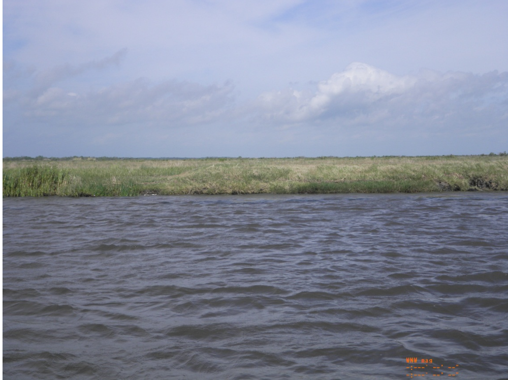
Photo 27: View of Breach Closure No. 1 which was part of the 2012 Maintenance Project
