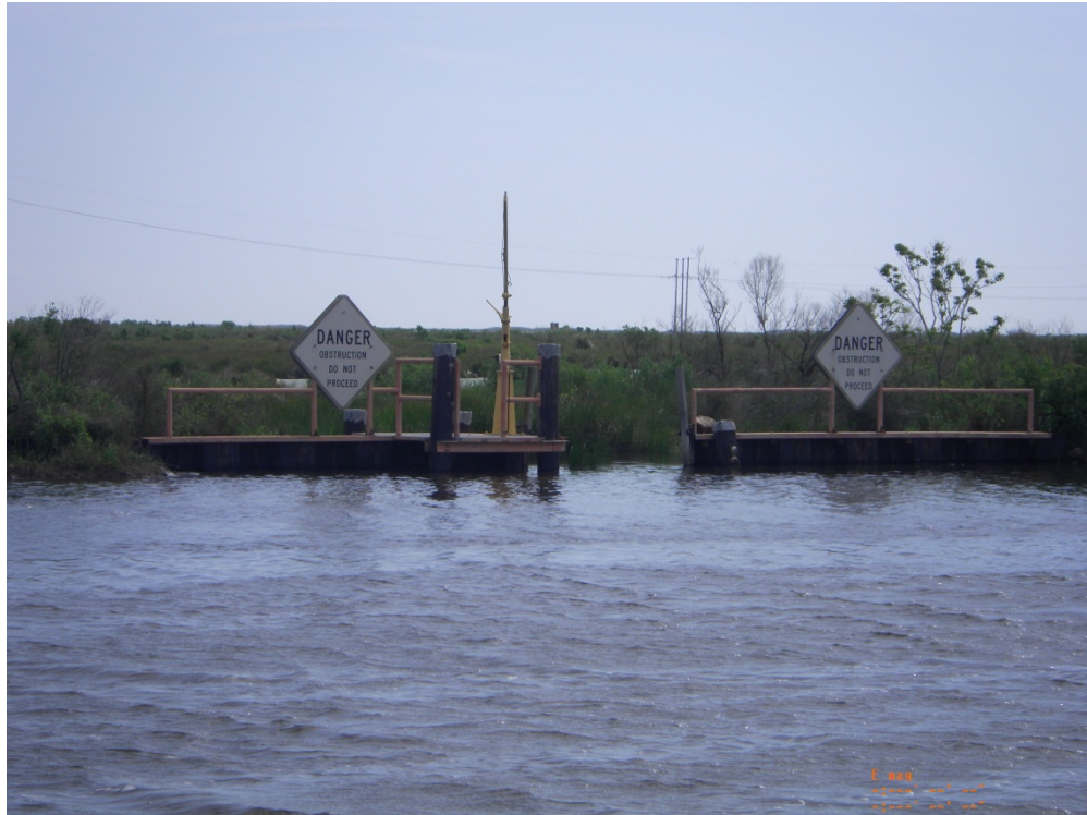
Photo 29: Overall view of Structure 35 variable crest weir, looking northeast
