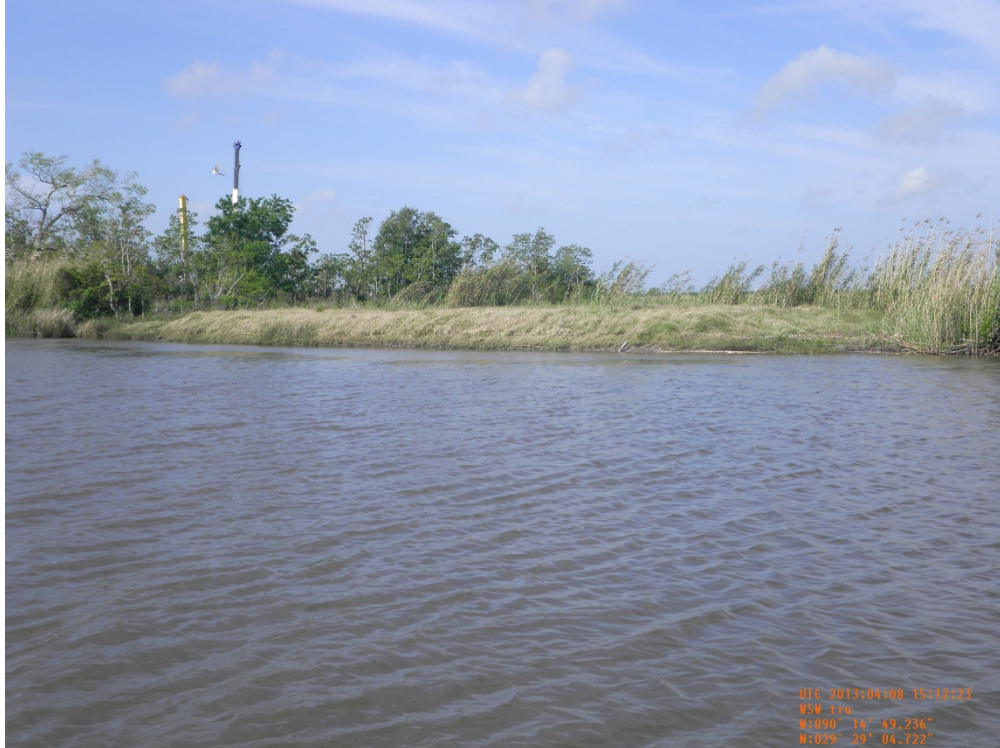
Photo 11: View of Breach Closure No. 4 which was part of the 2012 Maintenance Project
