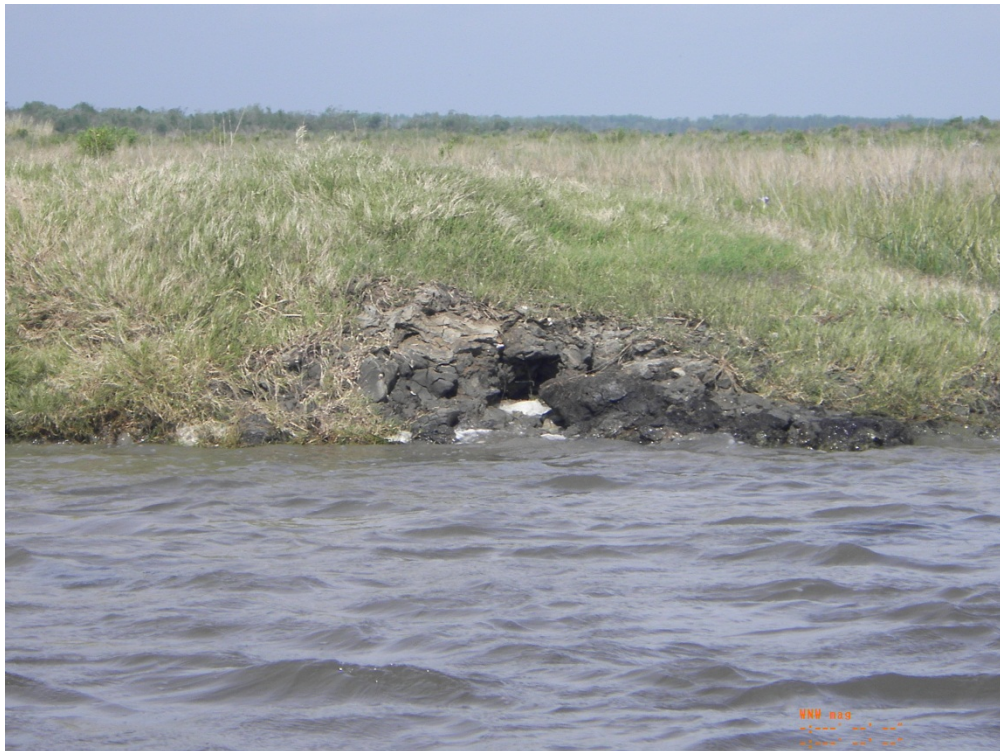
Photo 28: View of Breach Closure No. 1 which was part of the 2012 Maintenance Project
