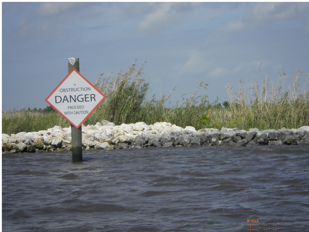
Photo 48: View of new warning sign and transition between Structure 4 and Rock Dike Extension
