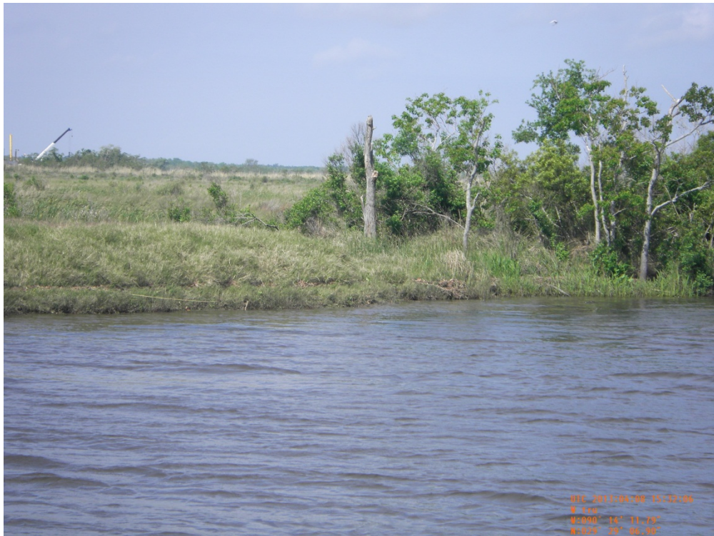
Photo 26: View of Breach Closure No. 3 which was part of the 2012 Maintenance Project
