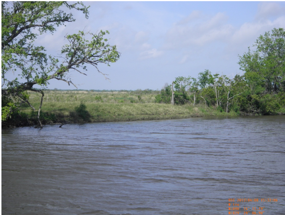
Photo 24: View of Breach Closure No. 3 which was part of the 2012 Maintenance Project
