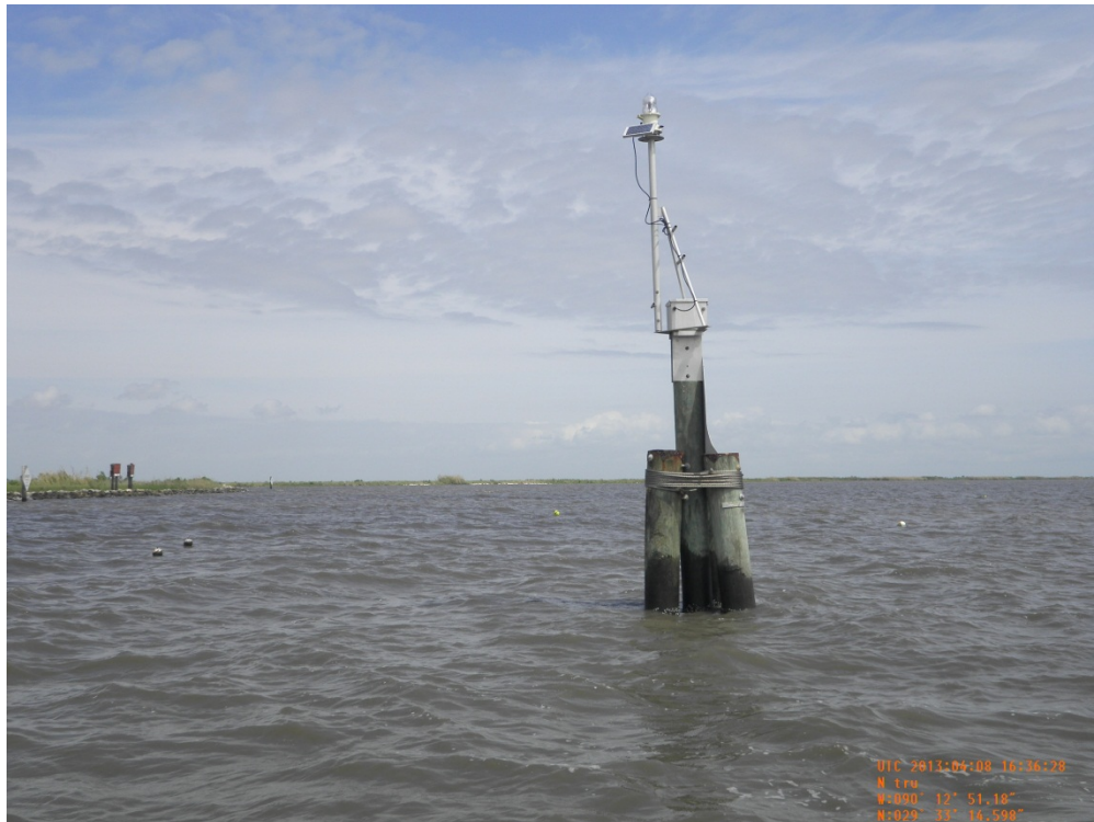
Photo 60: View of navigational light installed on the timber pile cluster at Structure 14
