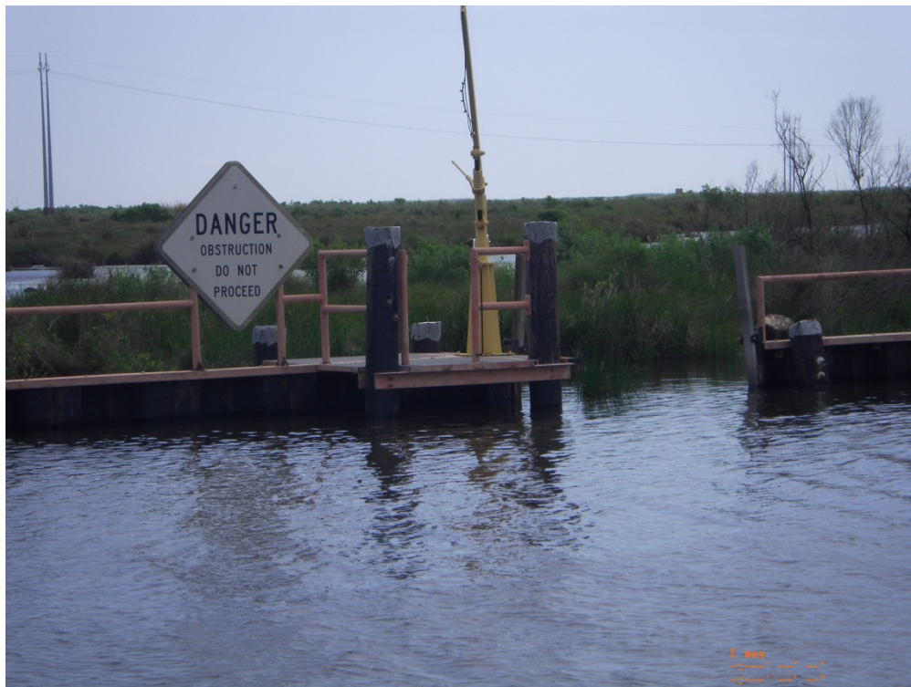
Photo 30: Close up view of Structure 35 warning signs, railings, steel bulkhead, and operating crane
