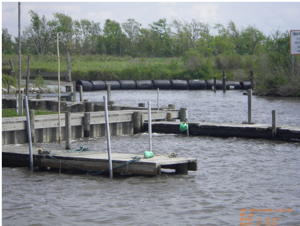
Photo 56: View of Structure 8 rock riprap channel plug, looking north
