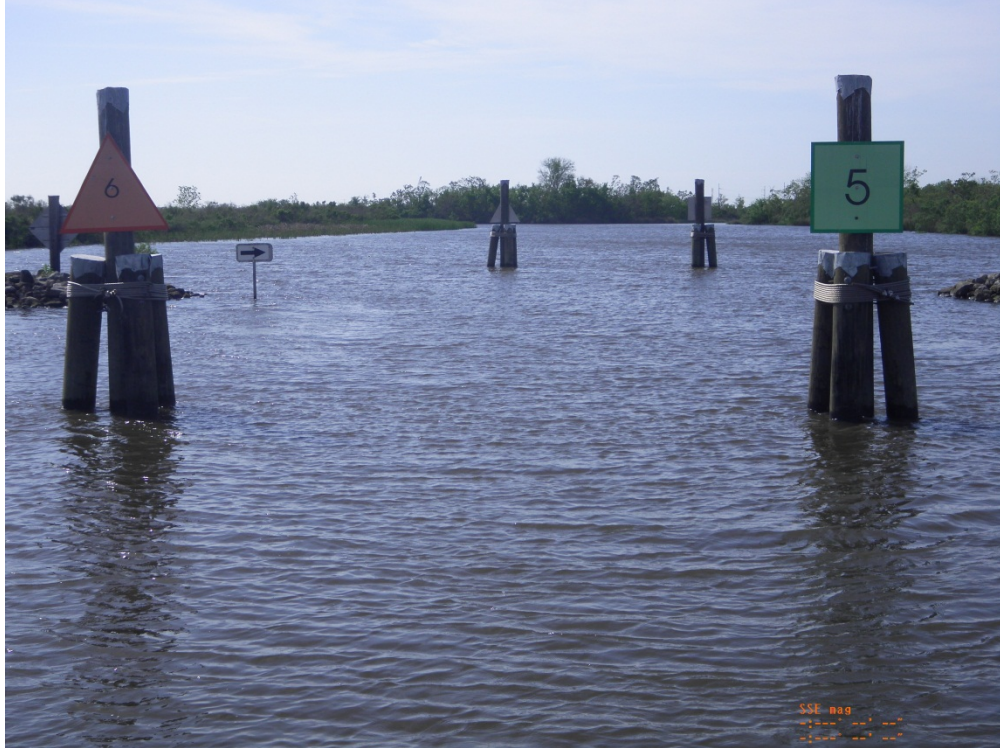
Photo 7: View of the newly installed timber pile clusters and signs on the north side of Structure 1
