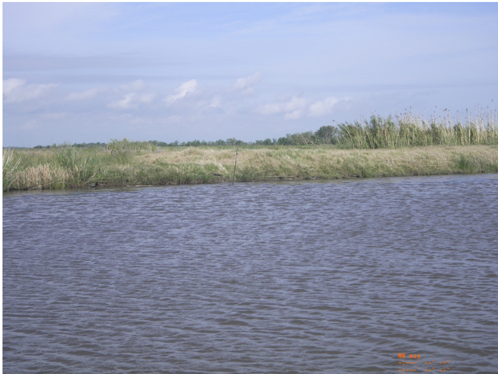
Photo 12: View of Breach Closure No. 4 which was part of the 2012 Maintenance Project
