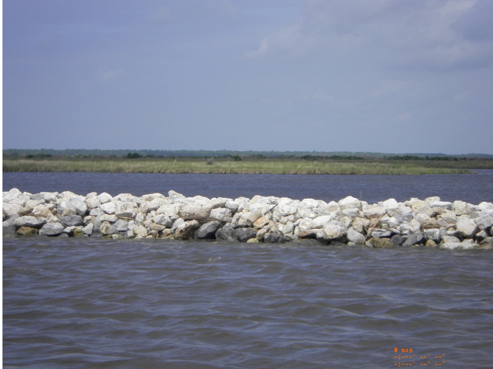
Photo 35: View of the Lake Rim rock dike refurbishment from Breton Canal, looking northwest
