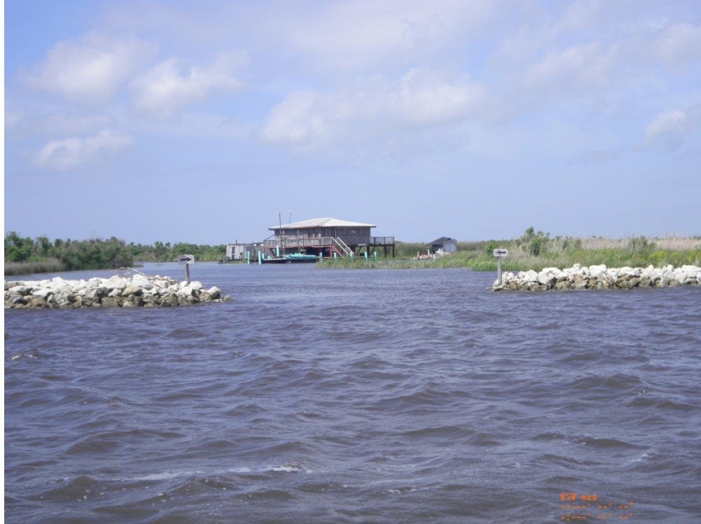
Photo 47: Overall view of Structure 4 fixed crest rock weir with boat bay, looking west
