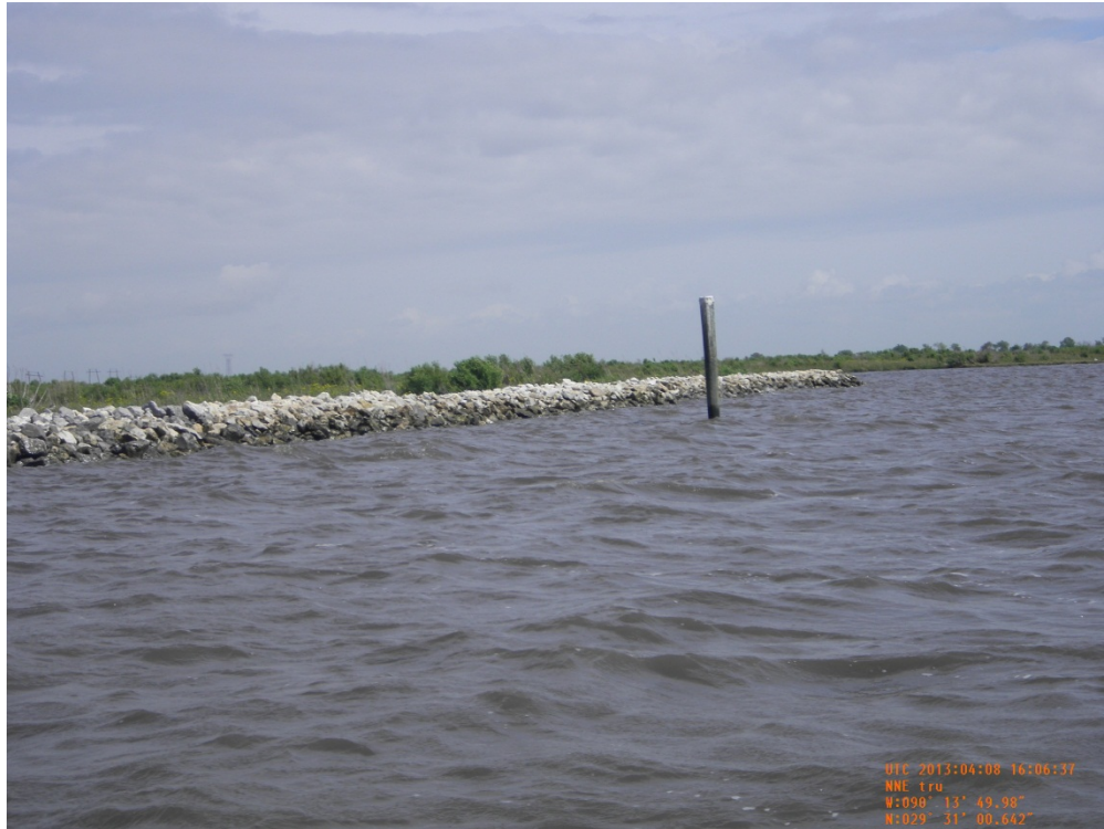
Photo 51: View of Structure 4A&4B rock recap along Little Lake, looking north
