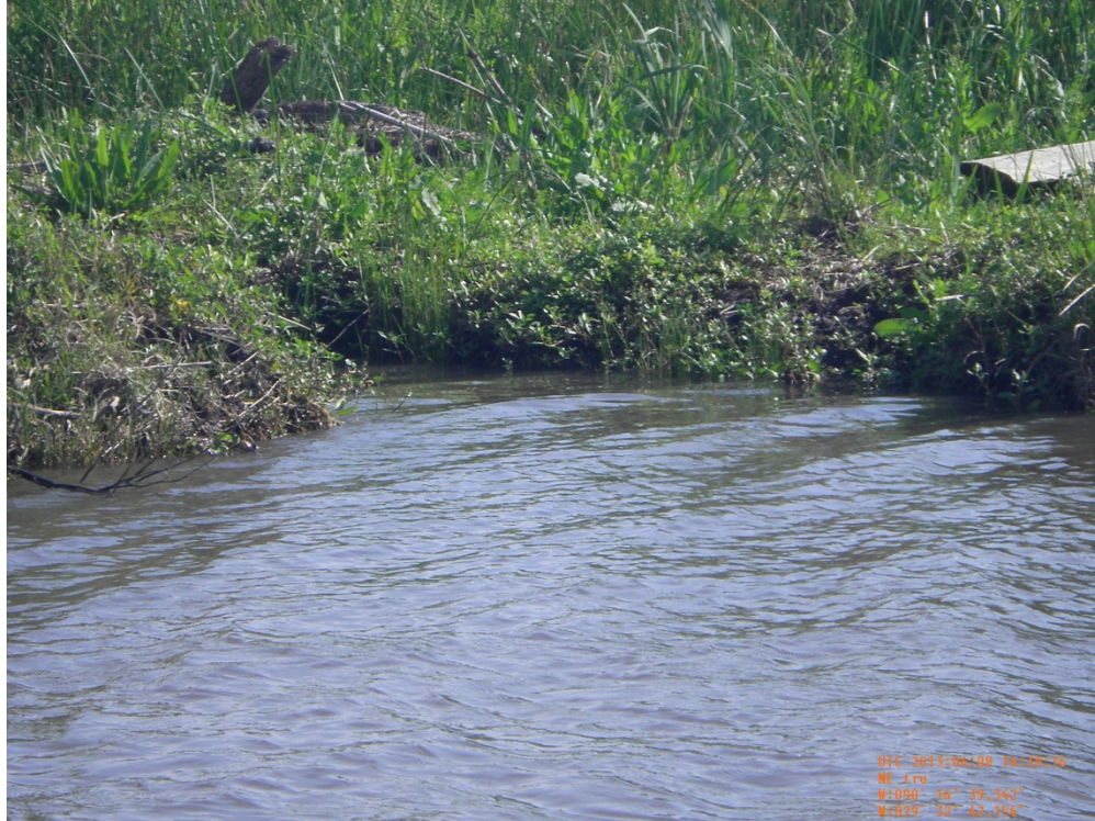
Photo 1: View of small breach around the east side of Structure 43
