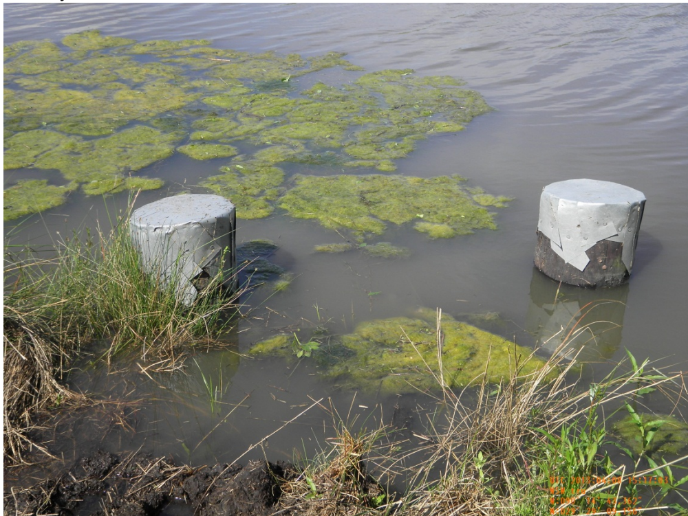
Photo 15: Galvanized pile caps installed on canal side of Structure 91 as part of 2012 Maintenance Project
