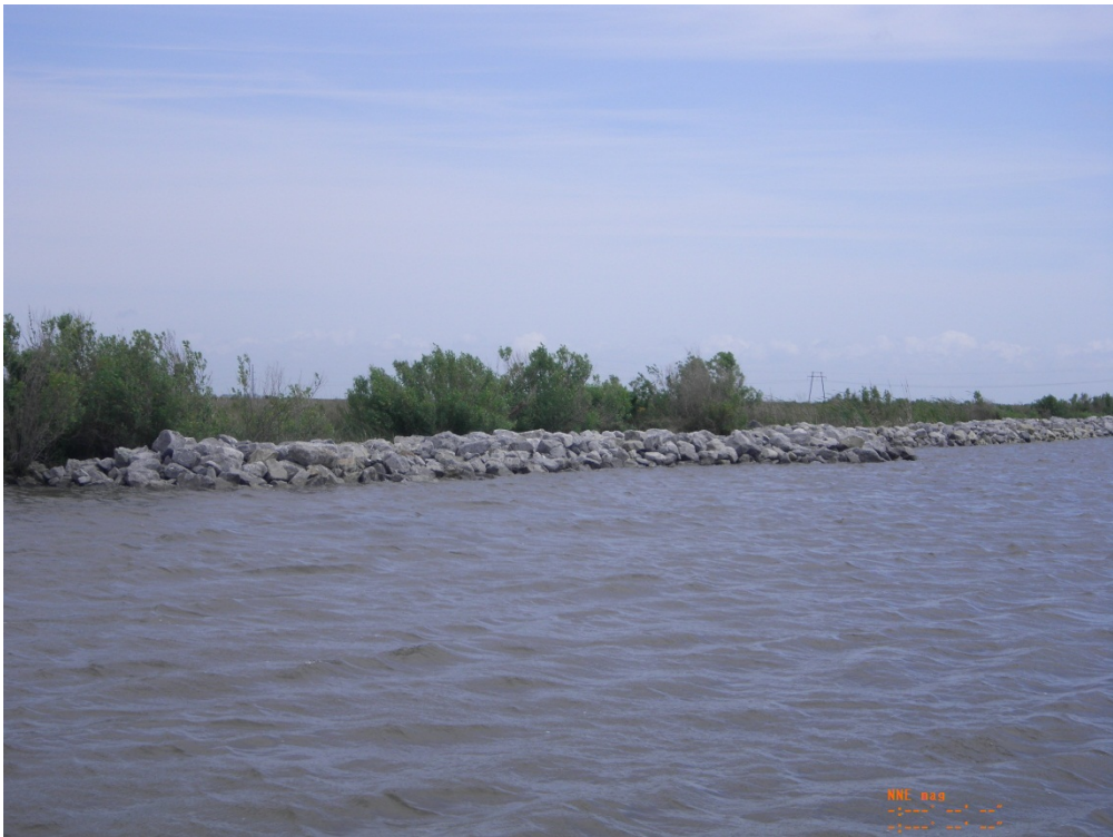
Photo 32: View of the Lake Rim rock dike refurbishment from Breton Canal, looking north
