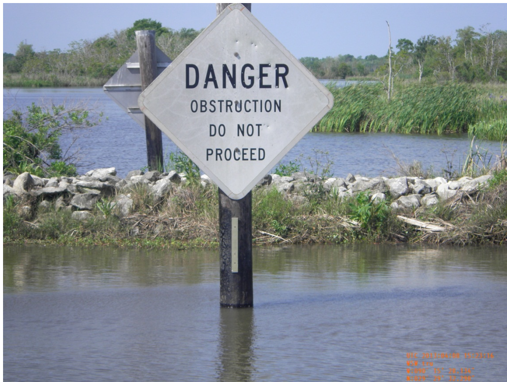
Photo 20: Close of view of the warning signs and supports of Structure 90
