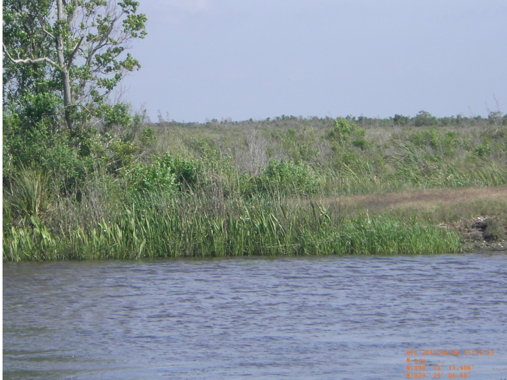
Photo 23: View of Breach Closure No. 2 which was part of the 2012 Maintenance Project
