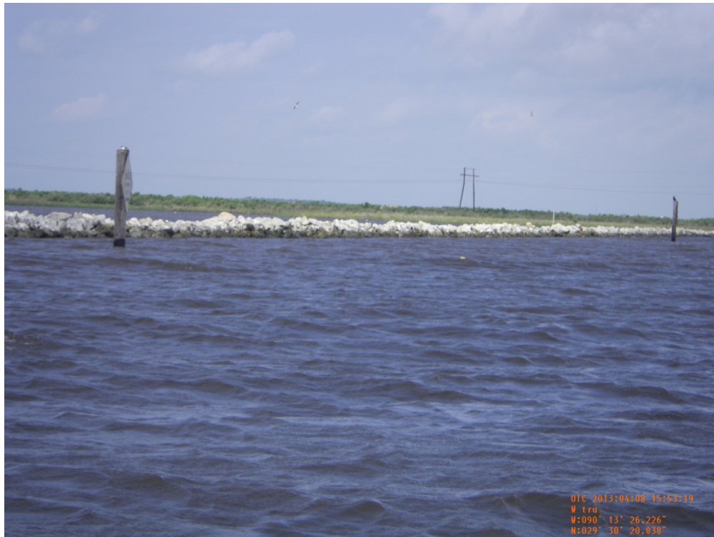
Photo 38: View along the Lake Rim rock dike refurbishment from Little Lake, looking west
