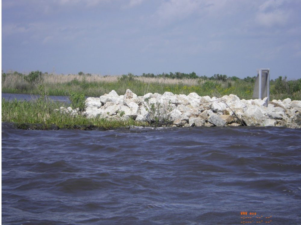
Photo 45: View of the warning sign and embankment tie-in on the south side of Structure 4
