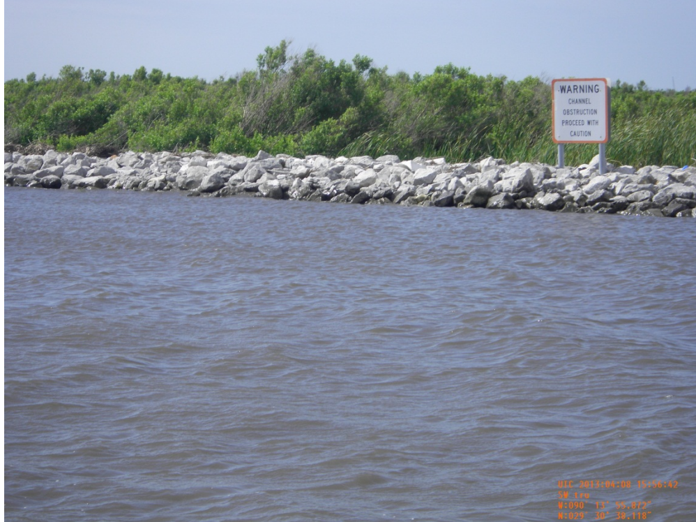
Photo 41: View of warning sign and rock recap on the southern side of Structure 2
