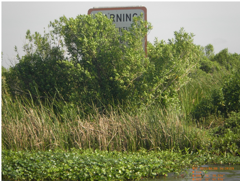
Photo 2: View of Structure 43 looking north. The rock plug is not visible through the vegetation.
