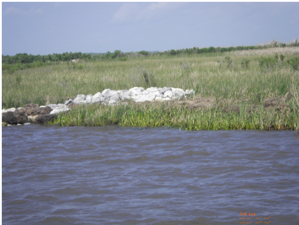
Photo 44: View of the embankment tie-in on the northern side of Structure 2
