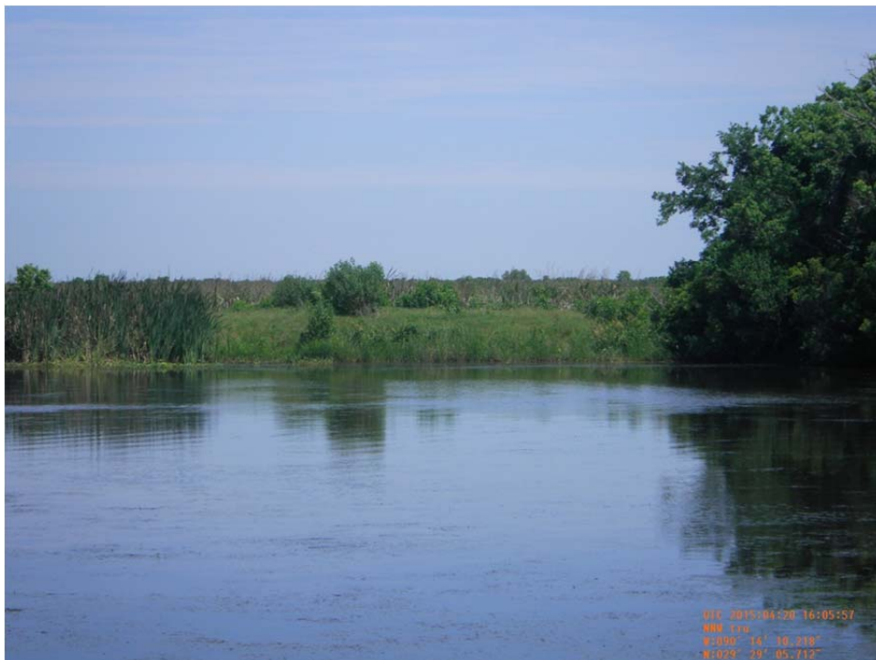
Photo 34: Breach location (Identified in as-built drawings as Breach 2) repaired in 2012 along the second location canal from Bay L' Ours via Breton Canal.
