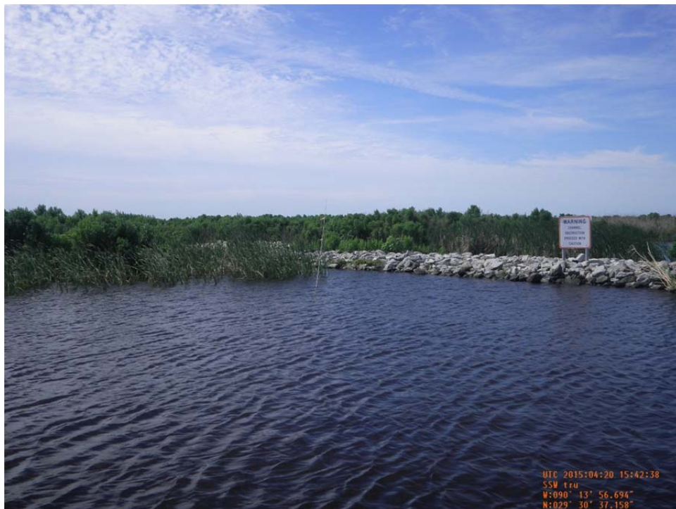
Photo 22: View of the south side of the rock weir at Structure No.2
