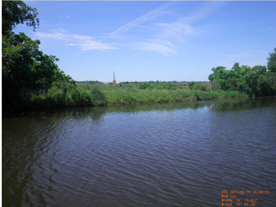
Photo 35: Breach repaired in 2012 (identified as Breach 3) off of third location along Breton Canal from By L' Ours.
