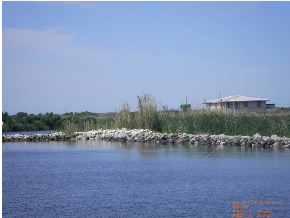
Photo 17: View of rock dike closure tie-in to the north side of Structure No.4 constructed in 2012.
