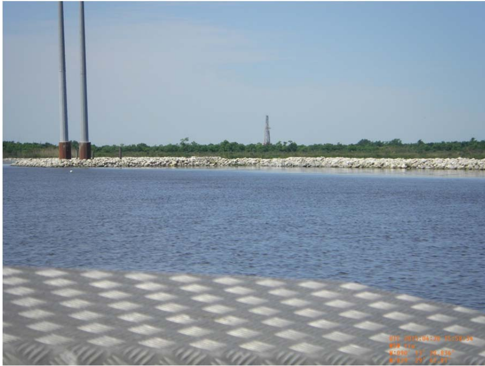
Photo 29: View of the rock dike along the north bank of Breton Canal near transmission power line.
