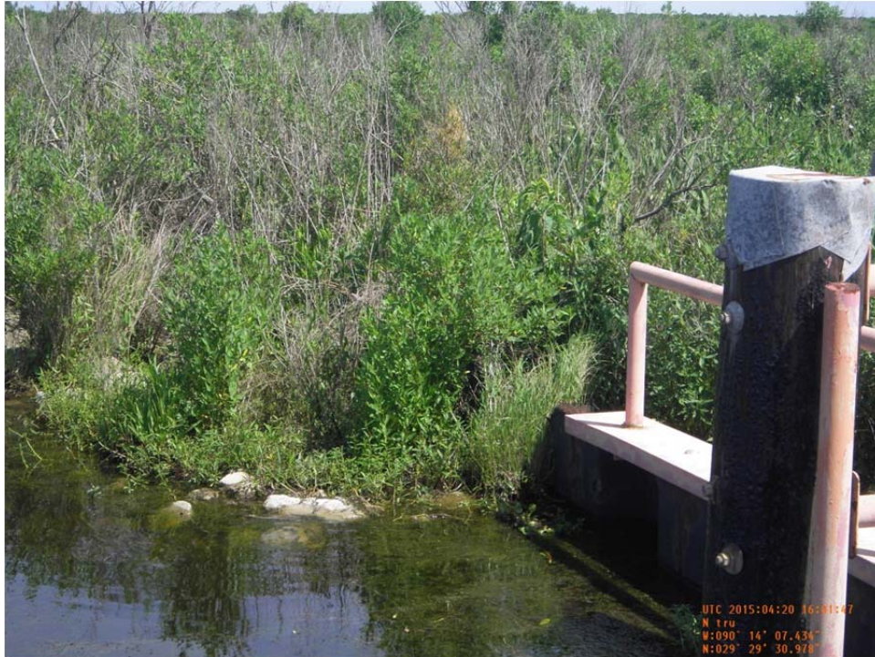
Photo 33: View of steel sheet pile weir and bank tie-in on the NE side of Structure No.35.
