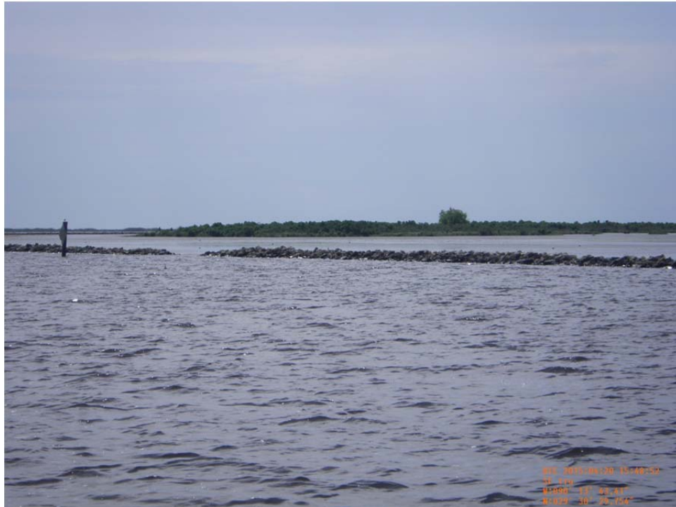
Photo 25: View of rock dike lake rip along the south shoreline of Bay L' Ours.
