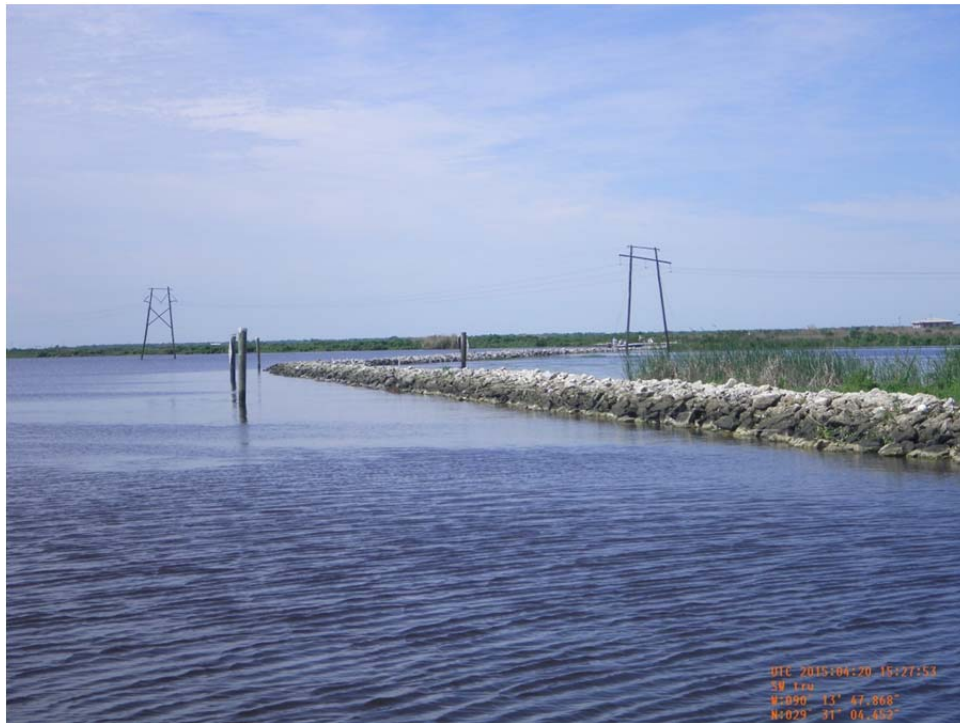
Photo 13: rock plug (Structure 4A & 4B) and rock dike extension to Structure 4 construction in 2012.
