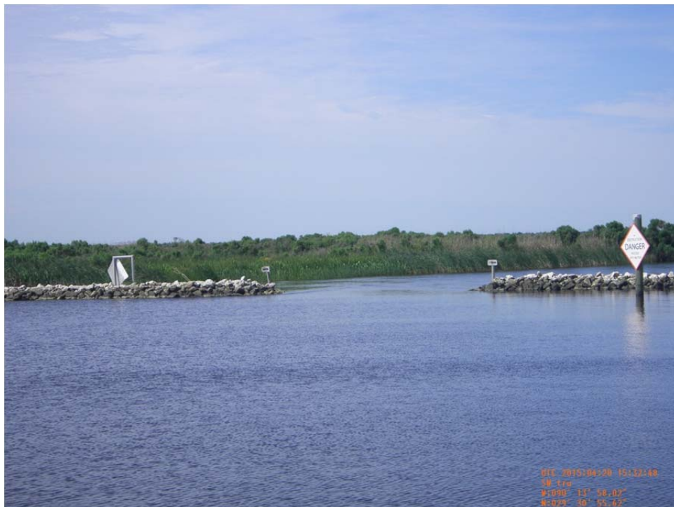
Photo 18: Overall view of rock weir with boat bay at Structure No.4.
