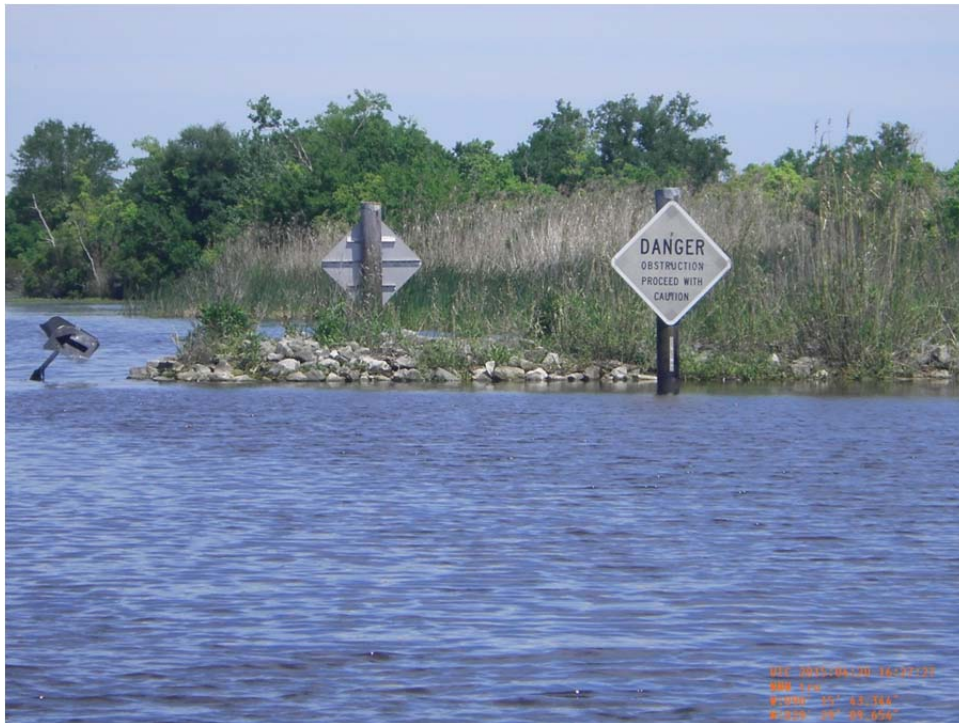
Photo 44: view of the rock weir on the east side of Structure No.1 and warning signs.
