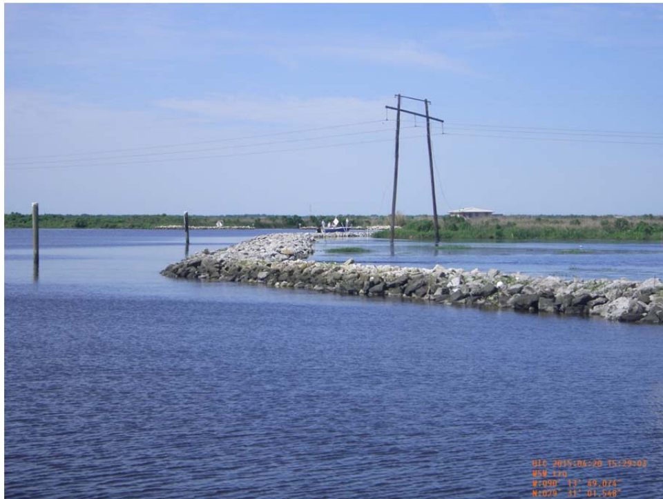
Photo 15: View of rock dike closure between Structure 4B and Structure 4 constructed in 2012.
