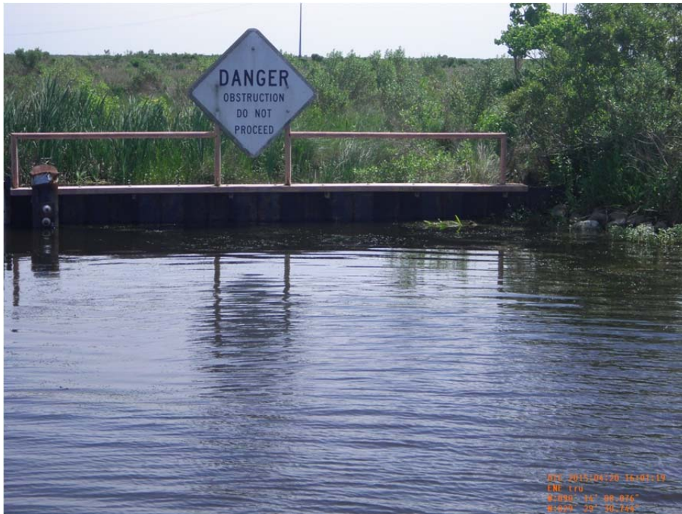
Photo 32: view of sheet pile weir and bank tie-in on the SW side of Structure No.35.
