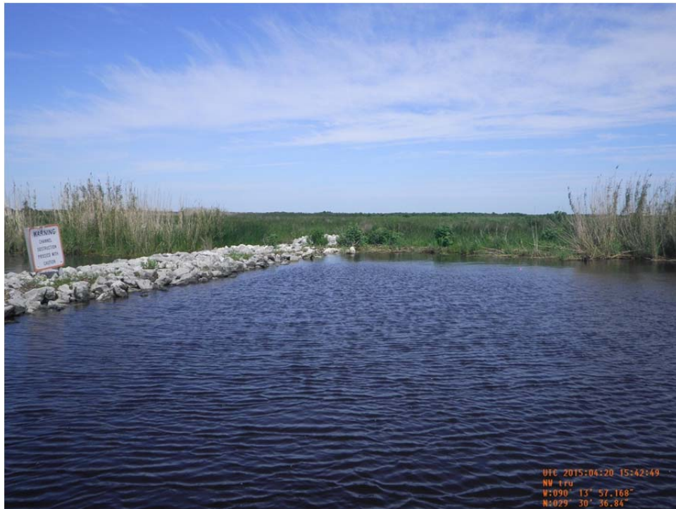
Photo 23: View of north side of rock weir at Structure No.2.
