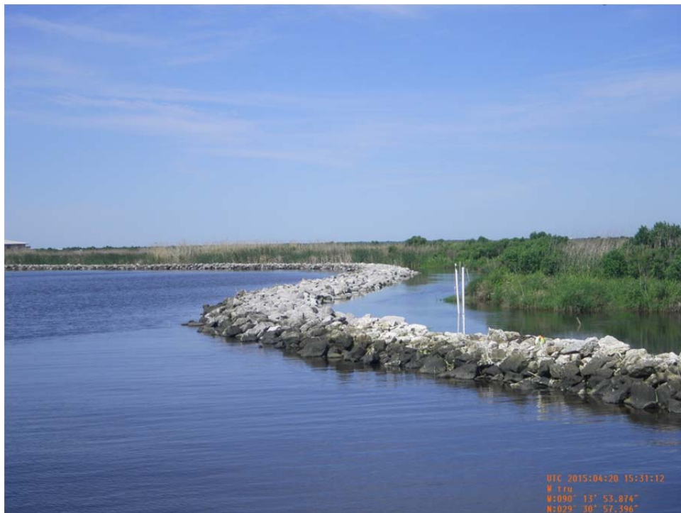
Photo 16: View of rock dike closure between Structure 4B and Structure 4 constructed in 2012.
