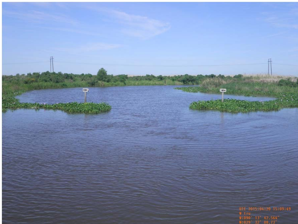
Photo 8: Overall view of the rock weir with boat bay of Structure No.7.
