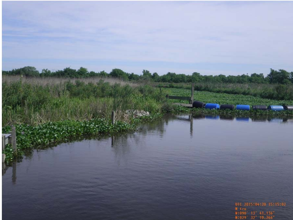
Photo 9: View of rock weir and floating barrel gate at Structure No. 8.
