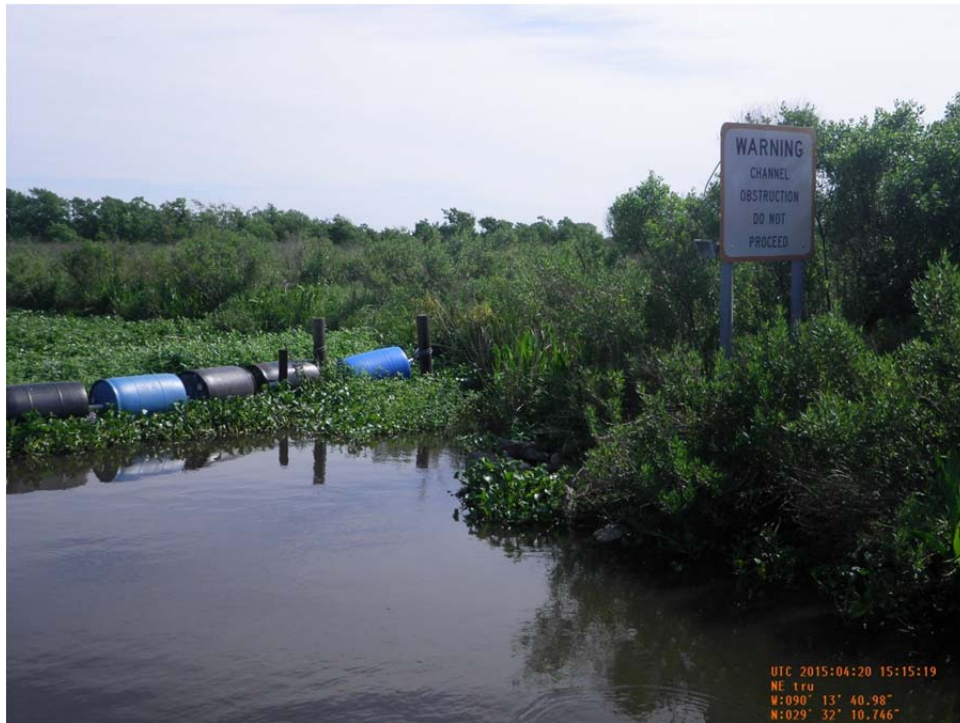
Photo 11: Viwe of the east side of rock weir and floating barrel gate closure of Structure No.8.
