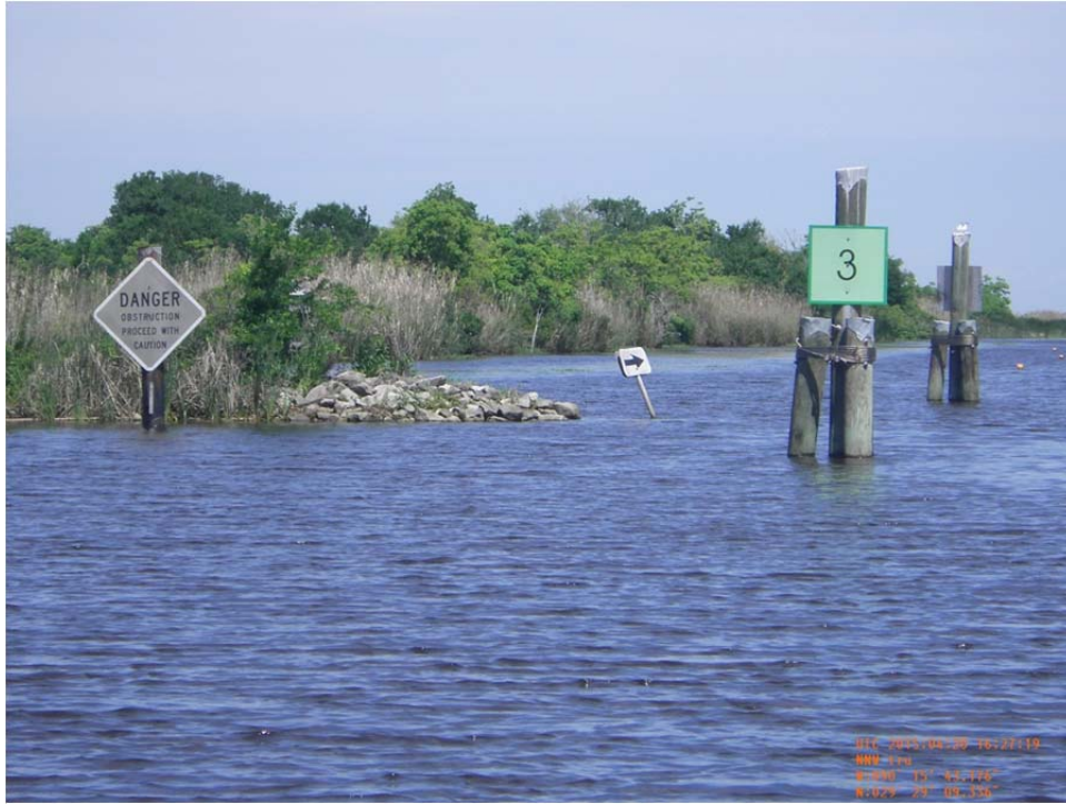
Photo 43: View of rock weir on the west side, warning signs and barge bay opening at Structure No.1 located along Superior Canal.
