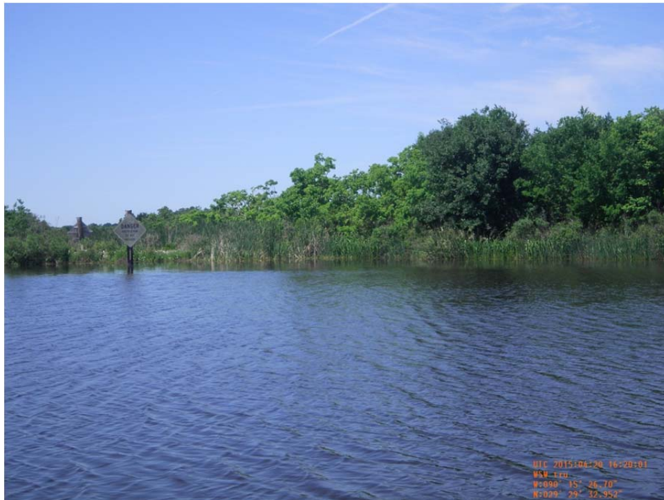
Photo 41: View of rock dike plug and warning signs at Structure No.90.
