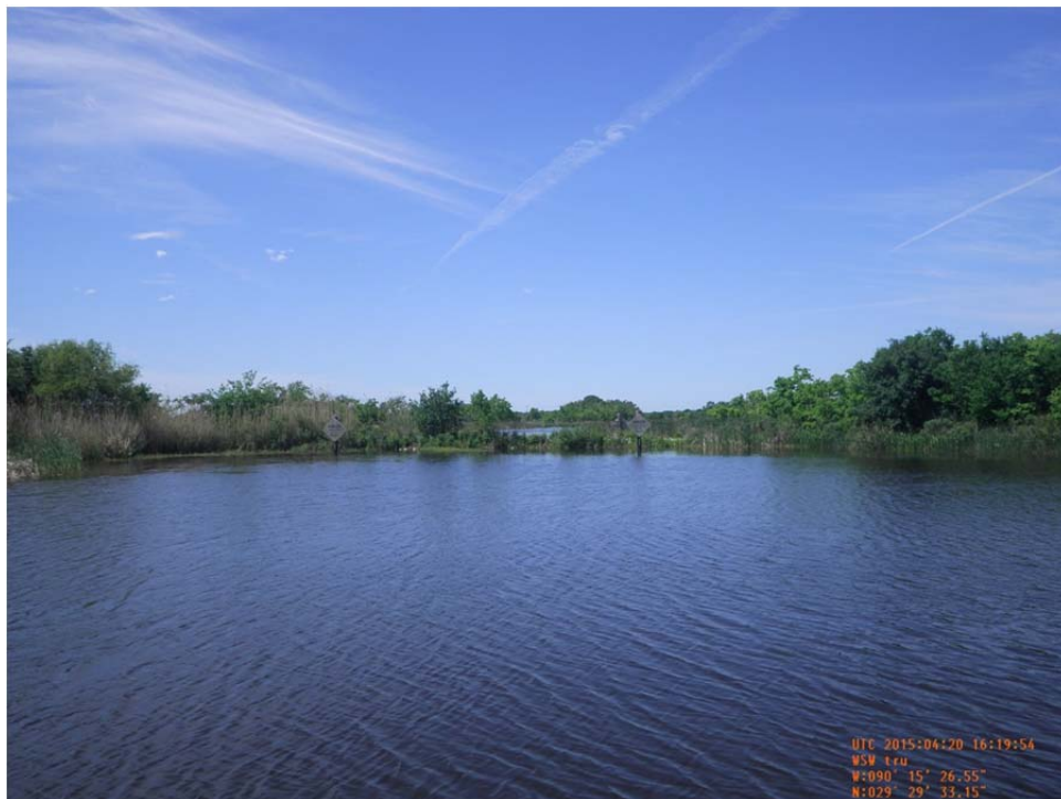
Photo 40: Overall View of Structure 90, a rock rip rap channel plug located in the second location canal on the east bank of Superior Canal from the Hurricane Protection Levee.
