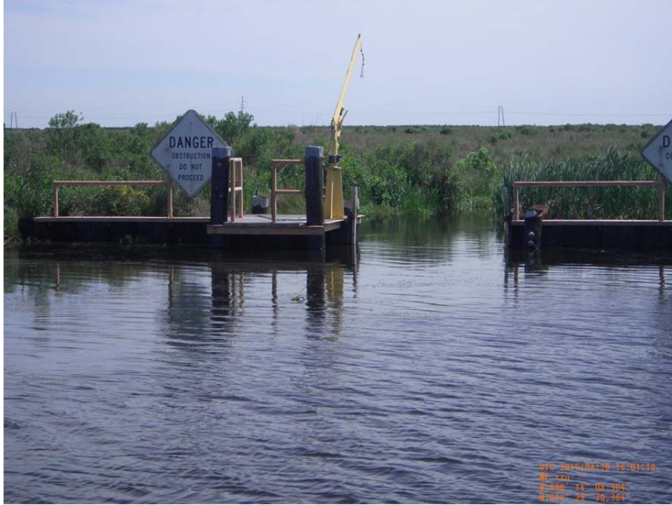
Photo 31: View of variable crest weir Structure No.35 on north bank of location canal off of Breton Canal.
