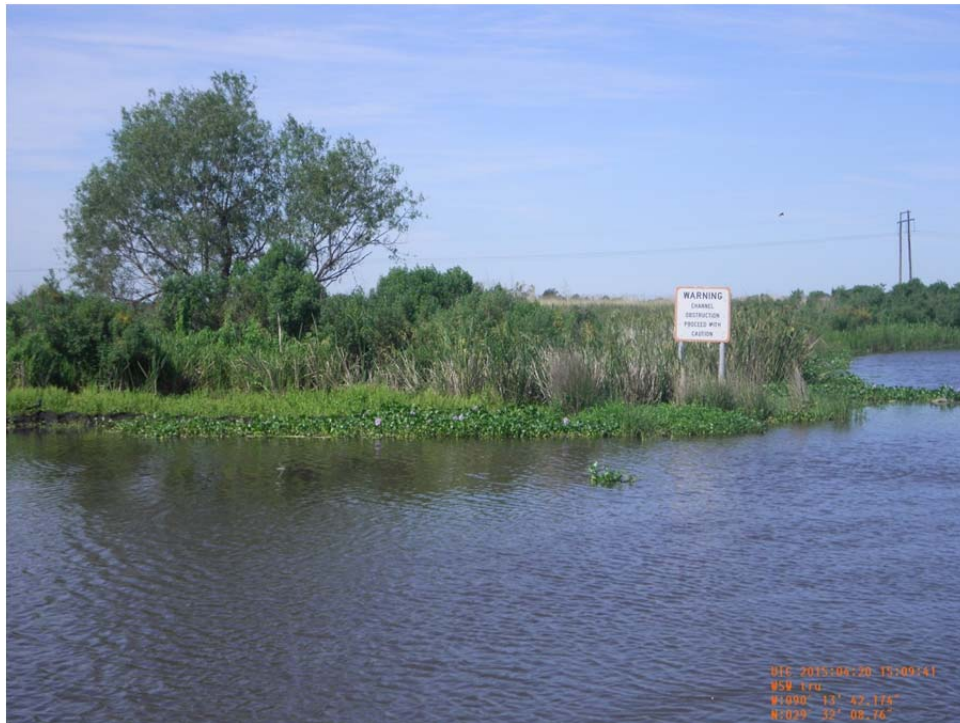
Photo 7: View of rock weir on the south side of boat bay on Structure No.7.
