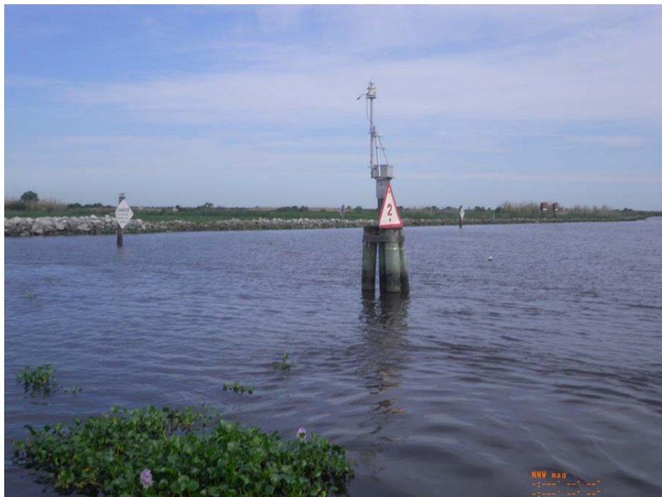
Photo 4: View of navigation aid lights on the NE side of Structure 14a and rock weir in background.
