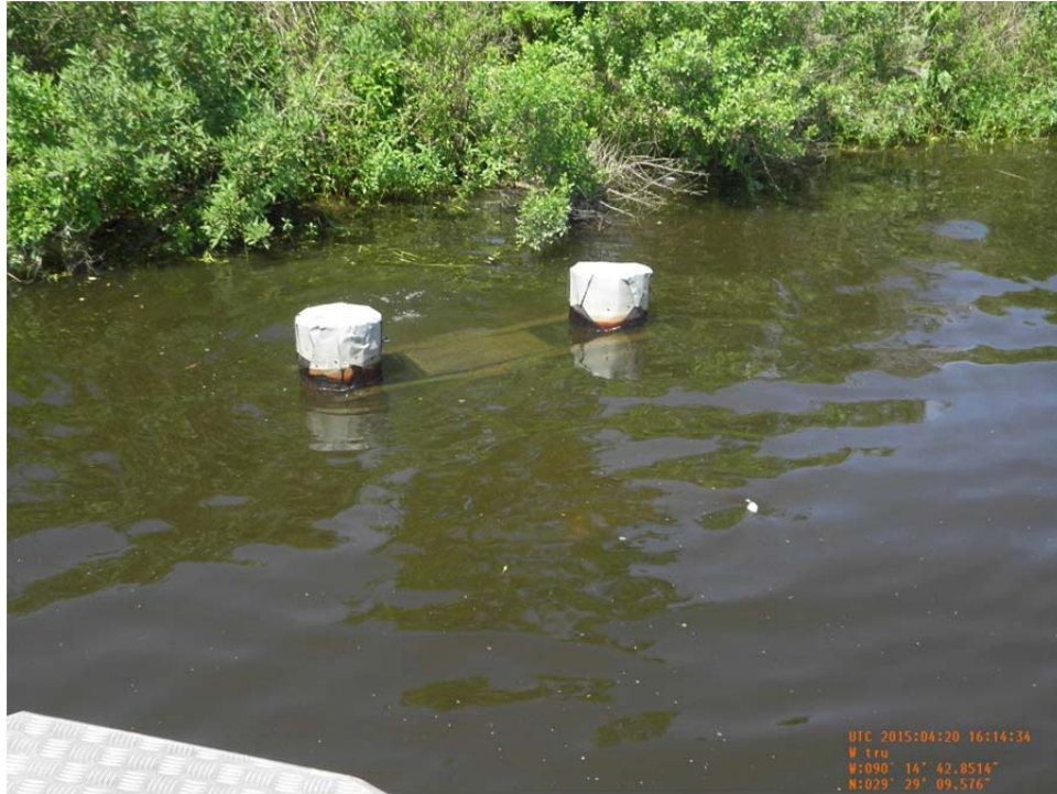
Photo 39: View of corrugated metal pipe support and flap gate at Structure No.91.
