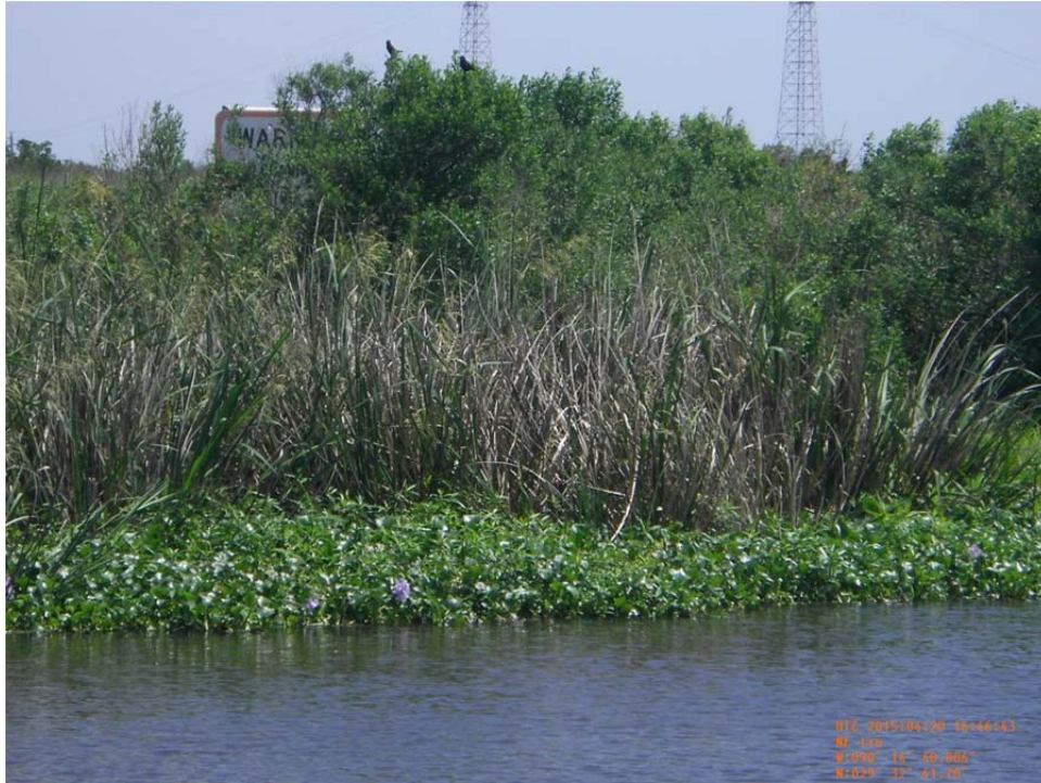
Photo 47: View rock rip rap channel plug (Structure 43) located along Bayou Des Amoreaux.
