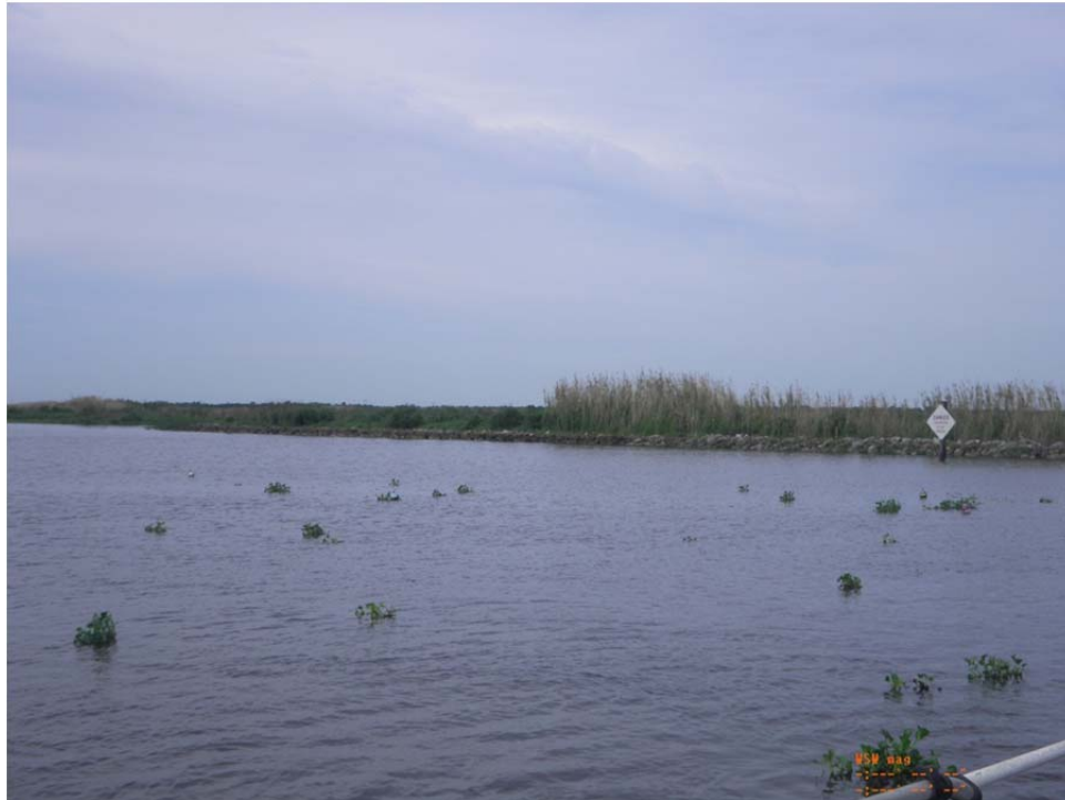
Photo 5: view of the rock weir on the south side of Structure No. 14A.
