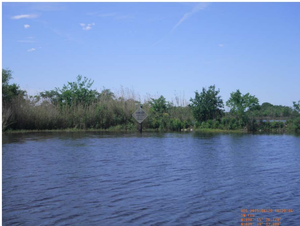
Photo 42: View of rock dike plug and warning signs at Structure No.90.
