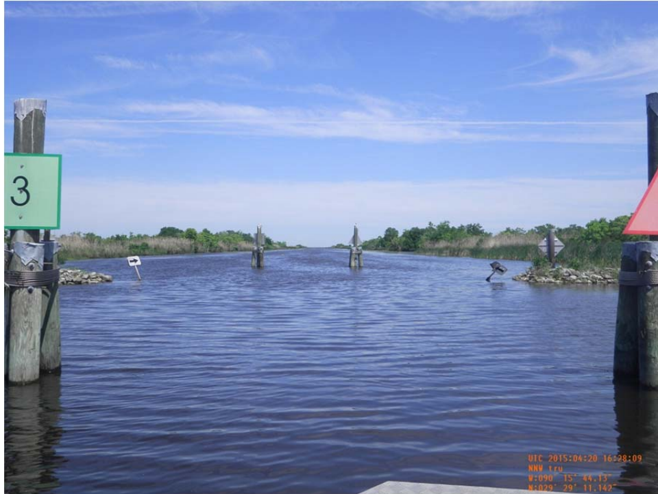
Photo 45: View of barge bay opening and timber warning signs at Structure No.1.
