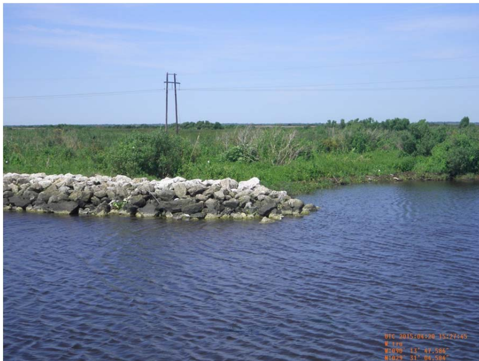
Photo 12: View of the north end of rock plug tie-in at Structures 4A and 4B.
