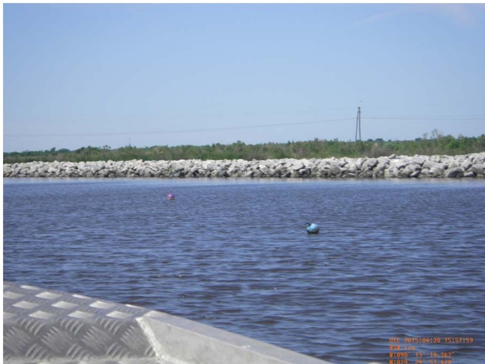
Photo 28: View of the rock dike along the north bank of Breton Canal.
