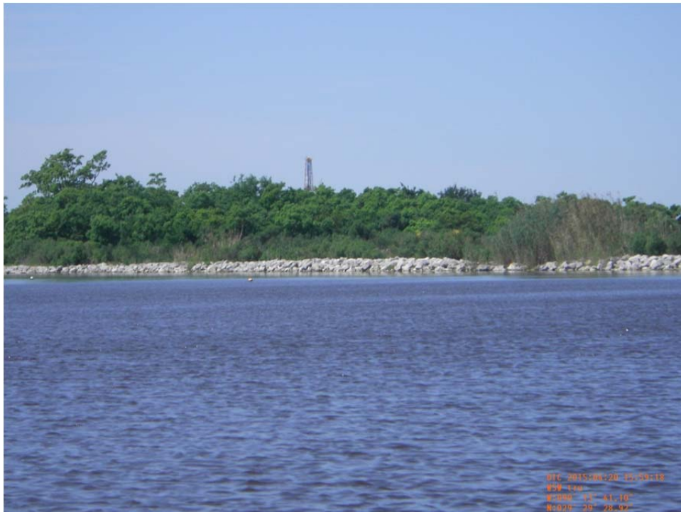
Photo 30: View of rock dike along the north bank of Breton Canal near the first location canal.
