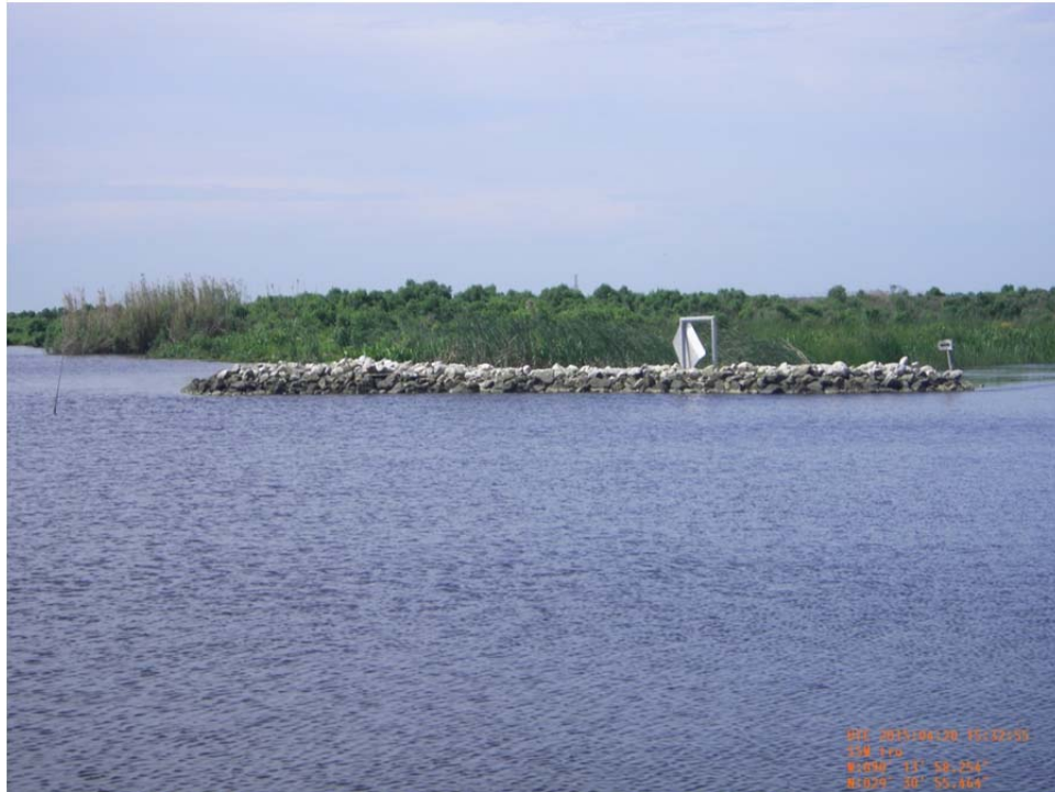
Photo 19: View of the rock weir on the south side of the boat bay of Structure No.4.
