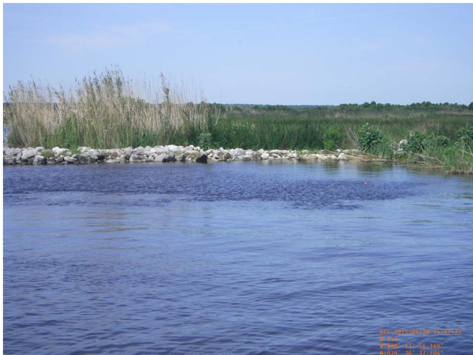
Photo 20: View of the rock weir on the north side of the boat bay of Structure No.2.
