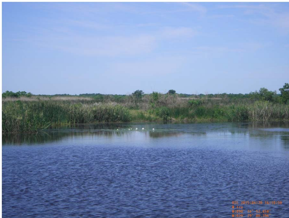
Photo 36: Breach repaired in 2012 (labeled Breach 4) off of third location along Breton Canal from Bay L' Ours.
