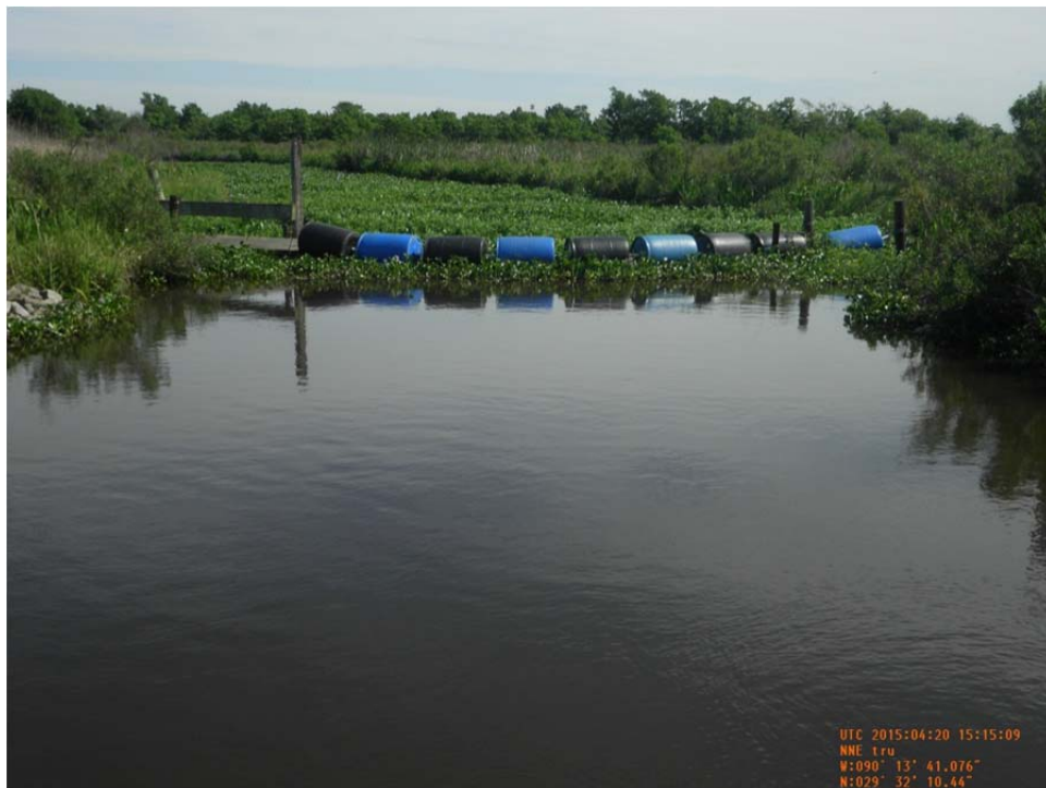
Photo 10: View of rock weir and floating barrel gate at Structure No.8.
