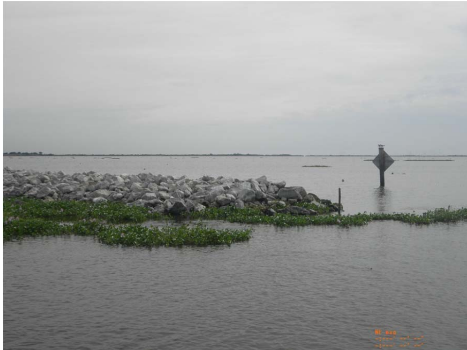
Photo 3: View of rock Weir at the barge bay on the north side of Structure 14A.
