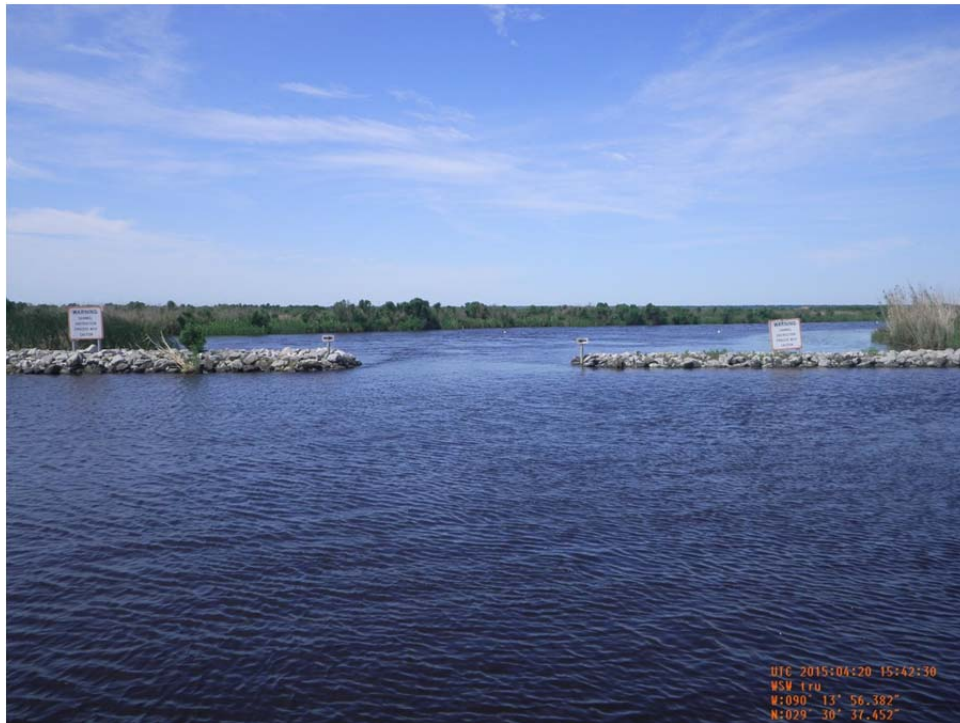
Photo 21: Overall view of the rock weir with boat bay at Structure No.2
