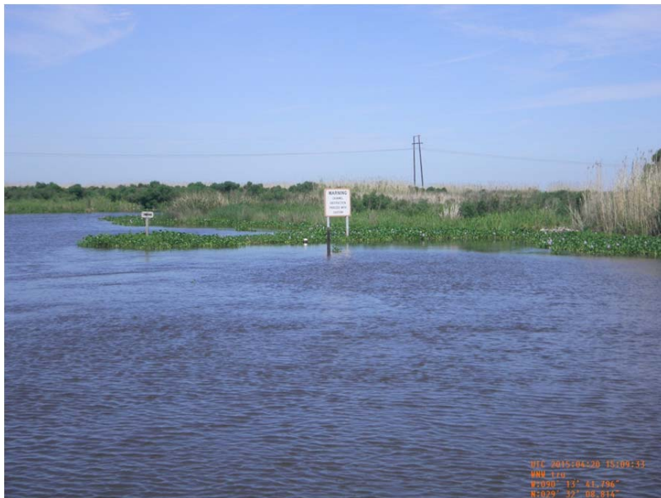
Photo 6: View of the rock weir on the north side of the boat bay on Structure No. 7.
