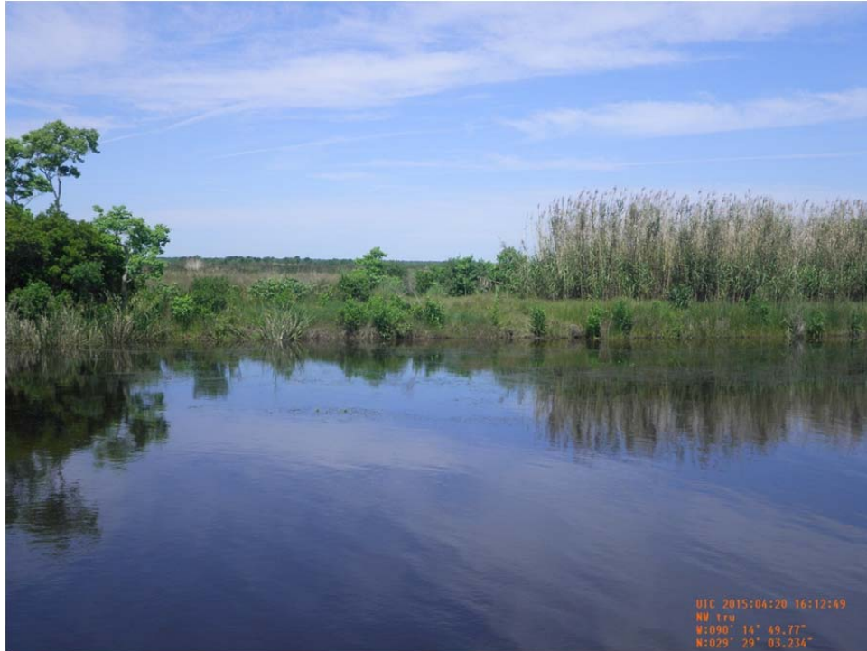
Photo 37: - Breach repaired in 2012 (labeled Breach 5) off of third location along Breton Canal from Bay L' Ours.
