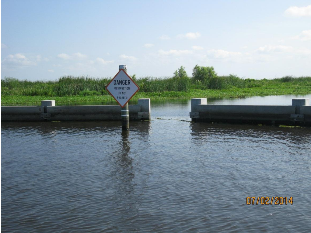
Photo #3 – CU #4 Concrete Panel Wall
