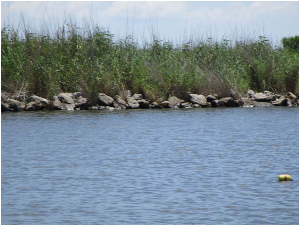
Photo # 4 – Accretion & vegetation behind the rock structure
