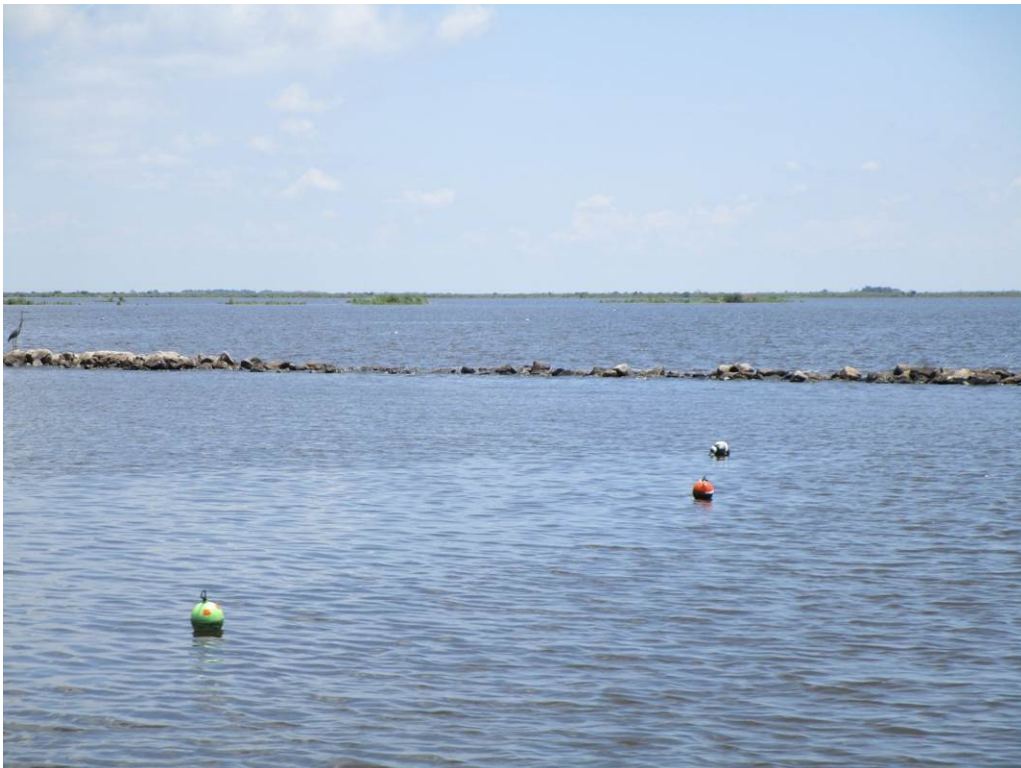
Photo # 2 – Settlement noted in open water area
