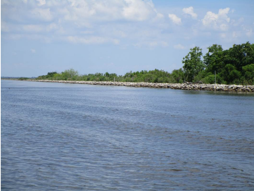
Photo #1 – Shoreline protection rock structure
