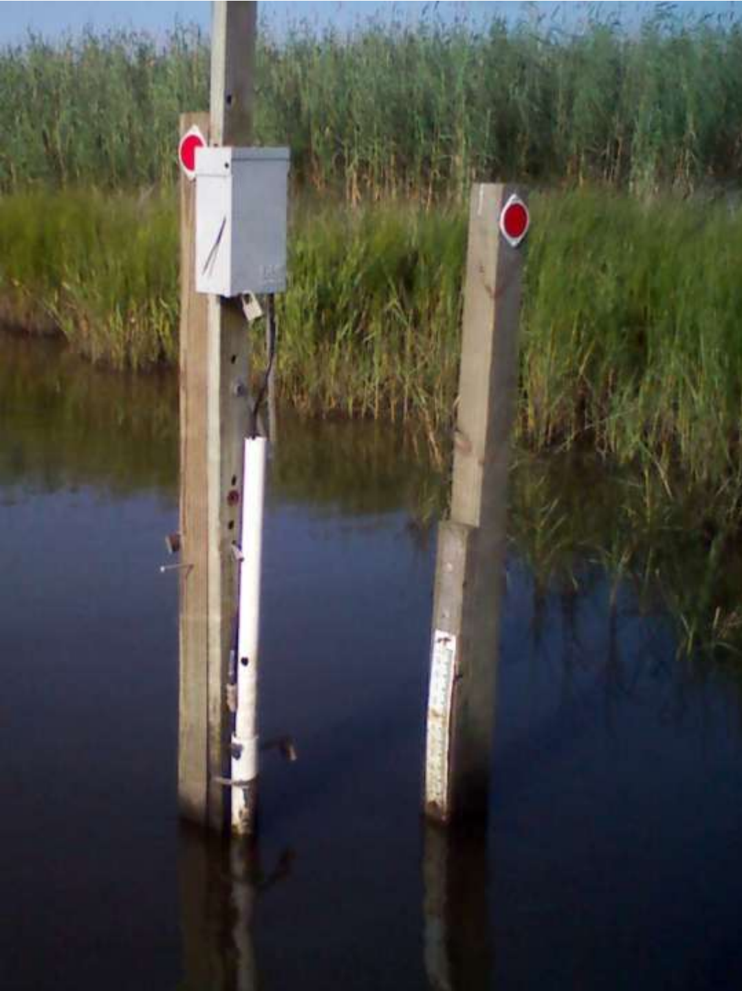
Figure 3.1b. Photograph of a typical wooden post hydro station.
