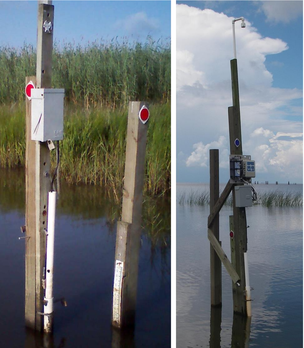
Figure 3.1b. Photographs of typical wooden post hydro stations. The original version is to the left and the newer version is to the right (see Fig. 3.6b for snorkel description).
