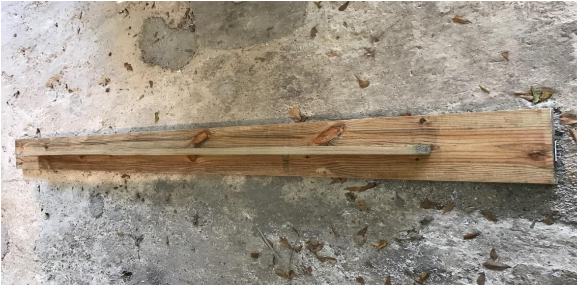
Figure 2.5c. Photograph of a 2"x12"x12' boardwalk plank with a 2"x4"x8' strong-back bracing underneath.
