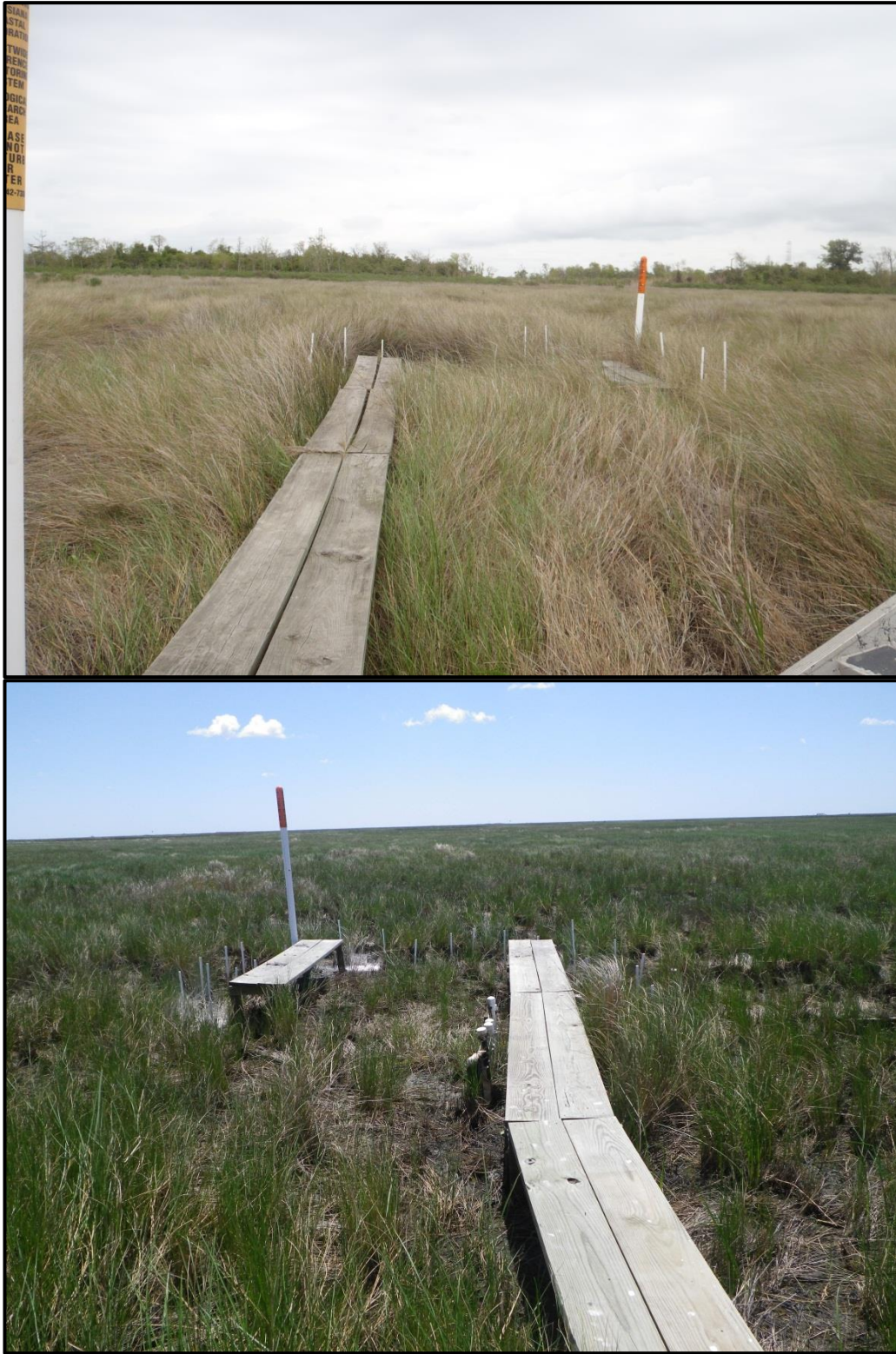
Figure 5.1c. Photographs of boardwalks with access on the left side (top) and right side (bottom).
