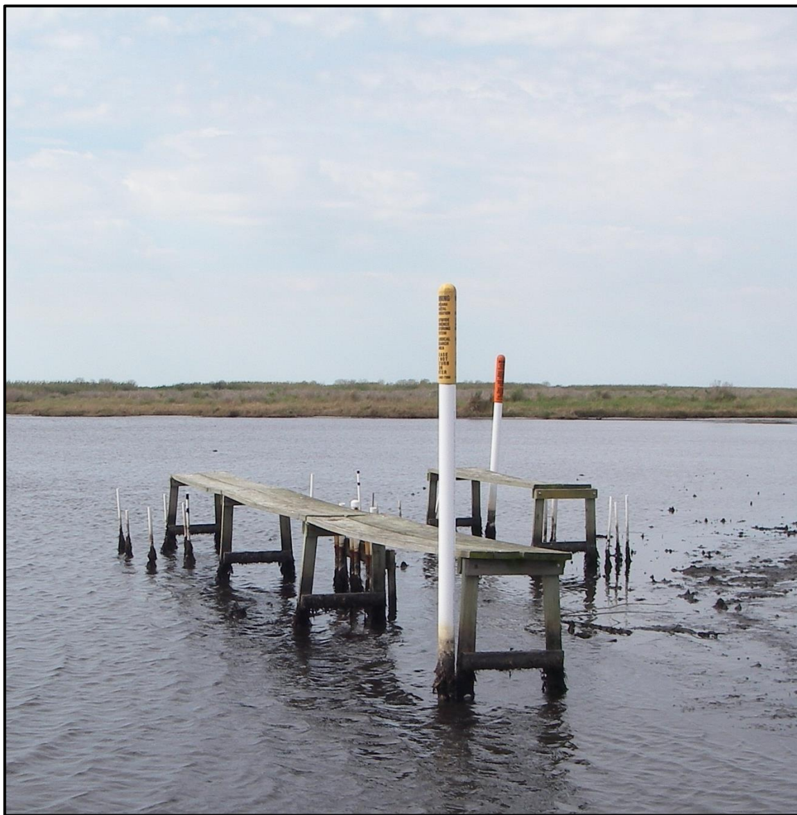
Figure 2.6b. Photograph of a boardwalk in a marsh that washed away. The portion of the teeth that is normally beneath the surface is exposed.
