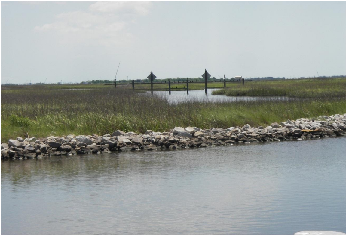
Photo No. 13 , boat barrier, Structure No. 4
