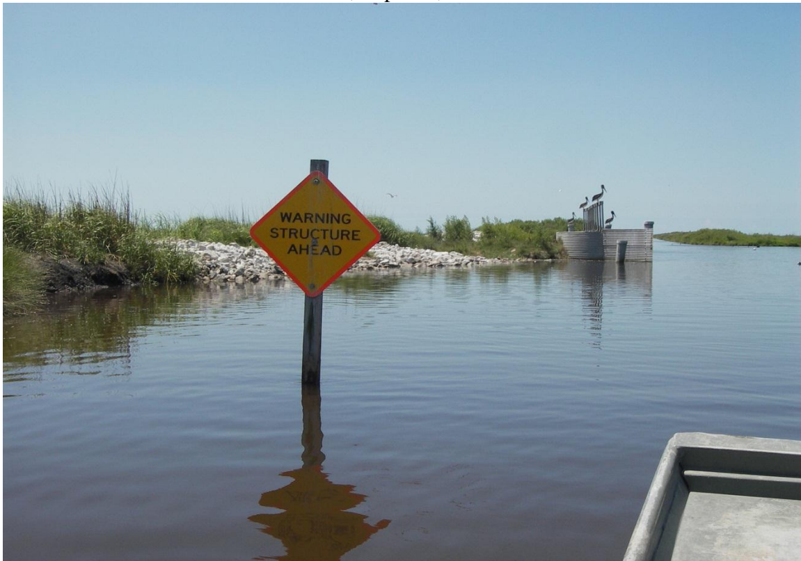
Photo No. 12, Structure No. 4
