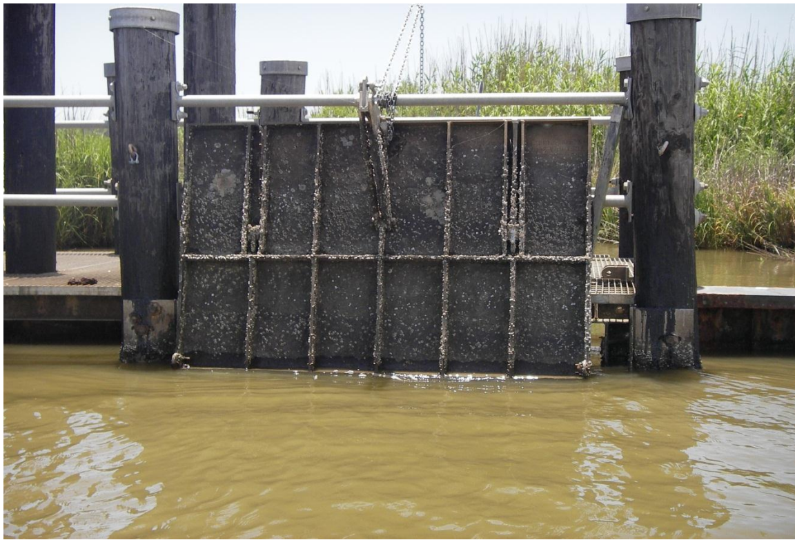
Photo 23 —disconnected flap on Structure 13
