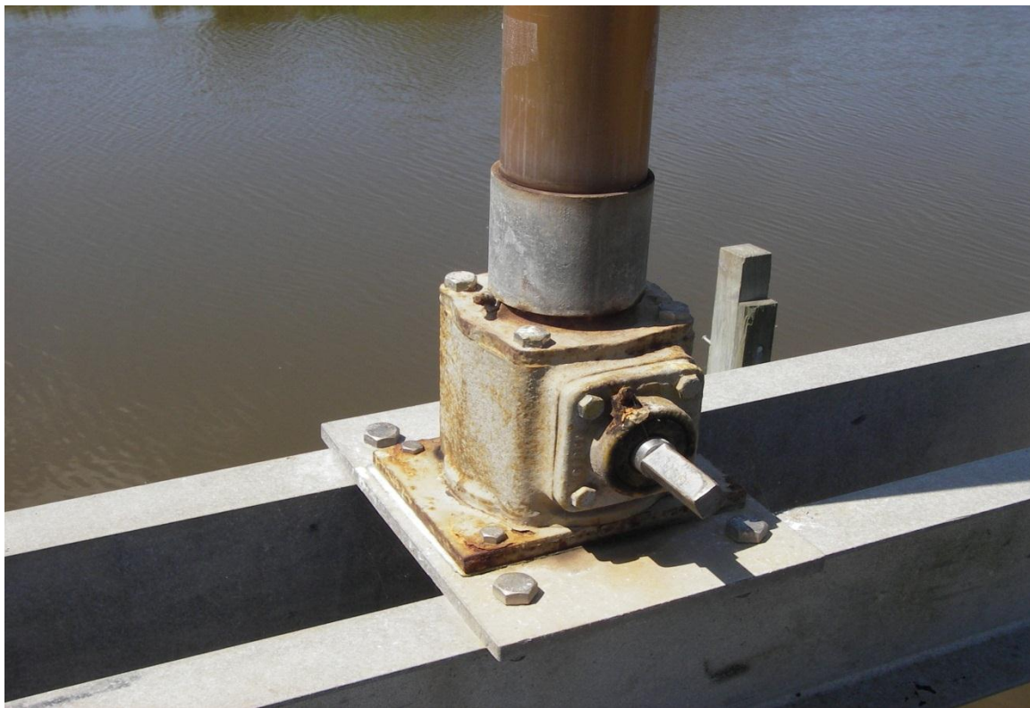
Photo No. 5, sluice gate gear box on Structure 9b
