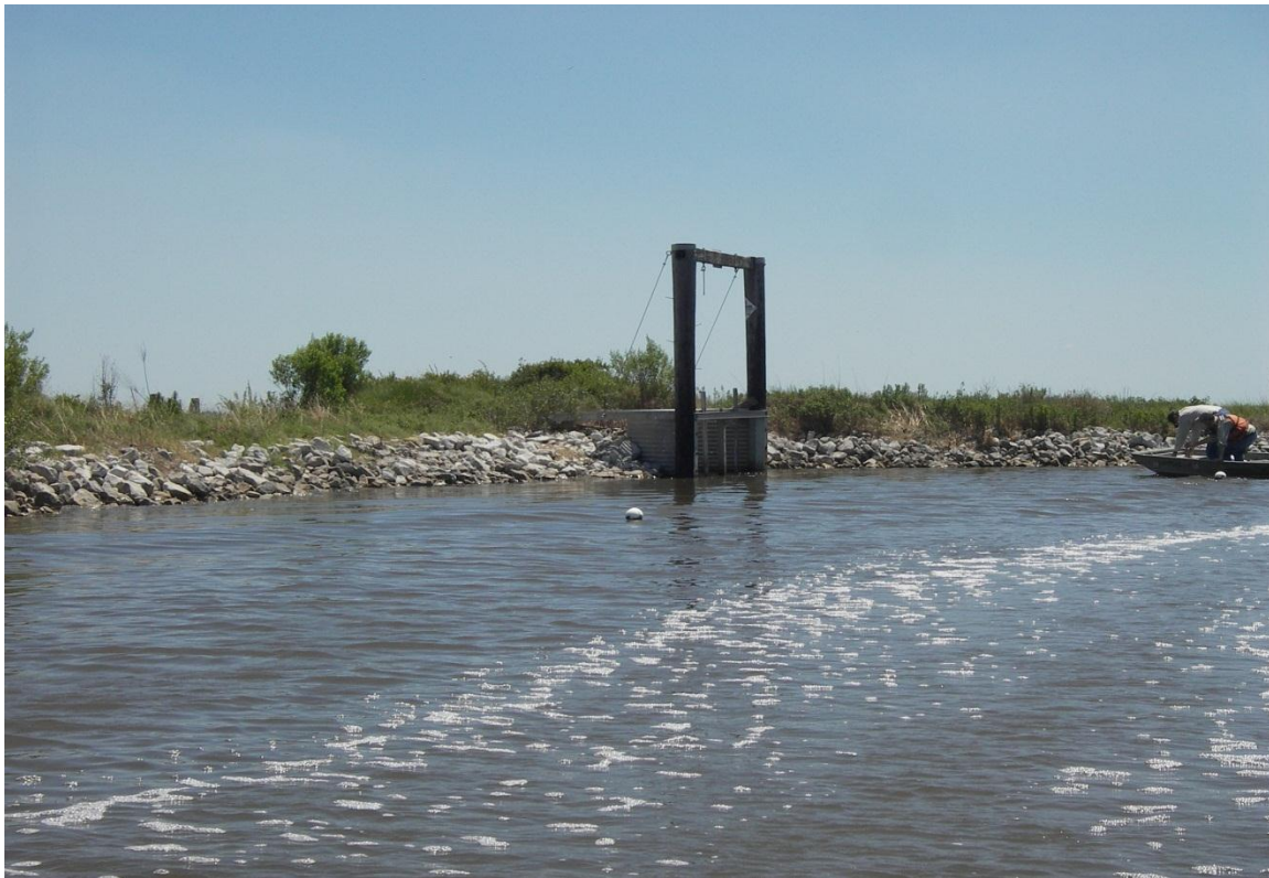
Photo No. 9, Structure No. 5
