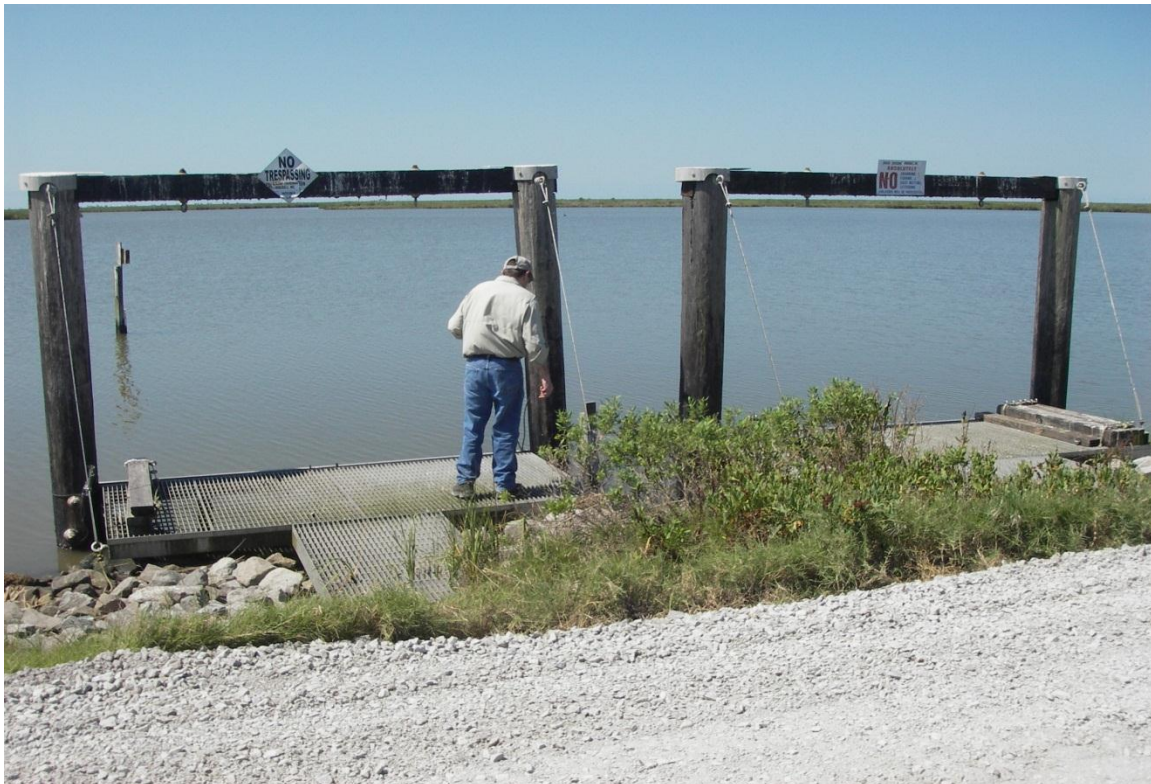
Photo No. 2 Structure No. 7
