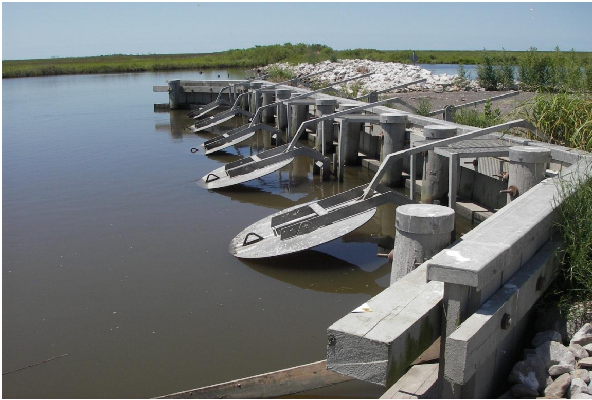
Photo No. 11, flap side, Structure No.4
