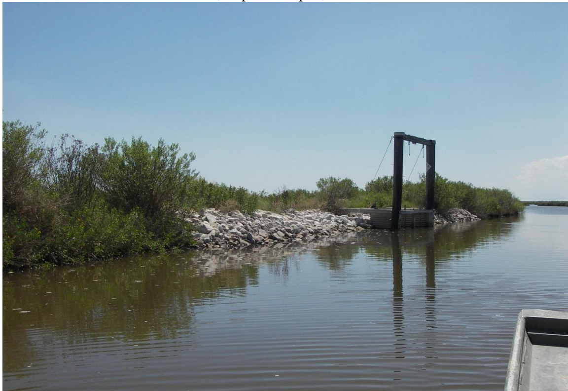
Photo No. 8, Structure No. 11
