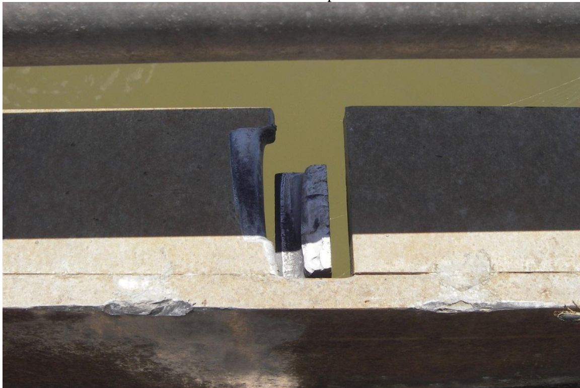
Photo 24 —broken pivot point on Structure 13 flap
