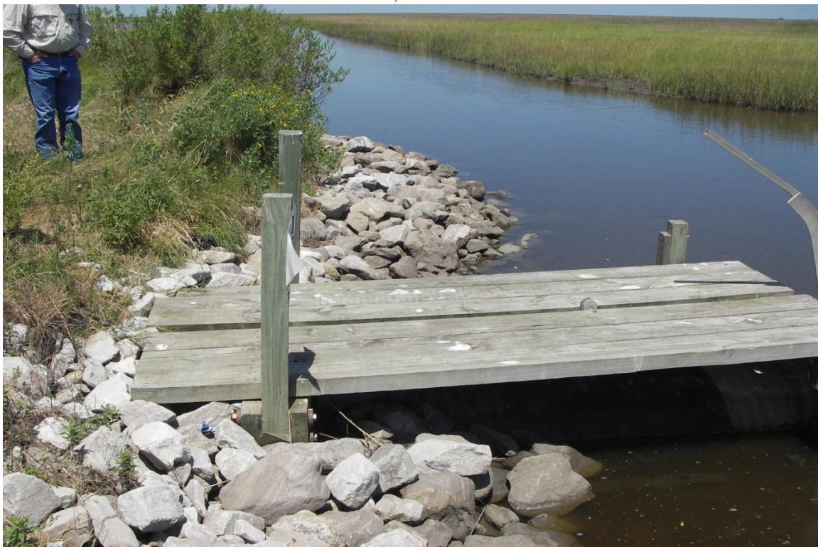
Photo No. 10, flap side, Structure No. 5
