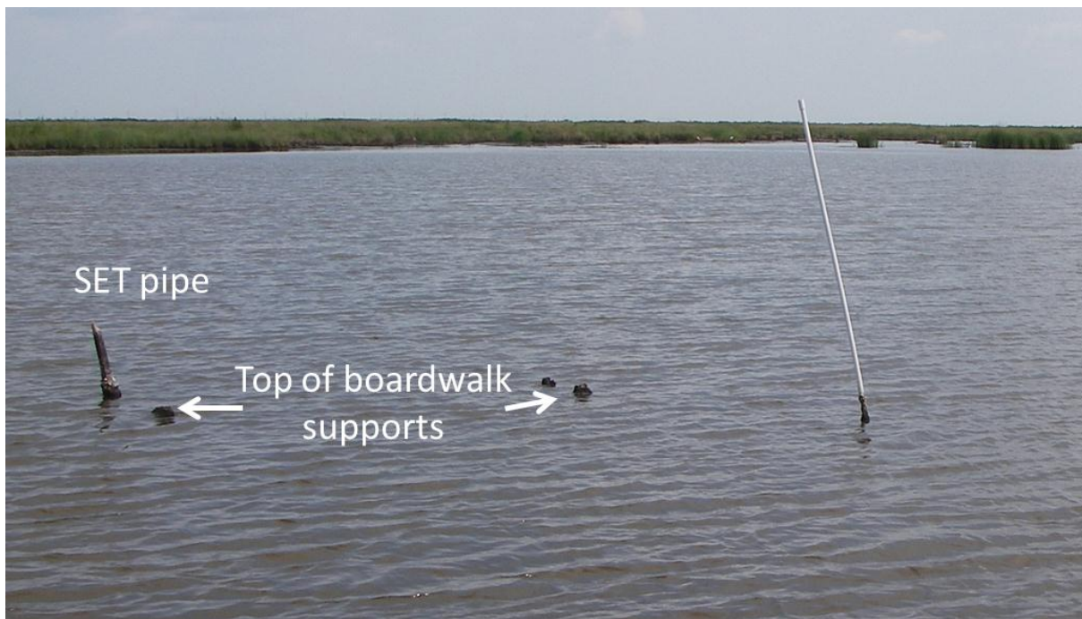
Picture 1. Picture of Station CS20-52R taken in Aug 2009 following Hurricanes Rita (2005) and Ike (2008). Most of the open water was marsh prior to the hurricane storm-surge scour (see figure 5B for extent of damage in Reference Area 1).
