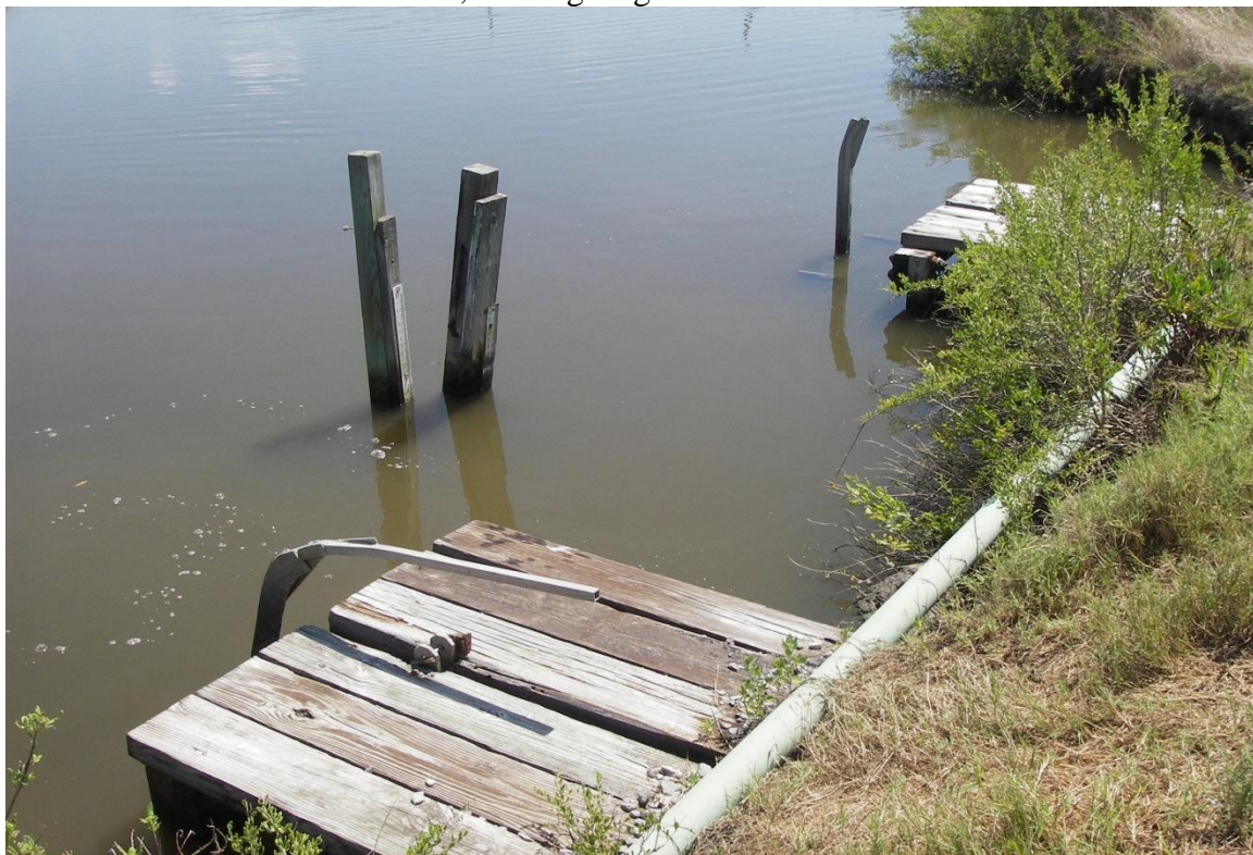
Photo No. 6, flapgates on Structures 9a & 9b
