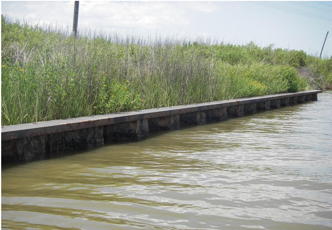
Photo 22 —sheet pile wall and cap at Structure 13
