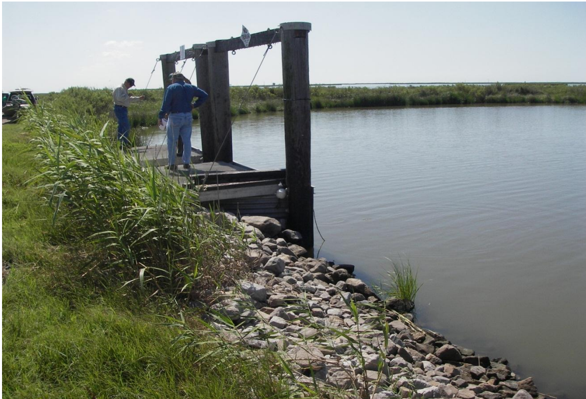
Photo No.1 Structure No. 6
