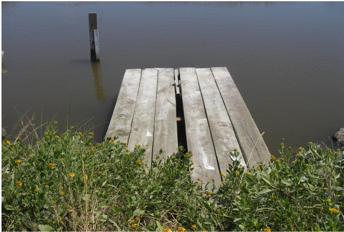
Photo No. 7, flap stuck open, Structure No. 11
