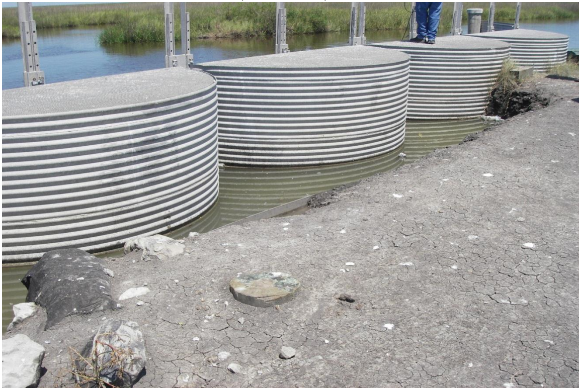
Photo 14 , sinkholes developing behind Structure 4 stoplog bays
