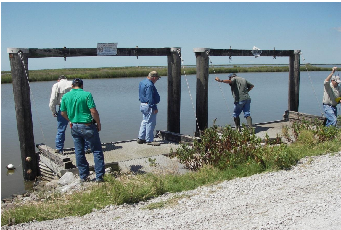
Photo No. 3, Structure No. 8
