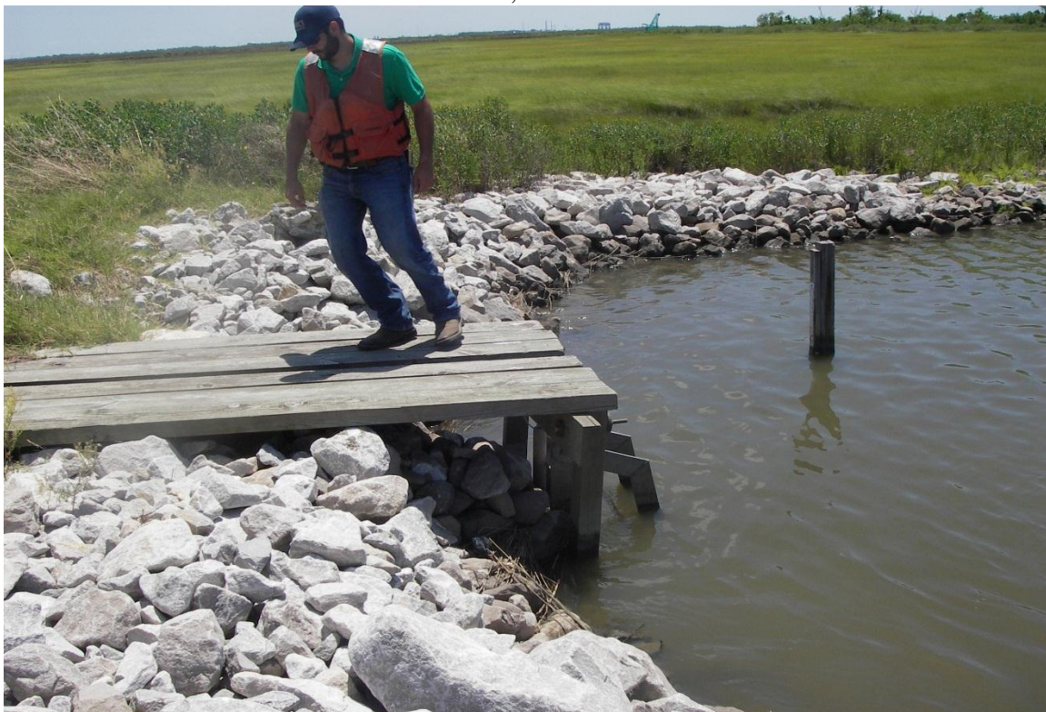
Photo 16, flap side, Structure 3
