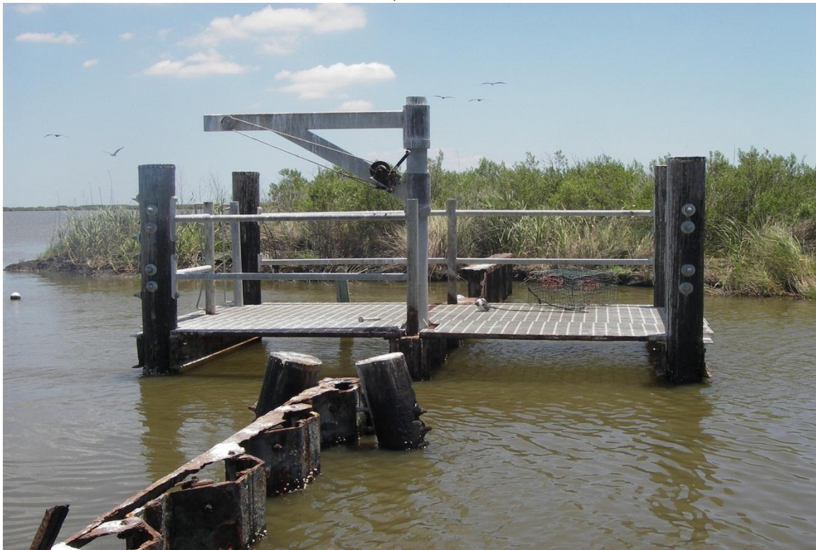
Photo 20, sheet pile, cap and lifting hardware at Structure 17
