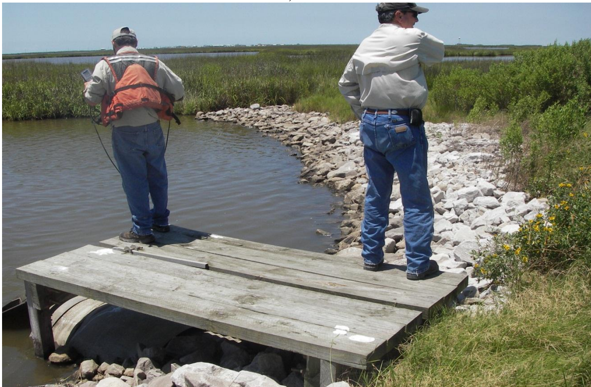
Photo 18, flap side, Structure 1
