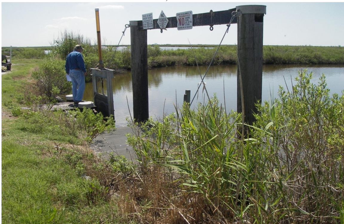
Photo No. 4, Structure No. 9a
