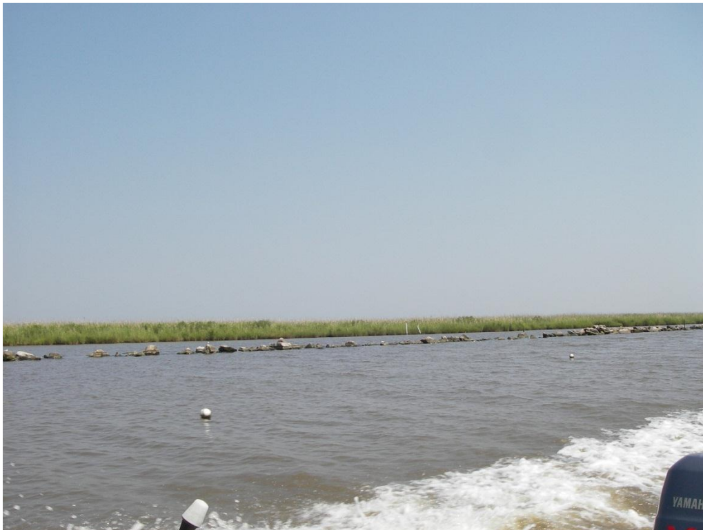
Photo No. 6, Low Areas in Rock Dike
