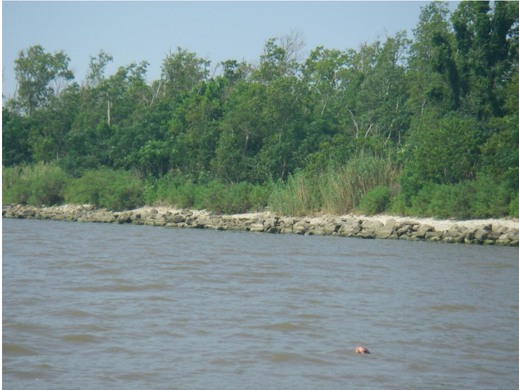
Photo No. 1, Typical Rock Dike
