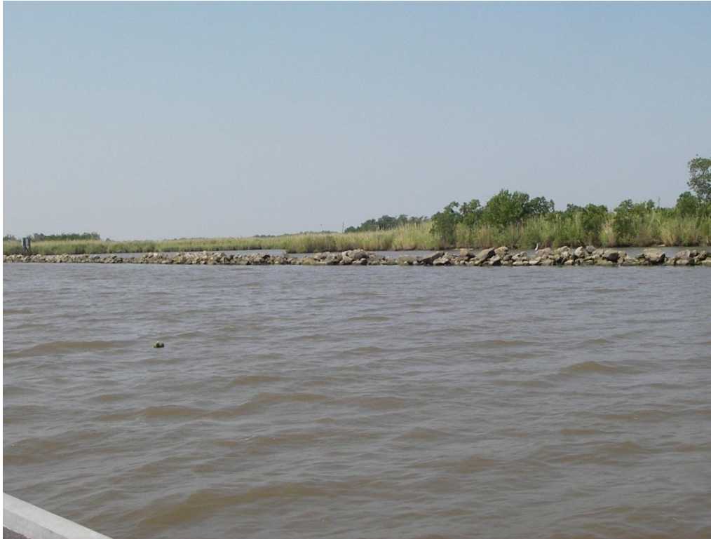
Photo No. 3, Typical Rock Dike
