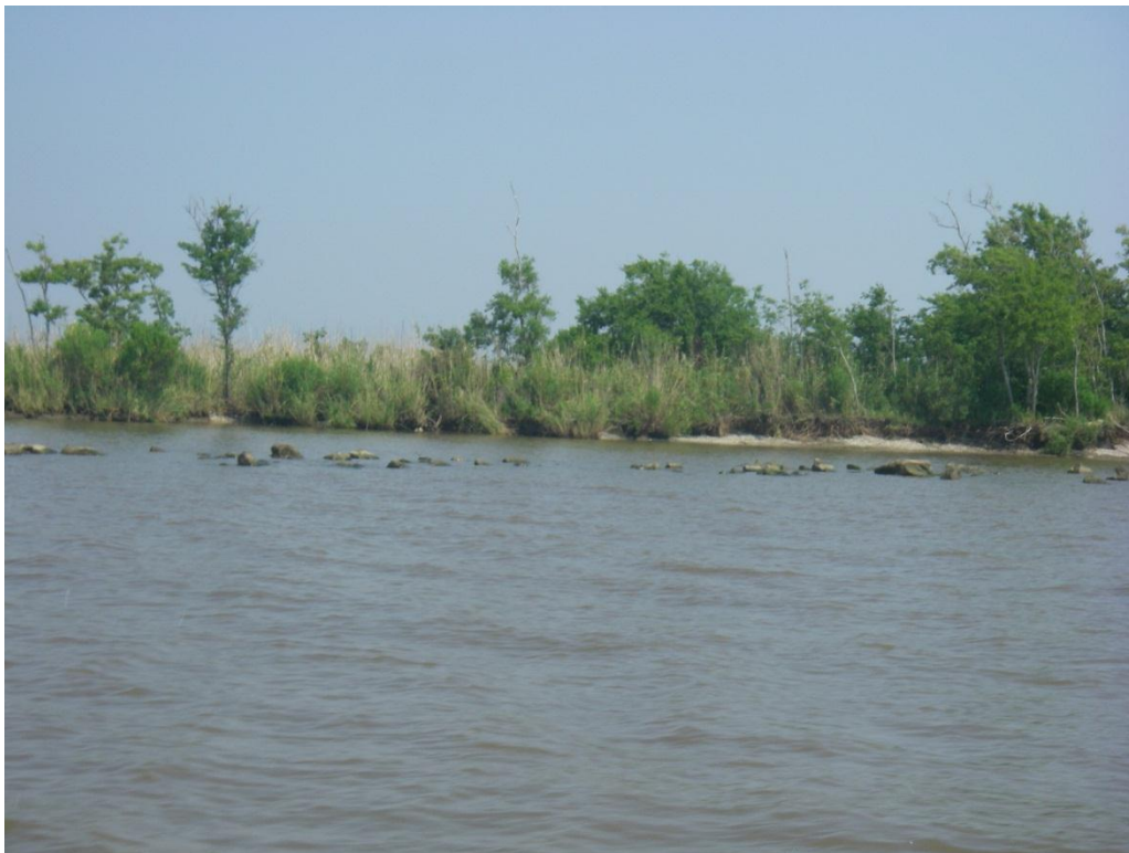
Photo No. 4, Low Areas in Rock Dike, Erosion of Bank
