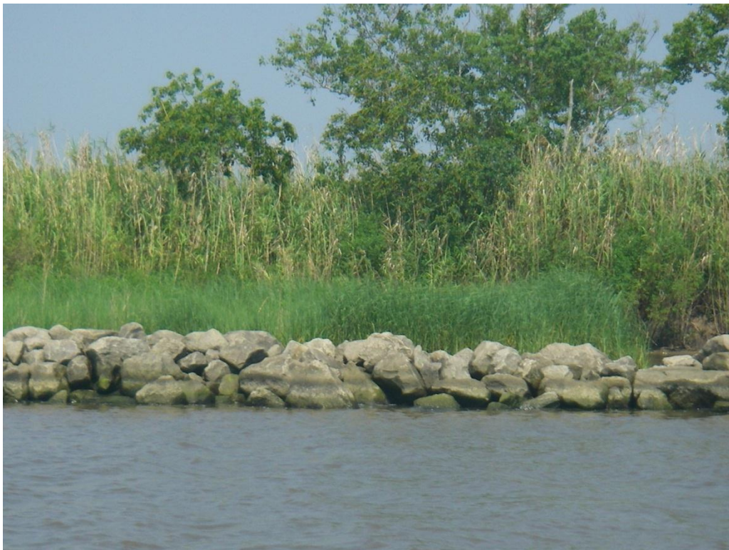
Photo No. 2, Vegetation Behind Rock Dike
