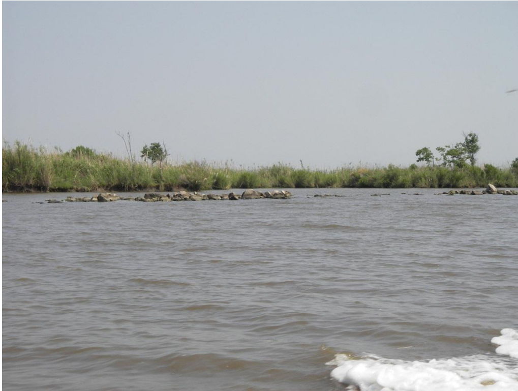
Photo No. 5, Low Areas in Rock Dike
