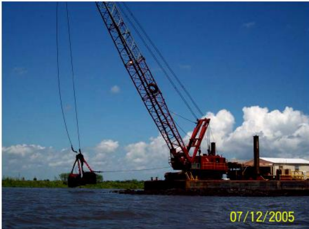
Figure 4 – Dredge utilized in the Barataria Basin Landbridge Shoreline Protection CWPPRA project (BA-27d, CU#6).
