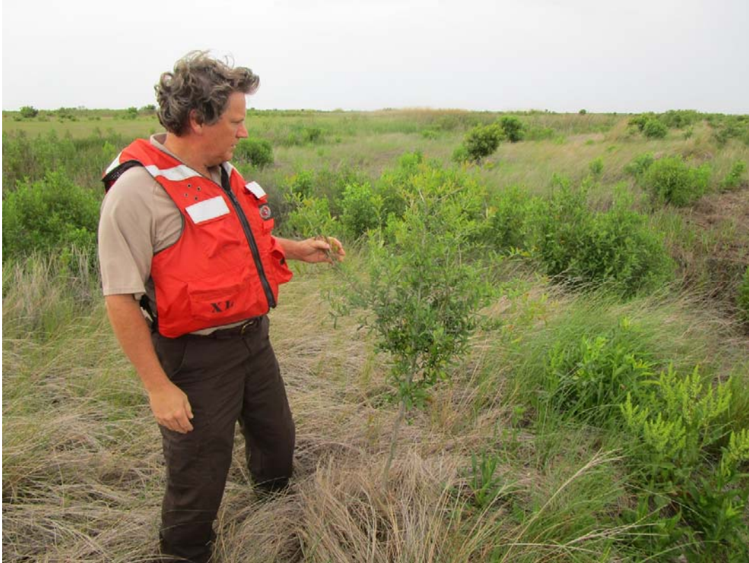
Area C – Oak tree growing on northern containment berm
