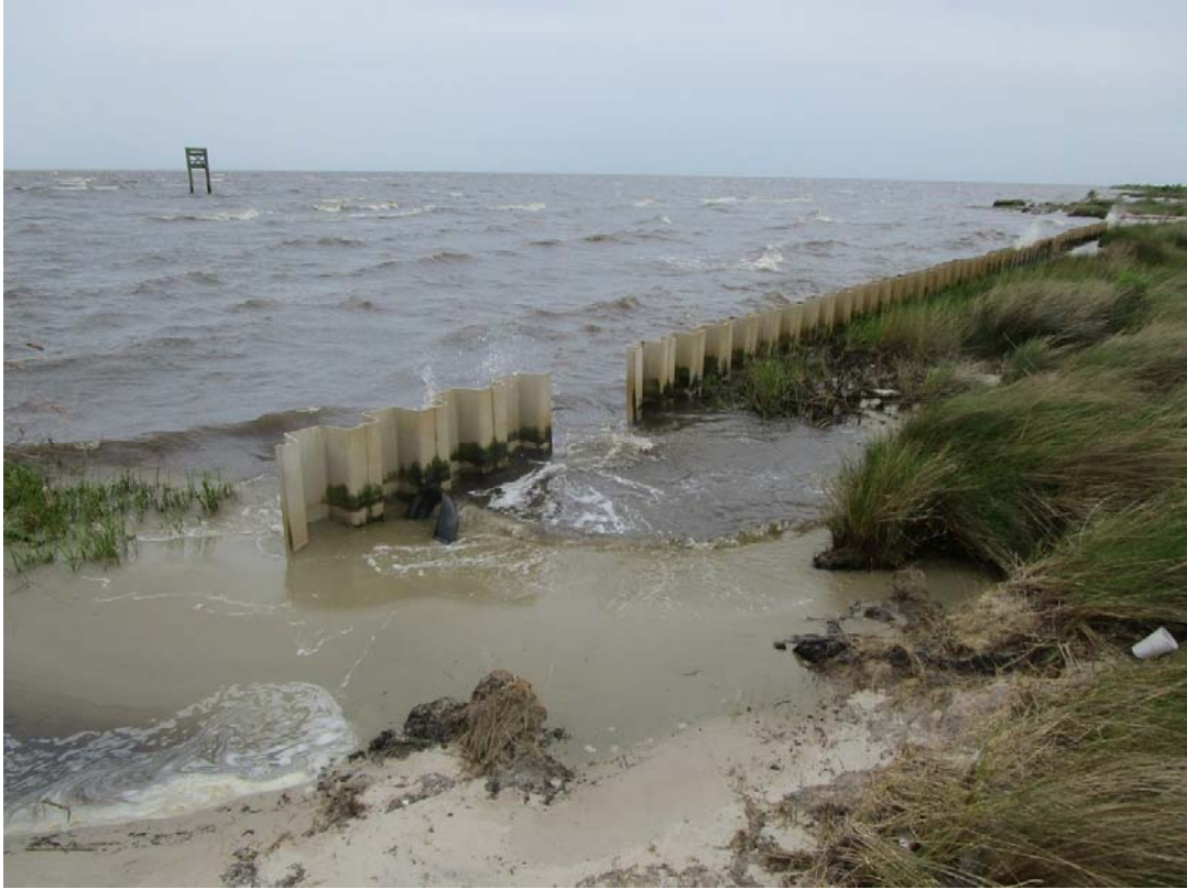
Area D –Vinyl sheet pile wall at Lake Pontchartrain shoreline
