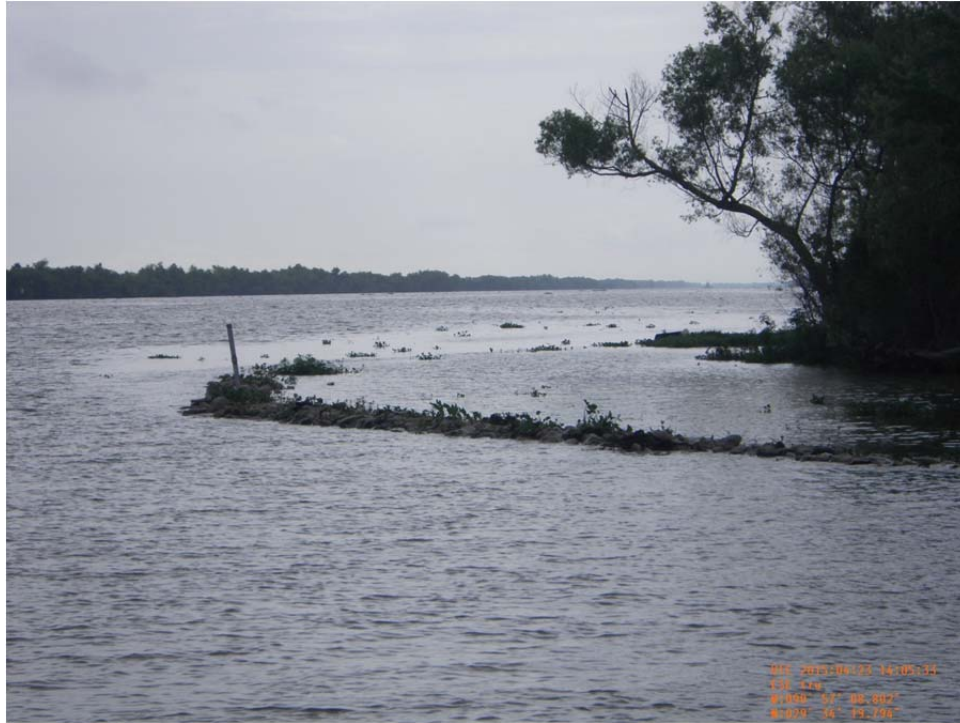
Photo 5: View of rock dike near Sta. 2+00 looking eastward.
