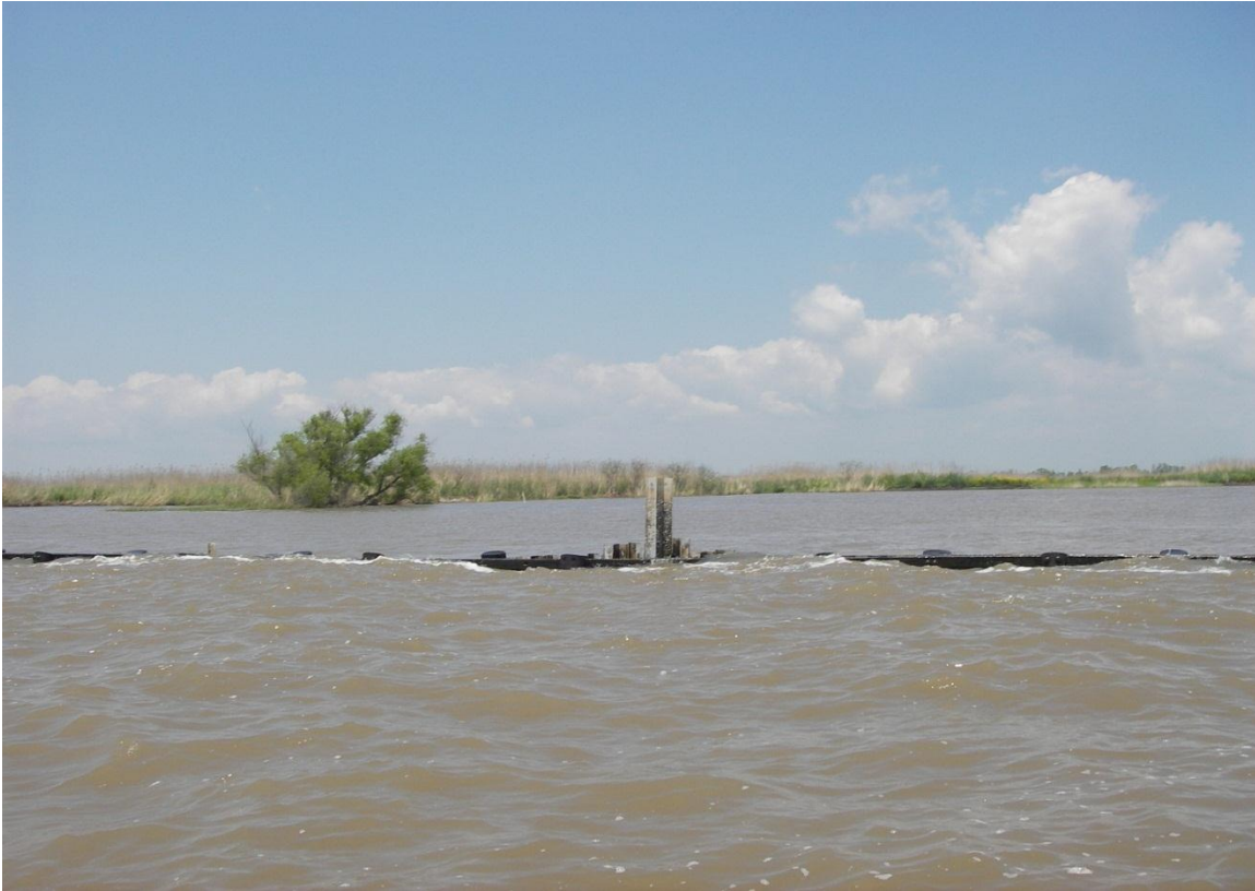
Photo 16 —rising sheet pile on PVC wall
