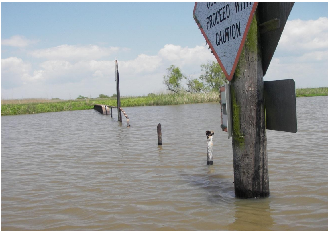
Photo 3 —damaged rail on Bayou Long structure
