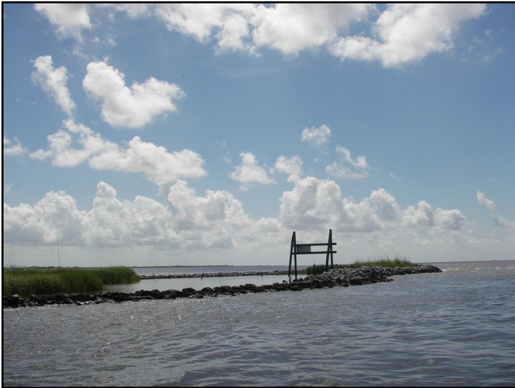
Photo No. 4, Rock dike at Oaks Canal, East side
