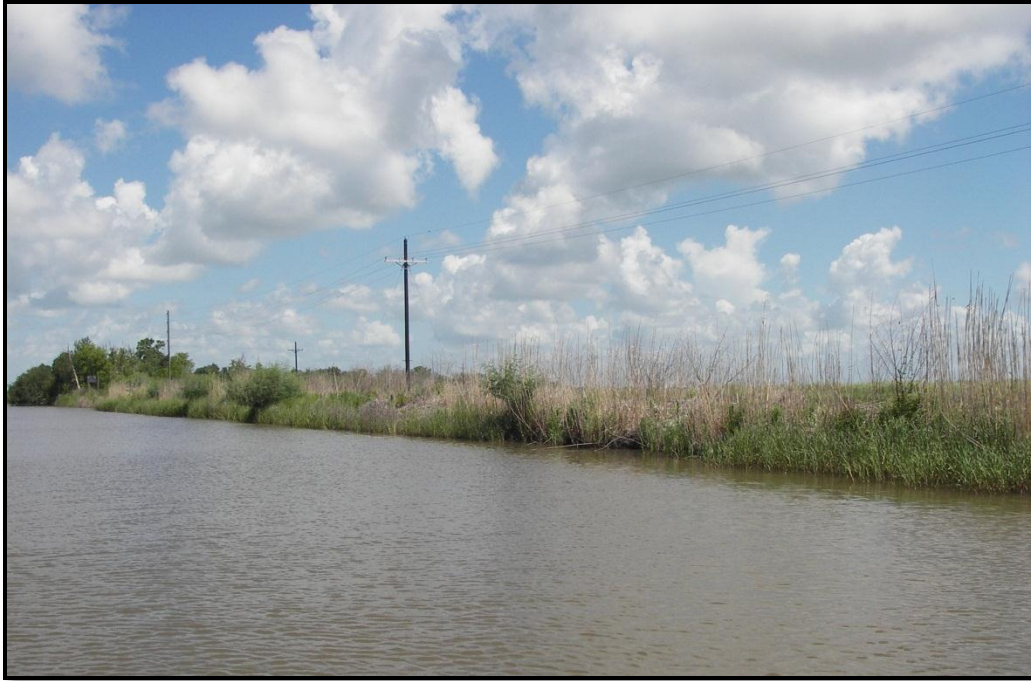
Photo No. 9 , Spoilbank Maintenance along Oaks Canal
