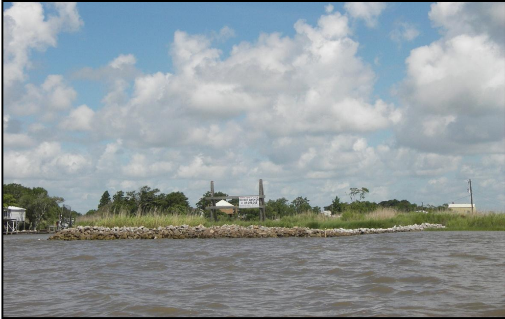
Photo No. 5 , Rock dike at Oaks Canal, East side
