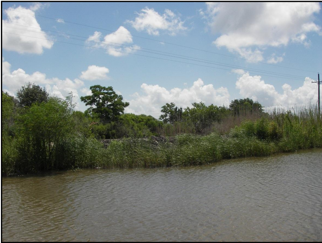
Photo No. 10 , Earthen Canal Plug on Oaks Canal
