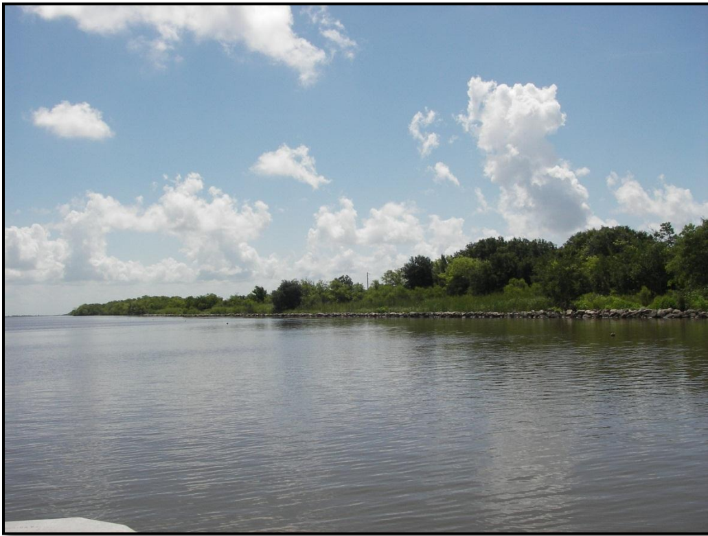
Photo No. 8, Rock dike along south bank of GIWW
