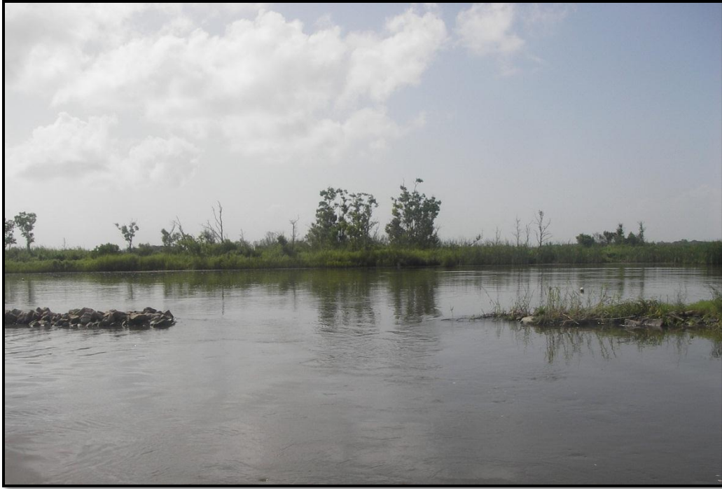
Photo No. 7, Rock plug gapped as part of maintenance event. (photo taken 07/02/2012)
