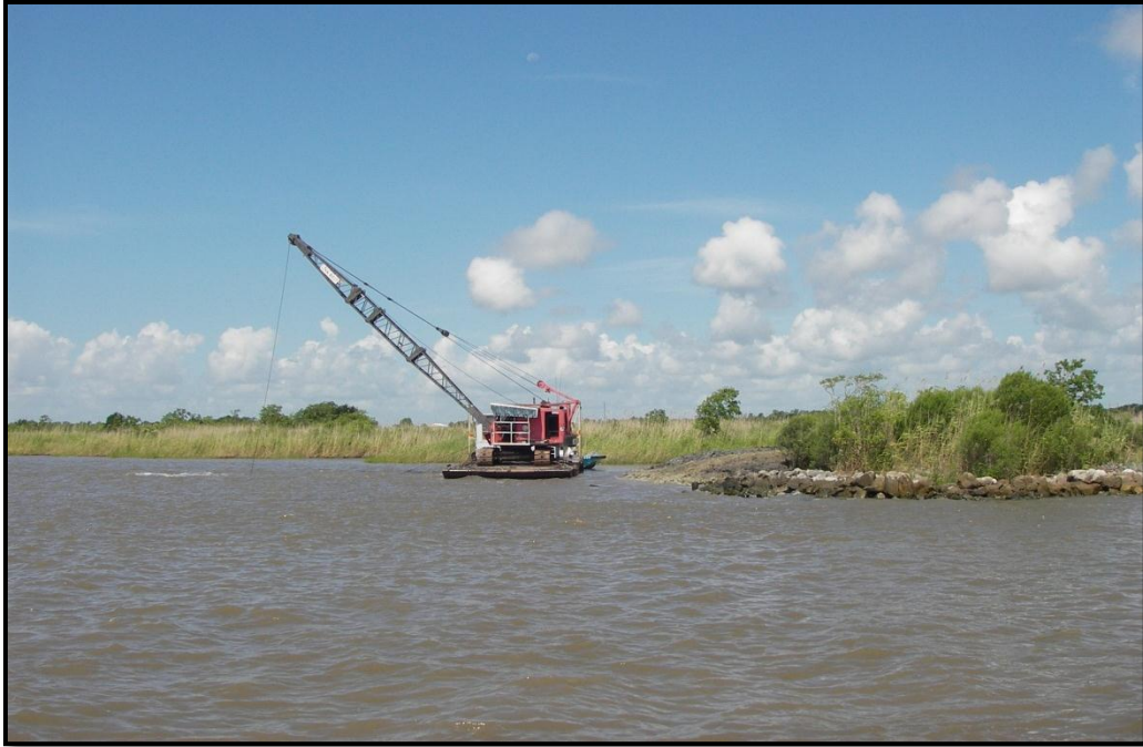
Photo No. 3, Rock dike at Oaks Canal, west side
