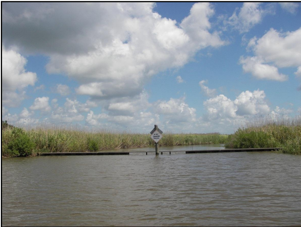
Photo No. 6 , Cow Path Structure
