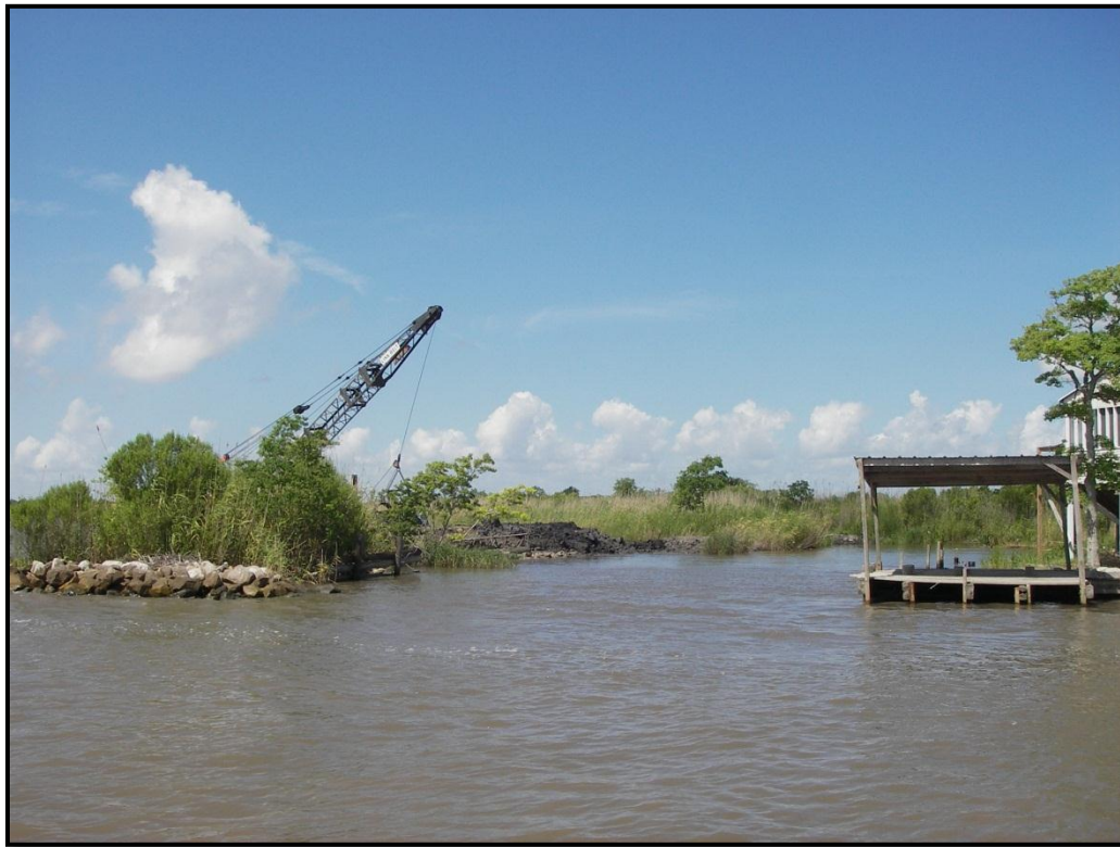
Photo No. 2, Rock dike at Oaks Canal, west side
