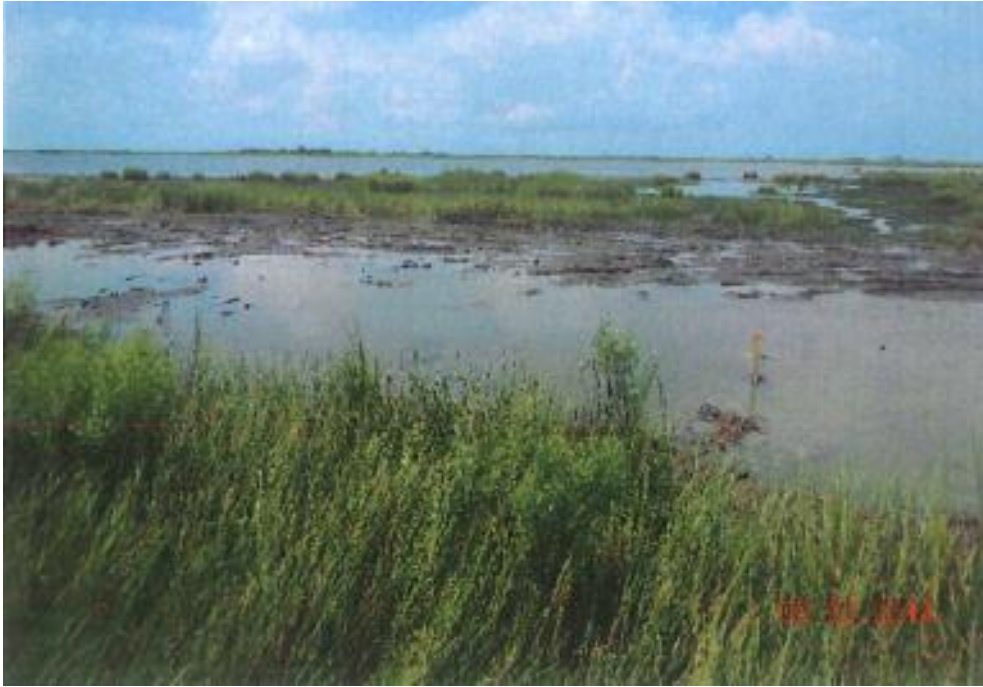
Photo No. 6, Containment Dike Excavation at Timber Mat location (Looking West towards Hawkins Lake)
