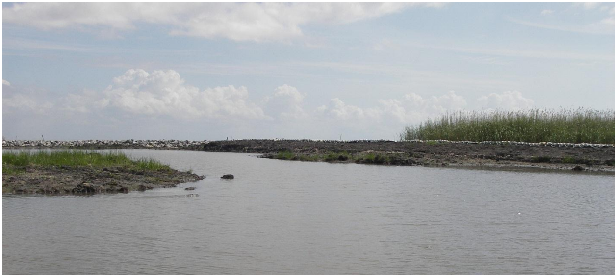
Photo No. 9, Shoreline Protection, Articulated Concrete Mats on Gulfward Shoreline/ MC Cell No. 1
