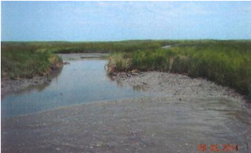
Photo No. 7, Nourished Area No. 2 at Eastern Plug No. 2 removal
