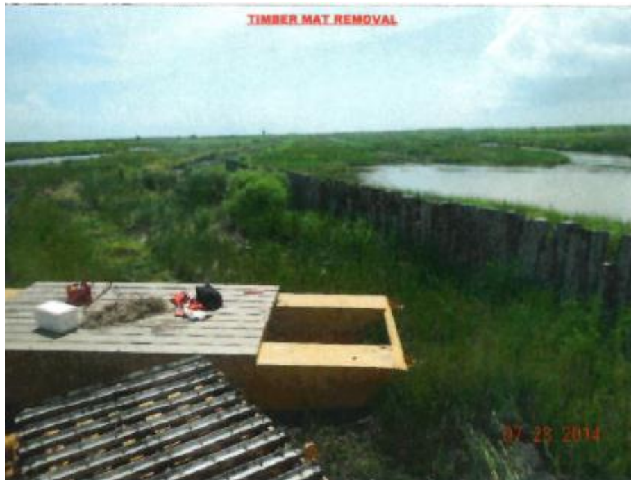
Photo No. 5, Marsh Creation Cell No. 2 & Nourishment Area No.3, Containment Dike at Timber Mat location (Prior to Removal - Looking East)
