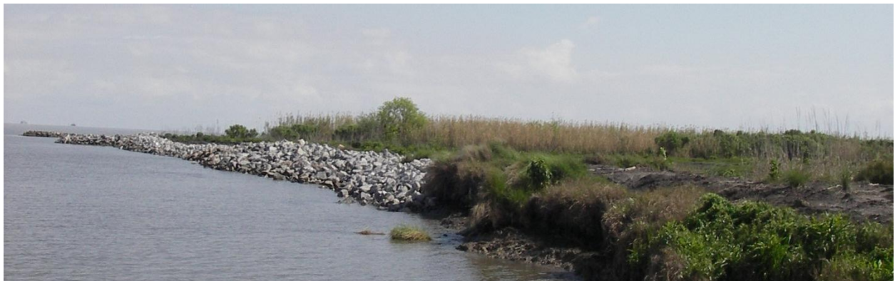
Photo No.2, TV-14 Rock Plug replacement - West end of the E-W Canal at Intersection of N-S Canal
