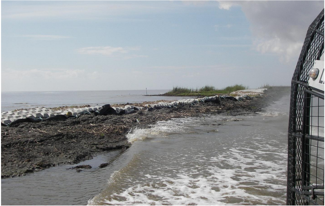
Photo No. 8, Shoreline Protection, Articulated Concrete Mats on Gulfward Shoreline/ MC Cell No. 1
