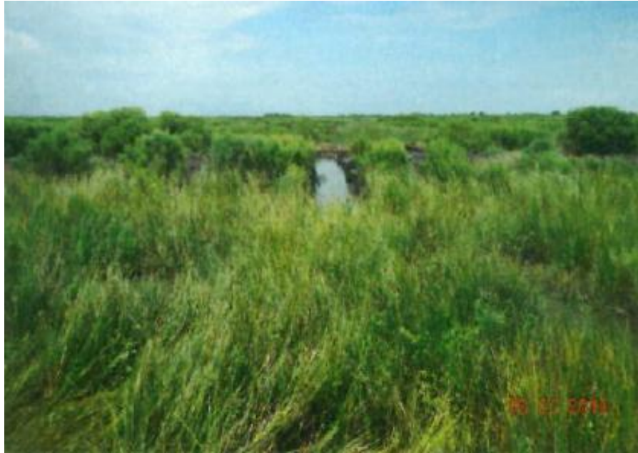
Photo No. 4, Gap N- Marsh Creation Cell No.2 & Nourishment Area No. 3 (Looking North)
