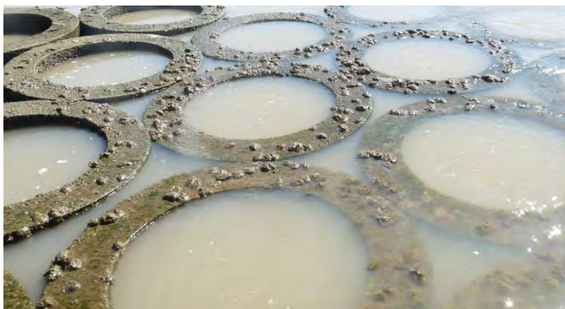
Figure 16. Colonization of oysters on east end of Oysterbreak-East 20 months (1.7 years) after construction.
