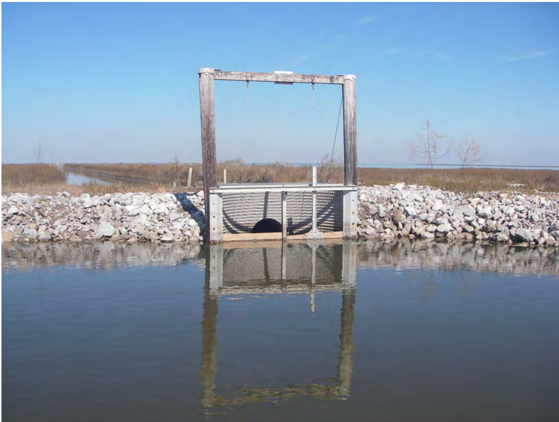
Figure 10. Structure No. 5 in the northwest corner of CTU 2 provides managed hydrologic connectivity between the East Mud Lake Marsh Management (CS-20) project area and Calcasieu Lake (background), which is connected to the higher salinities and water-level fluctuations of the Gulf of Mexico via the Calcasieu Ship Channel. This view is looking at the interior “marsh side” stop log header that controls water levels within the managed area.
