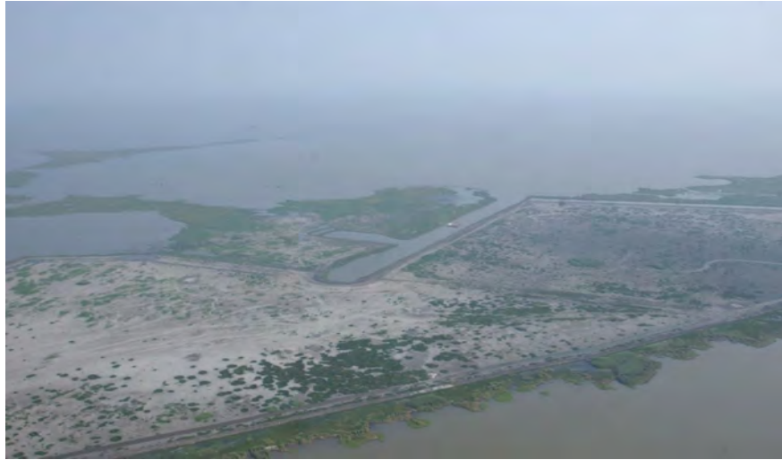
Figure 18. Aerial view of the eastern half of the East Marsh Island Marsh Creation (TV-21) project, June 2011. The areas in the foreground are the containment area portions of the project in which dredged material was contained by earthen retention dikes.
