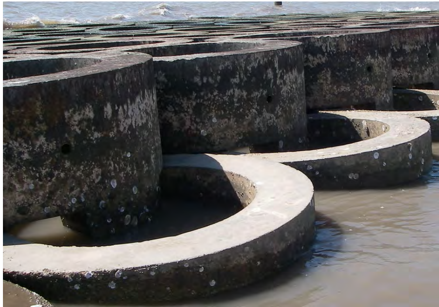
Figure 14. A , Oblique aerial photograph taken during low water about a year after construction of the Oysterbreak reefs at the Bioengineered Oyster Reef Demonstration (LA-08) project. Note the elevation difference (based on water inundation) between Oysterbreak–West composed of OysterKrete (lower) and Oysterbreak–East composed of standard weight concrete (taller). Also, note the new land that formed behind Oysterbreak–East after construction. B , Stacked, interlocking rings shown from behind Oysterbreak–East; note the waves crashing on the front of the reef and the calm water behind the reef.
