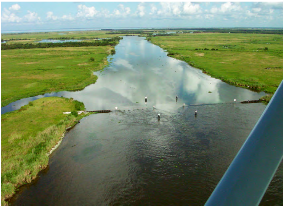
Figure 4. Low-level weir with boat bay (80 feet wide and 8 feet deep) at opening of Humble Canal (400 feet wide and 20 feet deep) reduces water exchange between East Cote Blanche Bay (West Cote Blanche Bay is in the background) and marshes between the Cote Blanche Bays. Note the wide and straight access canal.
