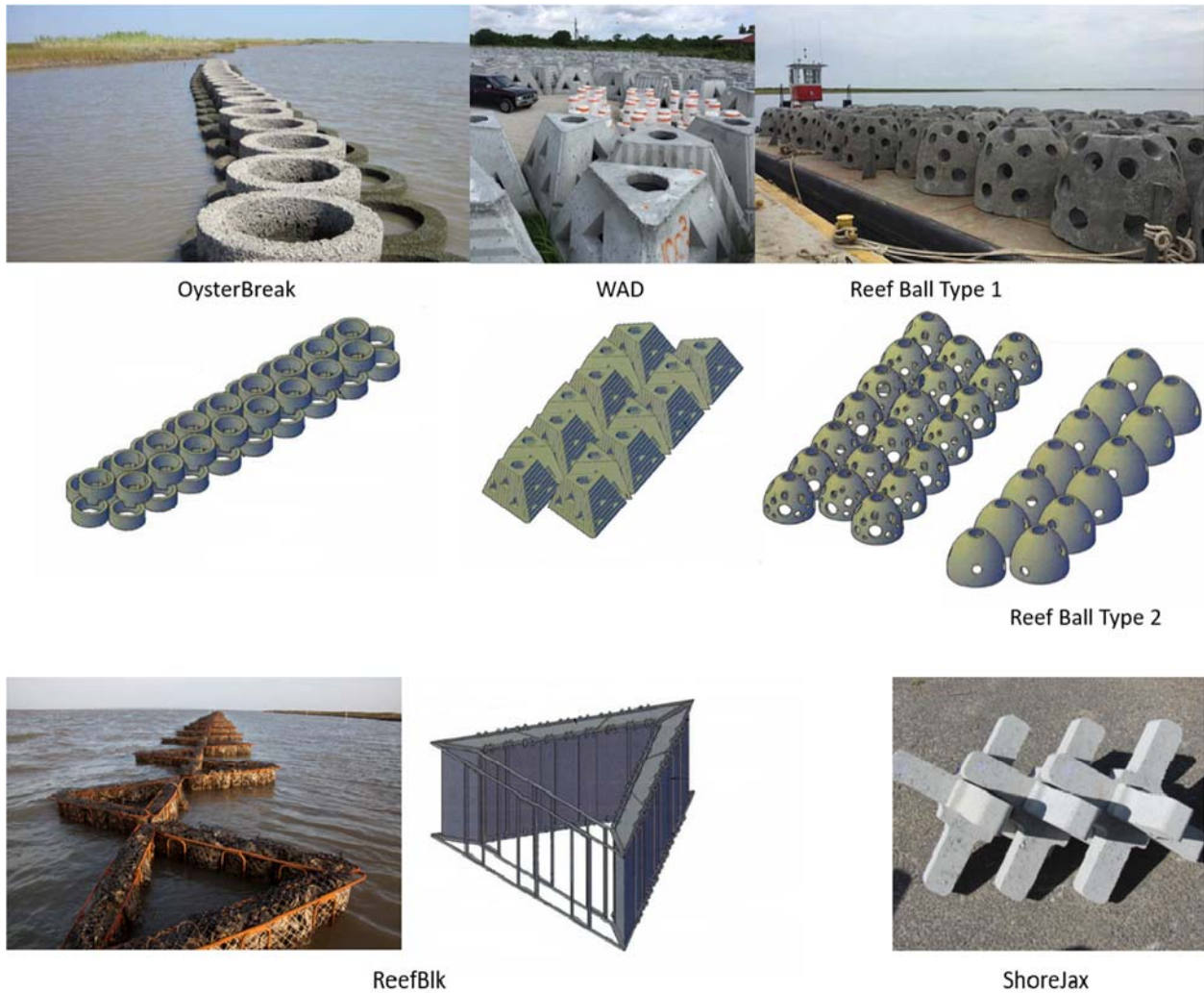
Figure 1.4: PO-148 shoreline protection structures (photo credits: OysterBreak – Wayfarer Environmental Technologies; WAD - Mott MacDonald; Reef Ball - Tetra Tech, Inc.; ReefBlk - Beth Maynor Young, 2010; ShoreJax - ACF Environmental. Sketches: Coast and Harbor Engineering, 2015).
