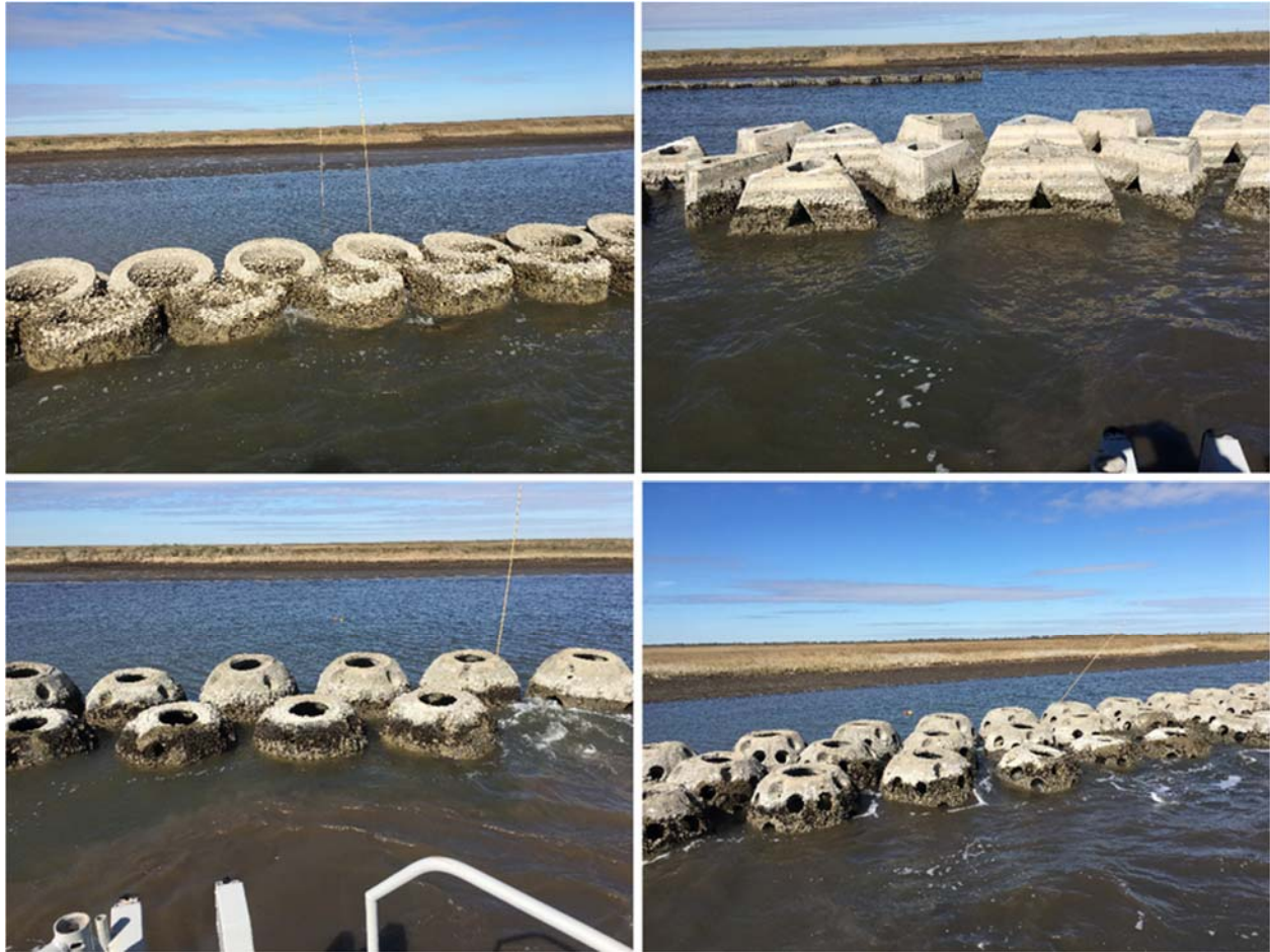
Figure 4.3: OysterBreak (top left), WAD (top right), Reef Ball Type 2 (bottom left), Reef Ball Type 1 (bottom right). Photos taken 15 January 2018.
