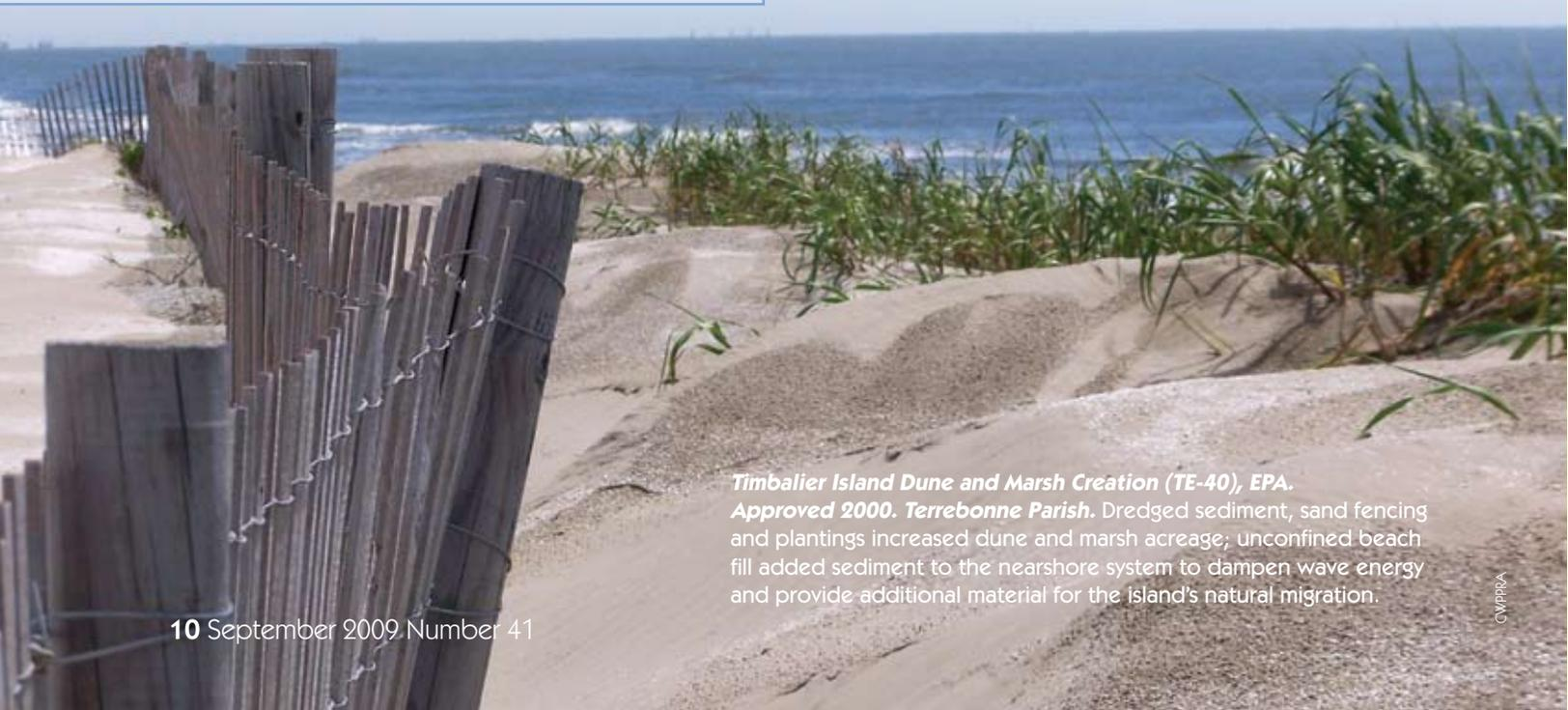
**Timbalier Island Dune and Marsh Creation (TE-40), EPA. Approved 2000. Terrebonne Parish.** Dredged sediment, sand fencing and plantings increased dune and marsh acreage; unconfined beach fill added sediment to the nearshore system to dampen wave energy and provide additional material for the island's natural migration.
