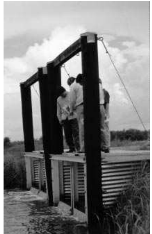
Dedication ceremony guests examine one of the double flap gates installed at the Mud Lake Project. (NRCS photo)
