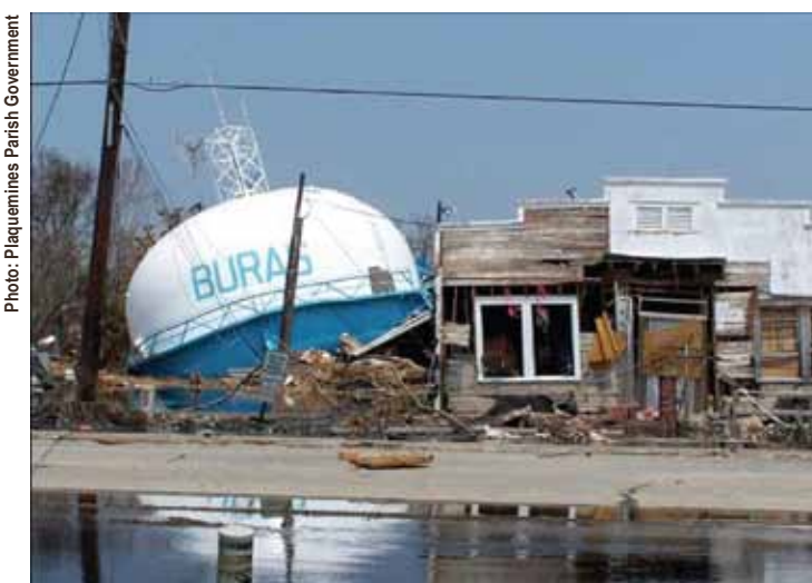
Storm surge from Hurricane Katrina (August 29, 2005) devastated the town of Buras, Louisiana. The Buras water tower was completely destroyed.
