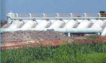
Box culvert control gates
