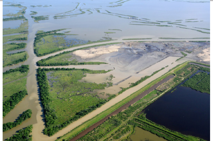
Construction of the Lake Hermitage Marsh Creation (BA-42) project with Grand Bayou on the left and the site of Grand Bayou Ridge and Marsh Restoration - Increment 2 (BA-257).
