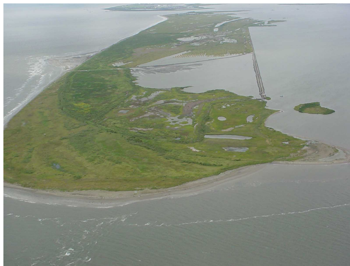
Approximately 40 acres of dune were created by this project that provided added protection to Grand Terre and helped contain the U.S. Army Corps of Engineers' beneficial use of dredged sediment site. Both projects have significantly added to the longevity of this barrier island.
