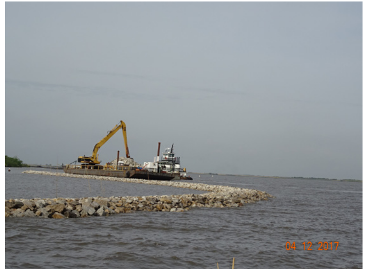
Construction of the project's stone breakwater.
