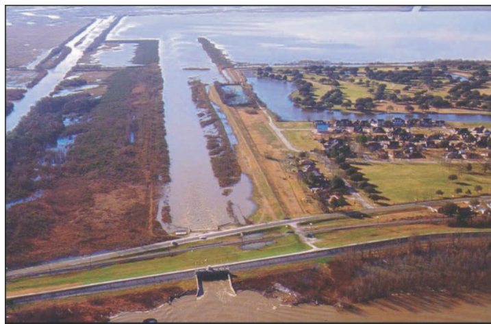
The Caernarvon diversion structure: a potential location of the sediment enrichment demonstration.
