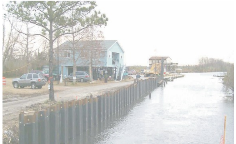
Steel sheet-pile will ensure that erosion will not enlarge this cross-sectional area of the channel. Actions such as these will restore a more natural hydrologic regime to the area.
