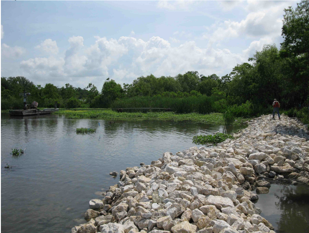
Photo #3 – New Rock to Structure #16 (under vegetation)
