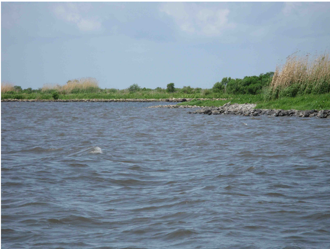
Photo #4 – Low spot near Structure #20
