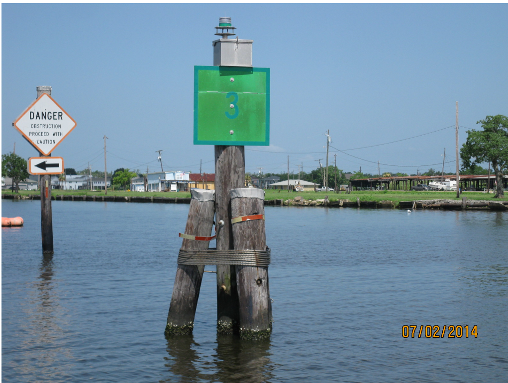
Photo #2 – Goose Bayou Pile Cluster
