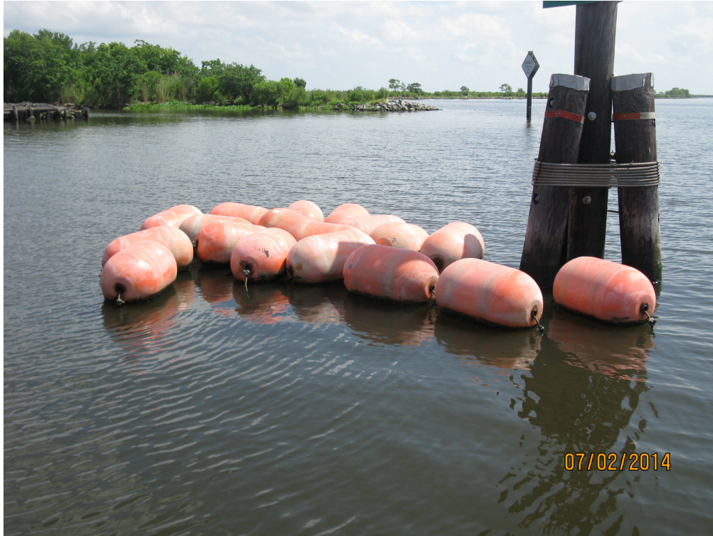
Photo #3 – Buoy Damage at Goose Bayou (North Side)
