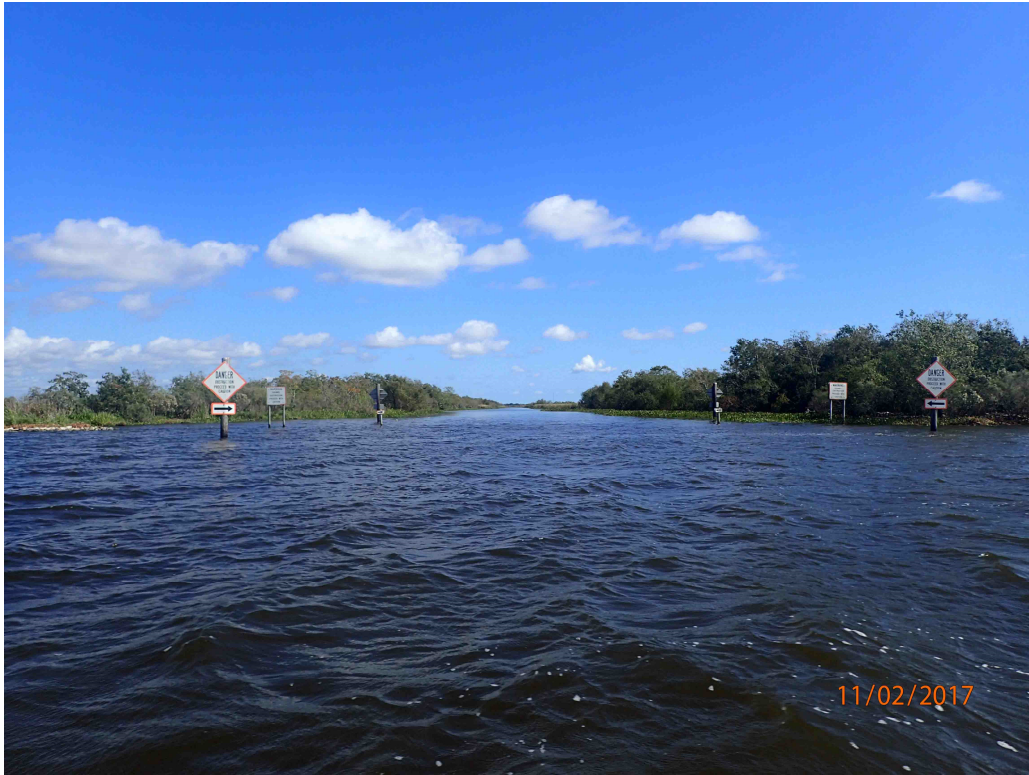
Photo #7 – Damaged Signs at Structure #19
