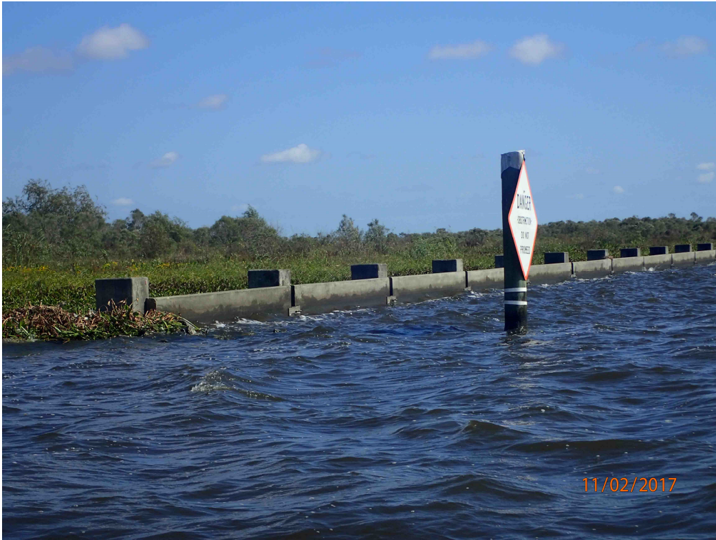
Photo #9 – Panel Wall Shoreline Protection (CU4)
