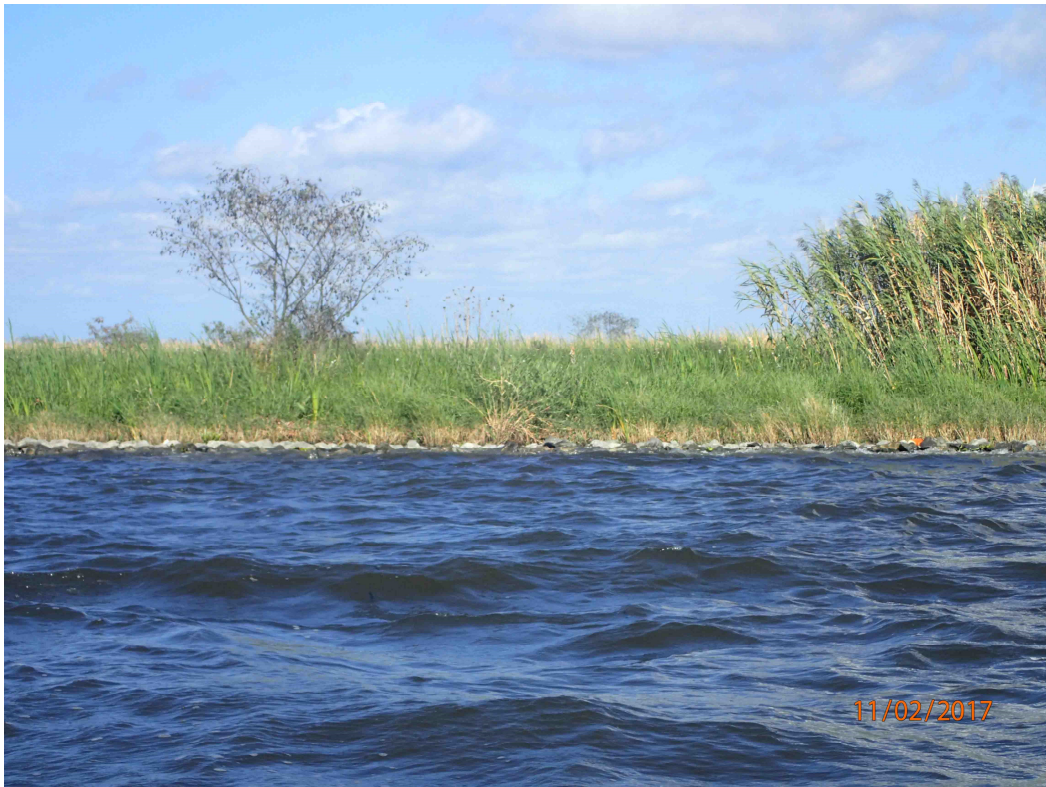
Photo #10 – Bayou Rigolettes Shoreline Protection (CU2)
