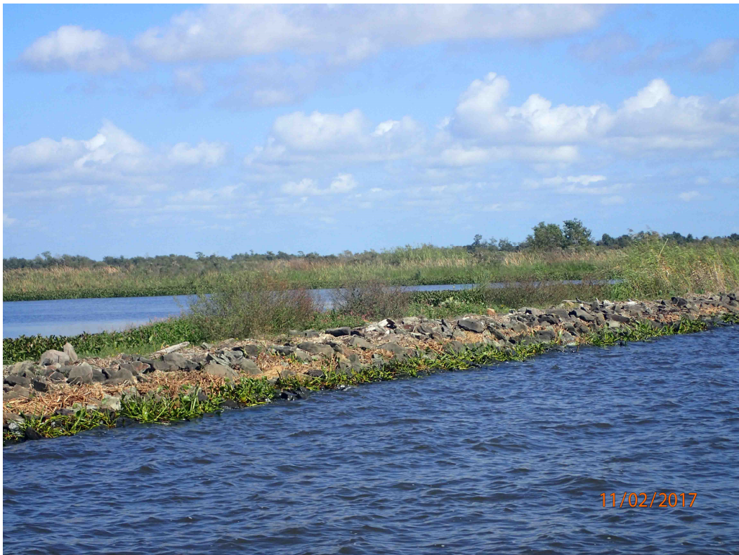
Photo #1 – Bayou Perot Shoreline Protection (CU3)
