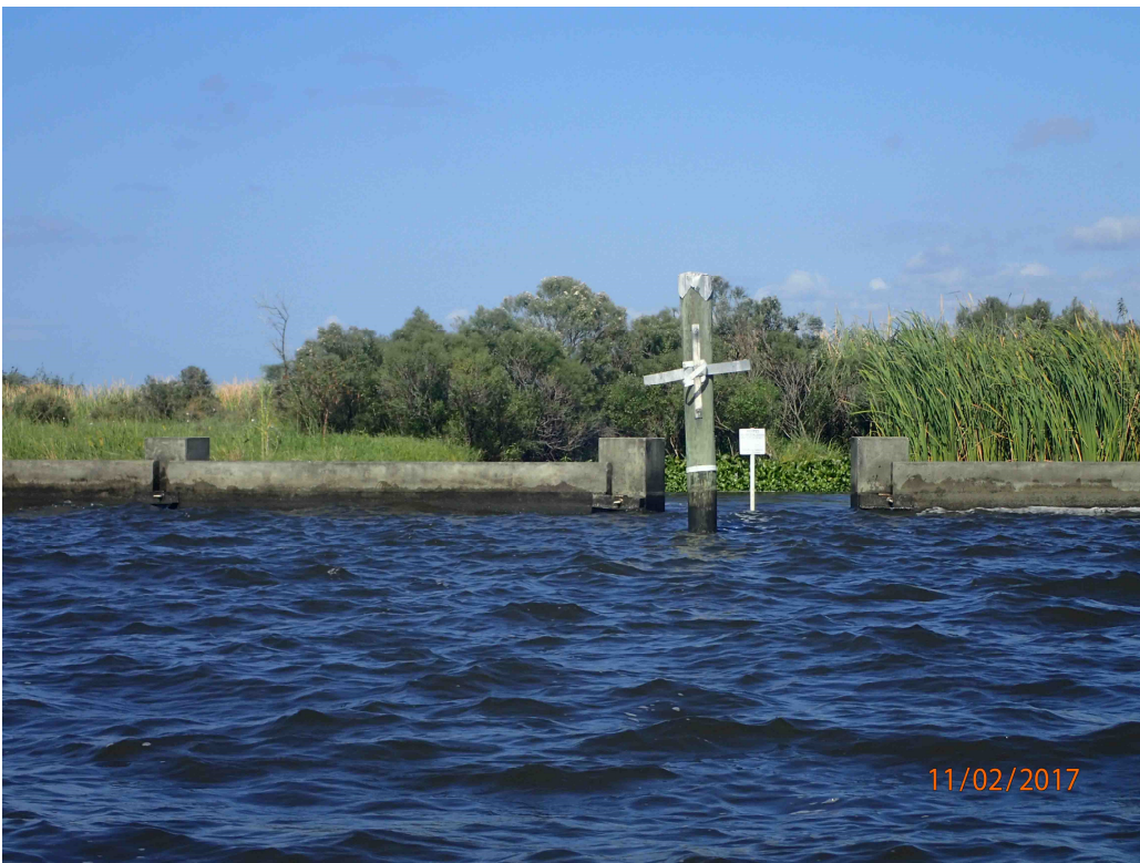
Photo #8 – Missing Sign (CU4)
