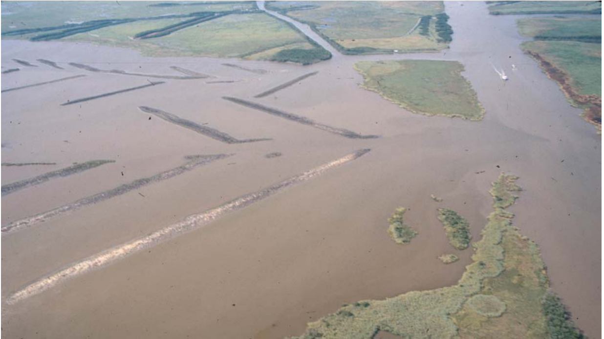
Figure 8. Aerial photo 9/30/99 immediately post construction. Freshwater Bayou is to the right.
