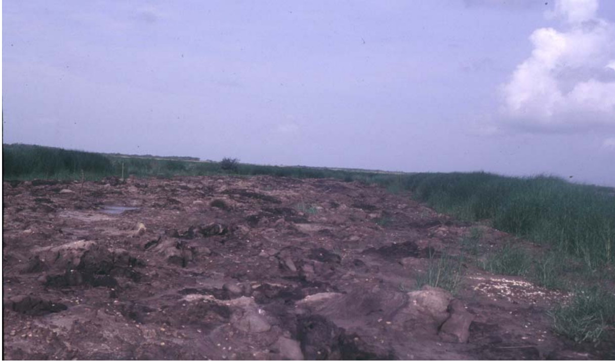
Figure 10. View from middle of a terrace in June 2000 one year after construction and planting, showing growth of planted Spartina alterniflora on either side.
