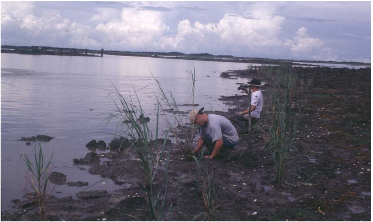
Figure 9. Newly constructed terrace being planted in summer 1999.
