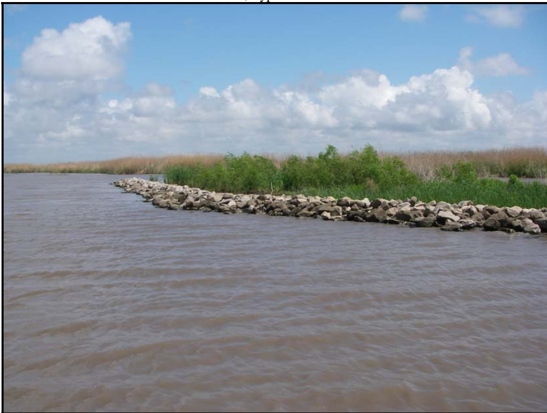
Photo 2, Rock foreshore dike.
