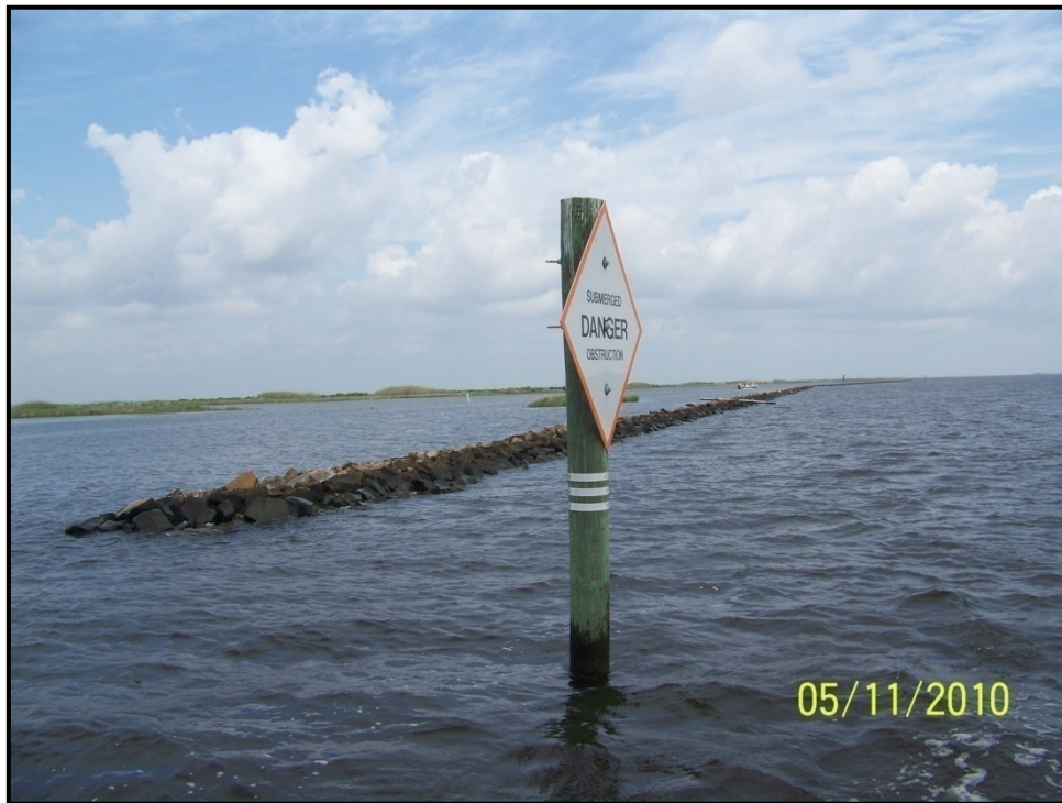
Photo 12 - Rock Segment 12. Tide Reading ~ 1.7 ft NAVD88.
