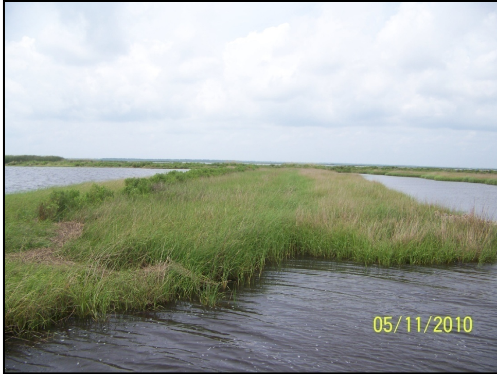
Photo 27 - Marsh creation area SW corner looking west along south dike. Tide Reading ~ 1.7 ft NAVD88.
