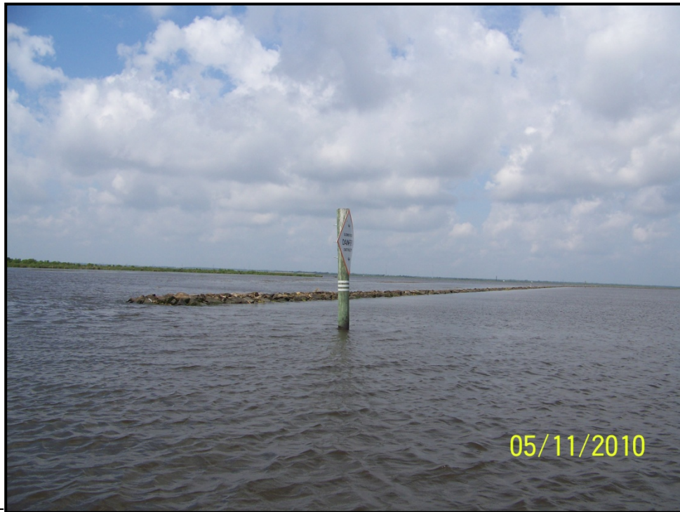
Photo 3 - Rock Segment 3. Tide Reading ~ 1.7 ft NAVD88.
