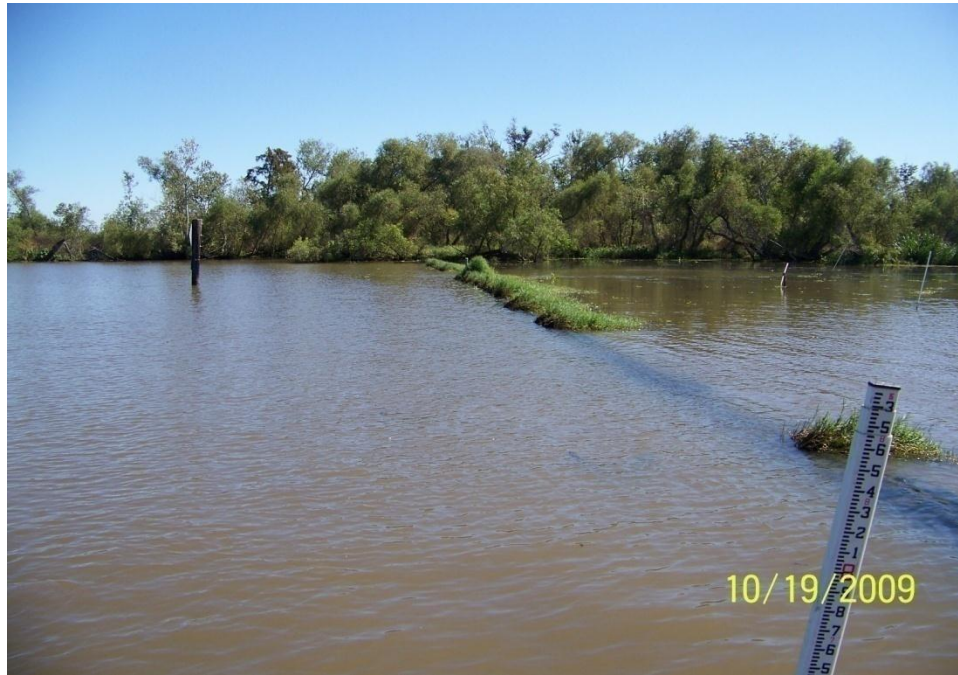
Photo No. 56 – Site R2 – view of settled areas along the elevated shoreline system.
