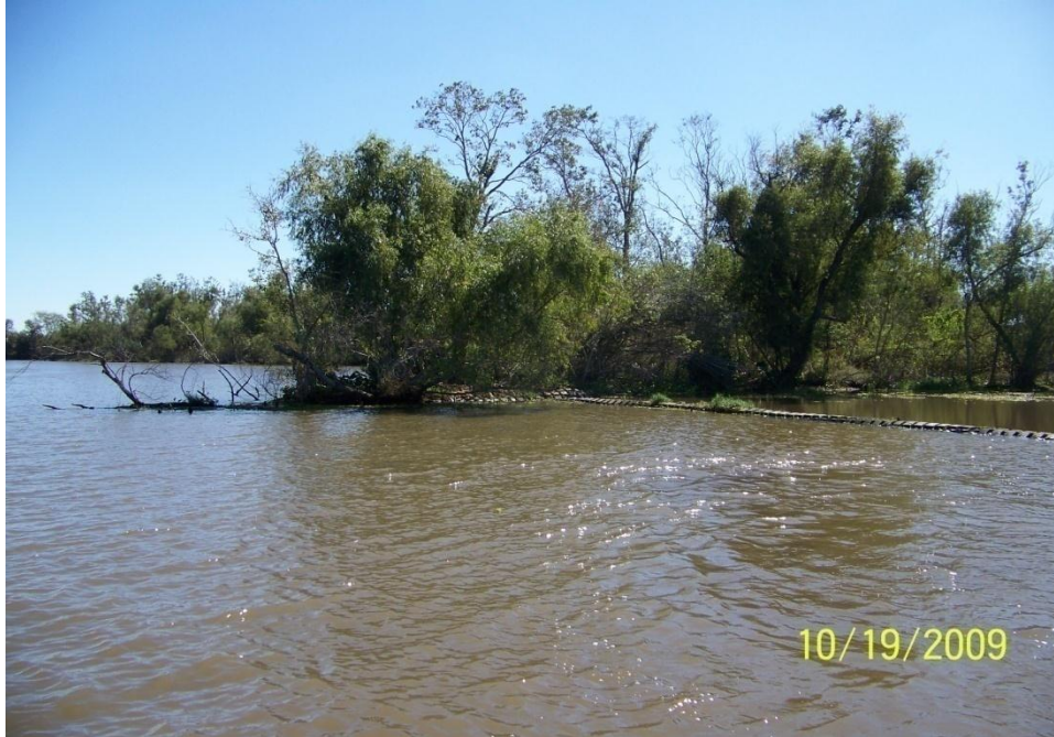
Photo No. 51 – Site R1 – elevated shoreline system tie-in to bank on east side of structure.
