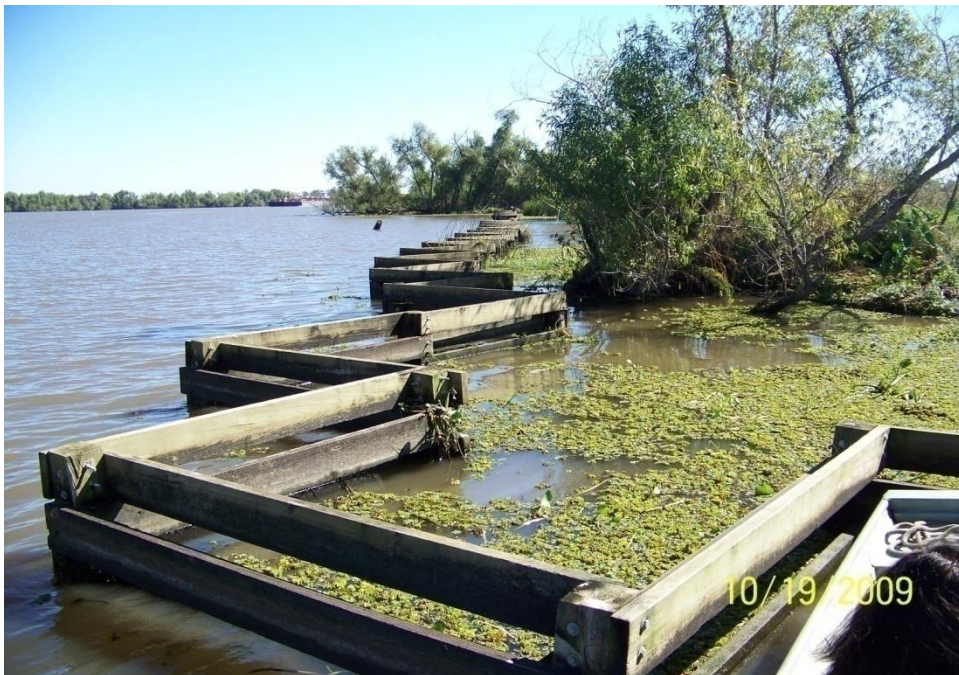
Photo No.30 – Site F2 – Timber fence treatment looking east.
