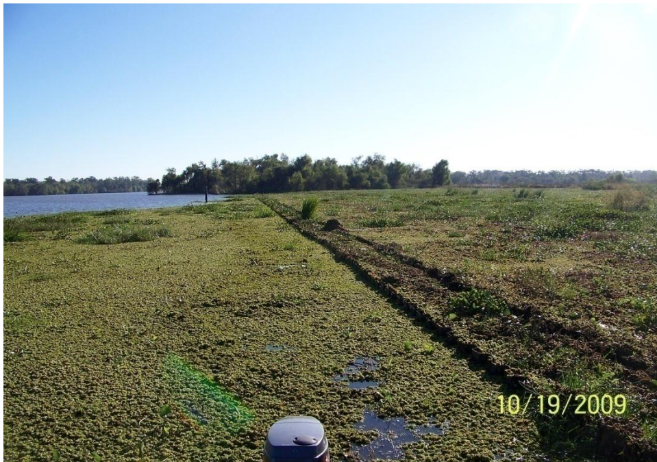
Photo No.4 – Site V3 – view of fiberglass sheet pile (double) wall structure looking east.
