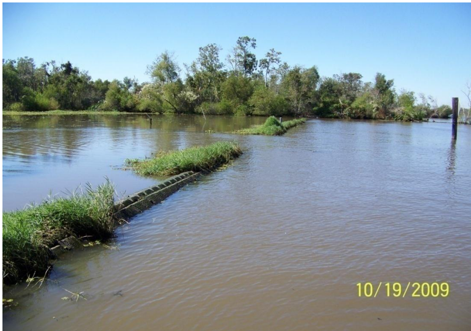
Photo No.58 – Site R2 – view of settled areas long the elevated shoreline system looking west.
