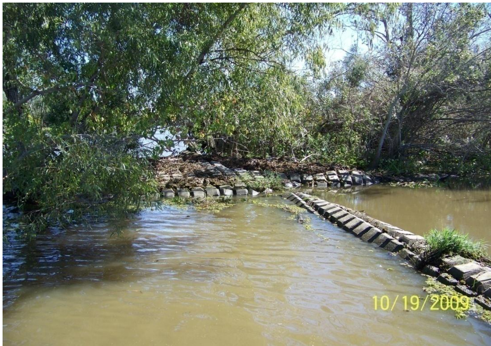
Photo No.52 – Site R1 – elevated shoreline system tie-in to bank on the east side of structure.
