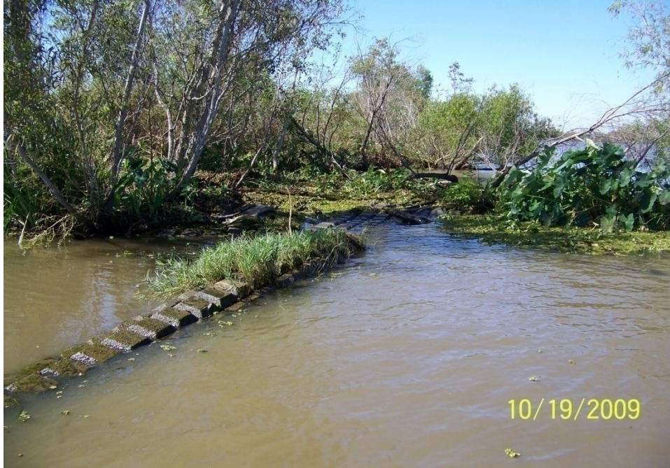
Photo No.49 – Site R1 – elevated system tie-in to bank on the west side of structure.
