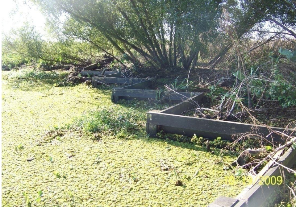
Photo No.19 – Site F3 – view of the timber fence structure along south bank line of GIWW.
