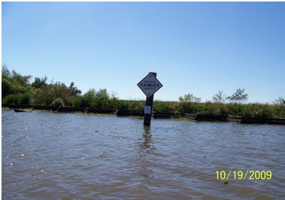
Photo No.38 – Site F1 – warning sign and timber fencing unit along south bank of GIWW.
