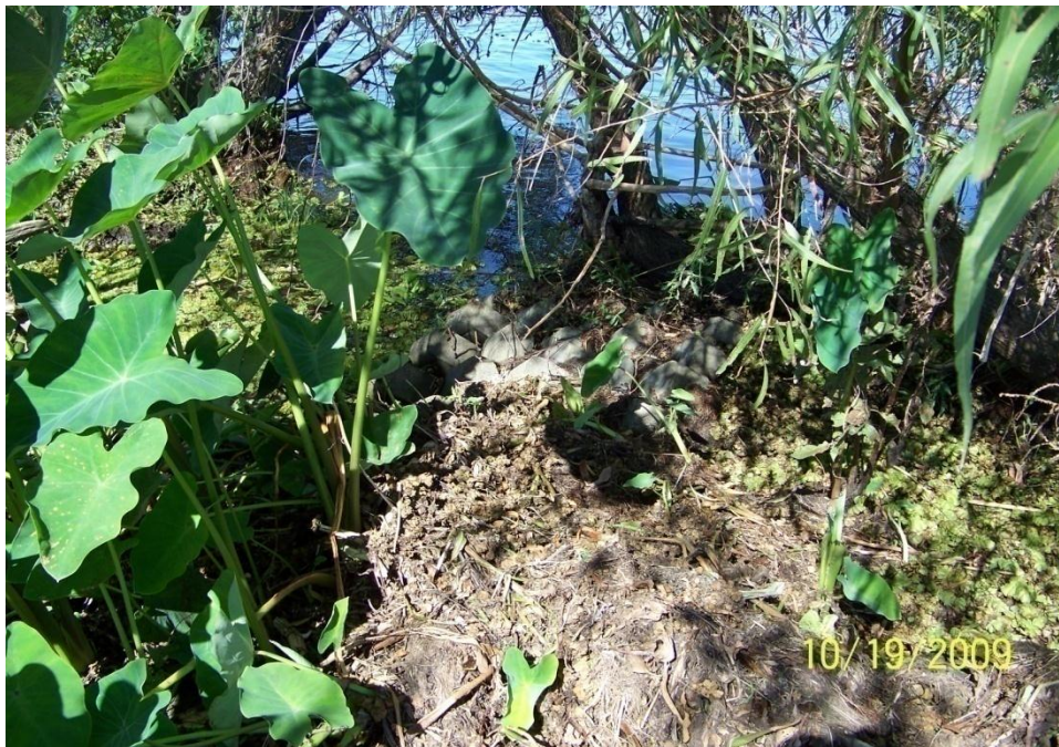
Photo No. 28 – Site J3 – Double row A-Jacks near bank tie-in.
