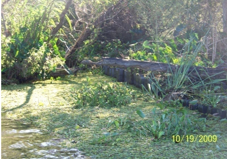
Photo No.15 – Site V2 – fiberglass sheet pile wall tie-in to bank on the east end of the structure.
