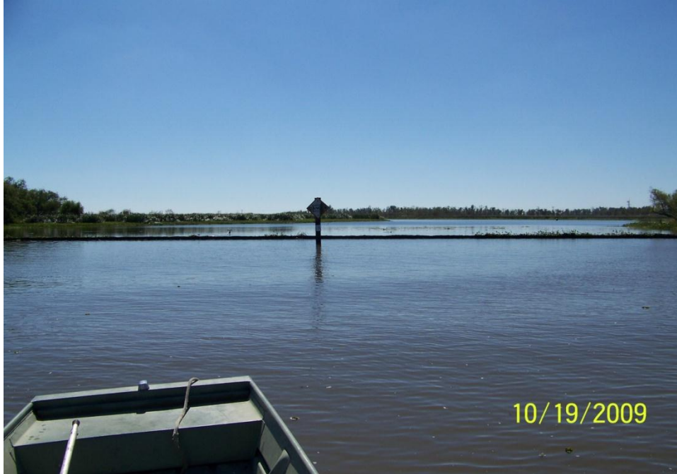
Photo No. 59 – Site V1 – view of warning sign in front of fiberglass sheet pile double wall.
