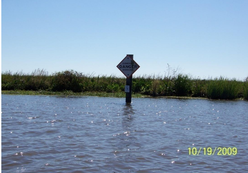
Photo No.27 – Site J3 – Double row A-Jacks units along the shoreline below water surface.
