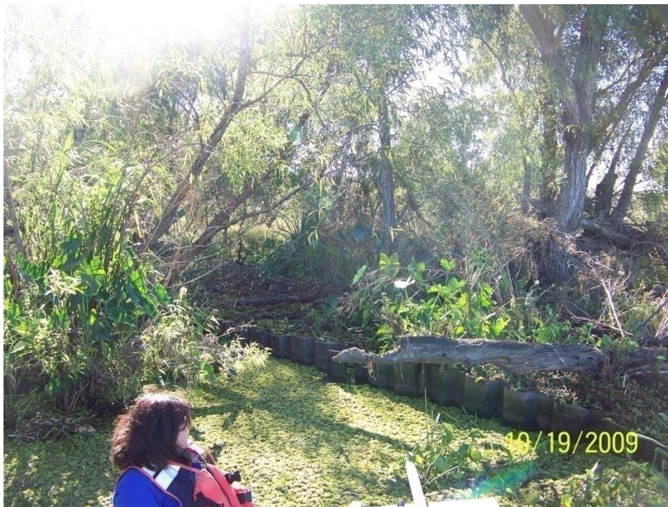
Photo No.16 - V2 - fiberglass sheet pile wall tie-in to bank on the east end of the structure.
