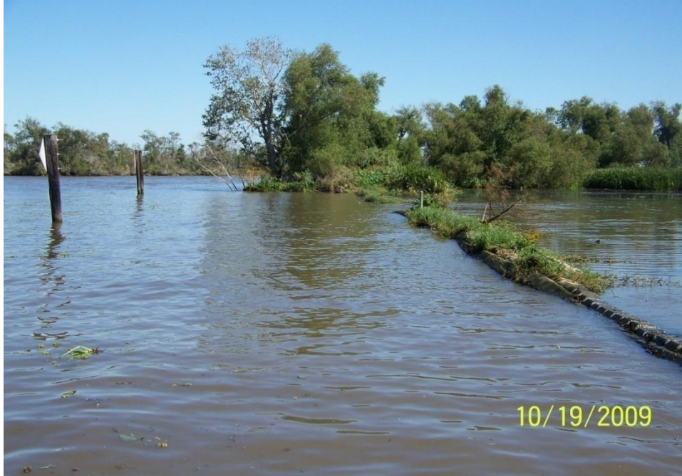
Photo No.67 – Site R1 – elevated shoreline system (revetment & CPE) looking eastward.
