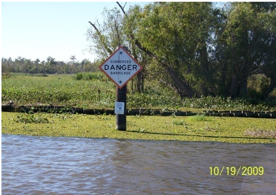
Photo No.12 – Site V2 –warning sign on north side of the fiberglass sheet pile (double) wall.
