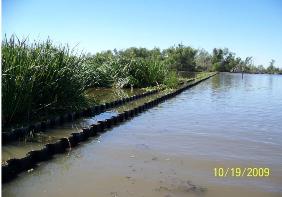
Photo No.63 – Site V1 – fiberglass sheet pile double wall looking westward.
