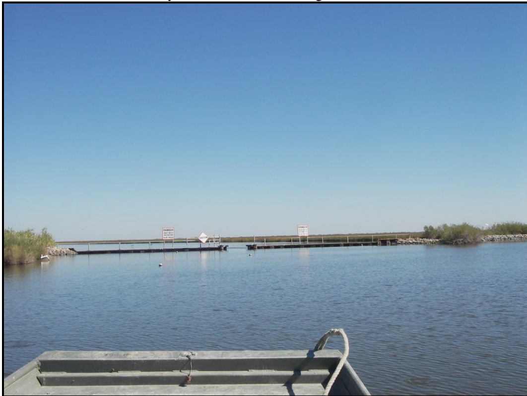
Photo 4 , Mangrove Weir, view looking north.
