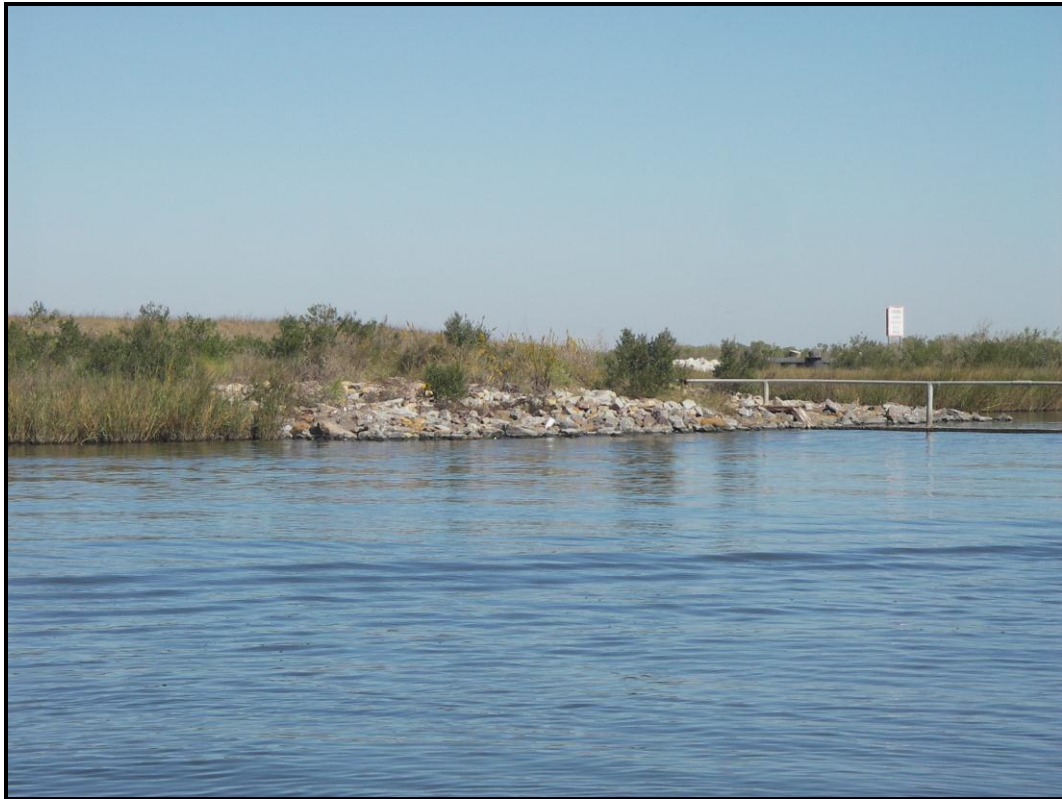
Photo 3 , Grand Bayou Weir, view showing rock armor on west side.
