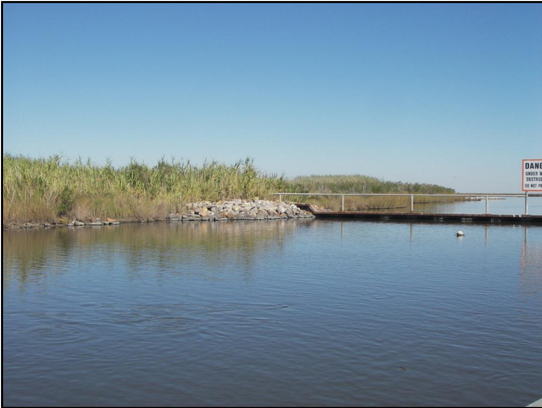
Photo No. 5, Mangrove Weir, view of rock armor west side.
