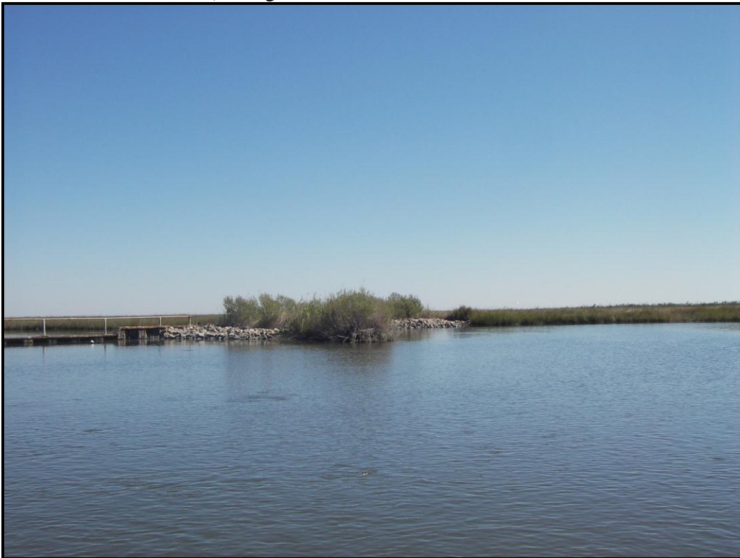
Photo No. 6, Mangrove Weir, view of sheet pile wall.
