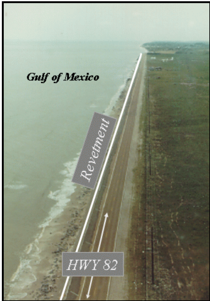
Figure 3. Aerial view of La. Hwy. 82 adjacent to the revetment installed by the La. Dept. of Transportation and Development during the 1970's. Image from Underwood et al. (1999).
