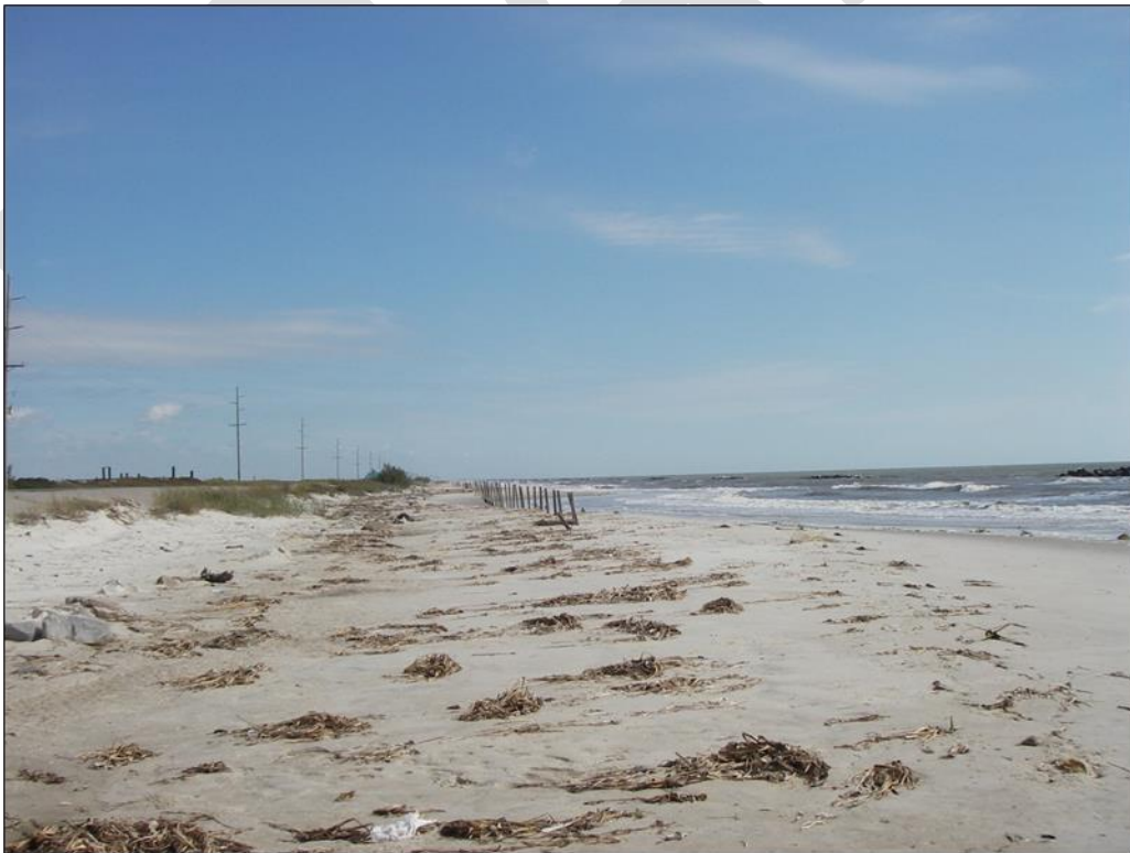
Photo No. 4 , Little to no sand fence remains on the eastern end of the project.
