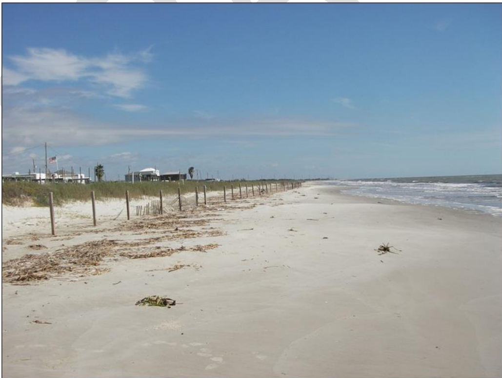
Photo No. 2, Double section of sand fence on western end of project. The section of fence closest to the water is no longer intact, due to tidal action, while the section further away from the water has successfully created a dune.
