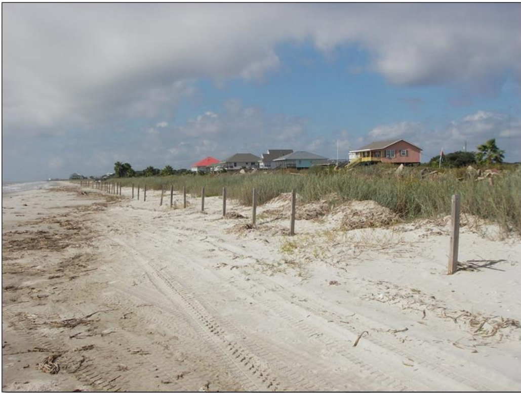
Photo No. 1, Double section of sand fence on western end of project. The section of fence closest to the water is no longer intact, due to tidal action, while the section further away from the water has successfully created a dune.
