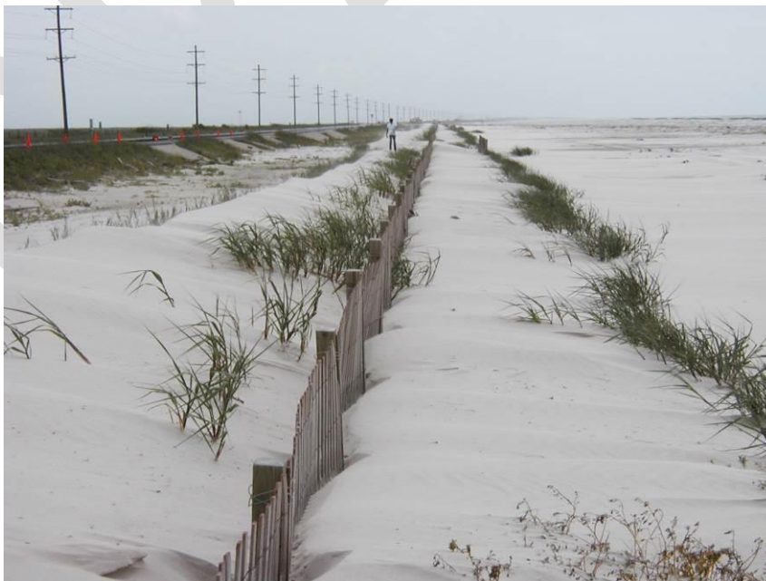
Figure 8a. View of the sand fencing and Vegetation Plantings at Station CS31-108 taken in April 2004. Note the dune formation almost covering the fences. The photograph is facing east.
