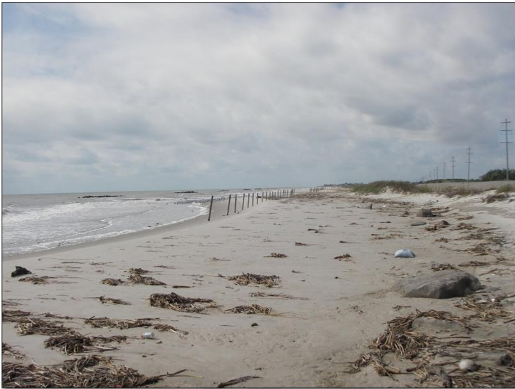
Photo No. 3 , Little to no sand fence remains on the eastern end of the project.
