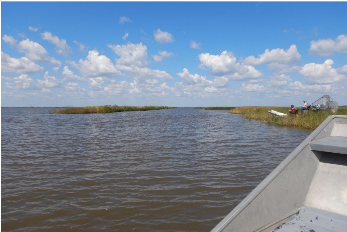
Photo No. 6 , Marsh Creation Cycle No. 5 – West side containment dike
