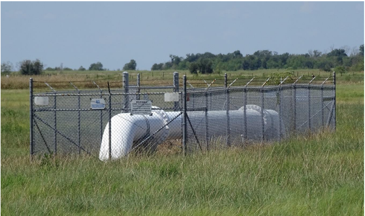
Photo No. 8, East Booster Station – looking Southwest
