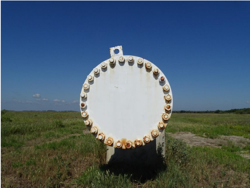
Photo No. 1, East end blind flange and riser (looking West)
