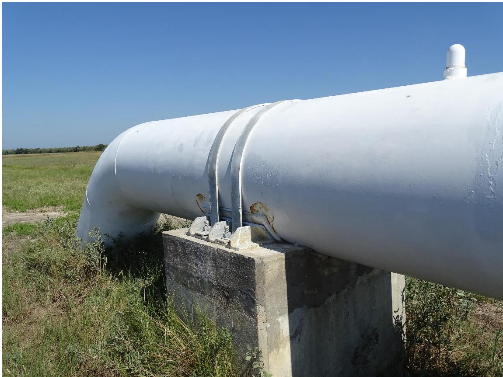
Photo No. 2, East end blind flange and riser (looking Northwest)
