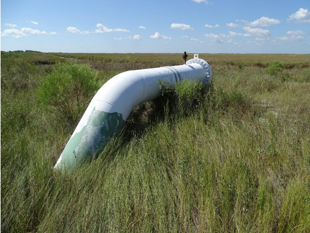
Photo No. 17 West Blind Flange and Riser looking South West
