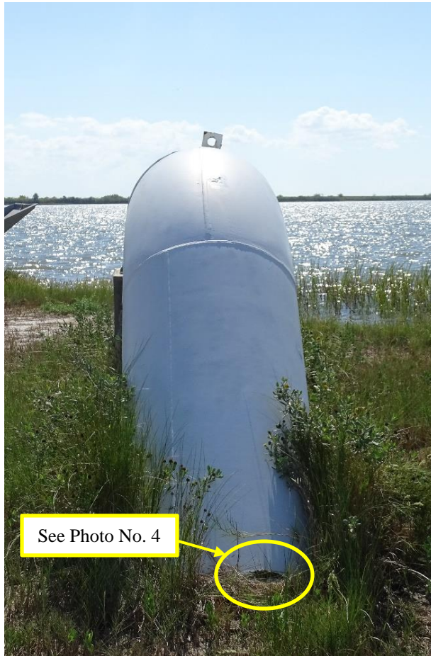
Photo No. 3, East end blind flange and riser (looking East)
