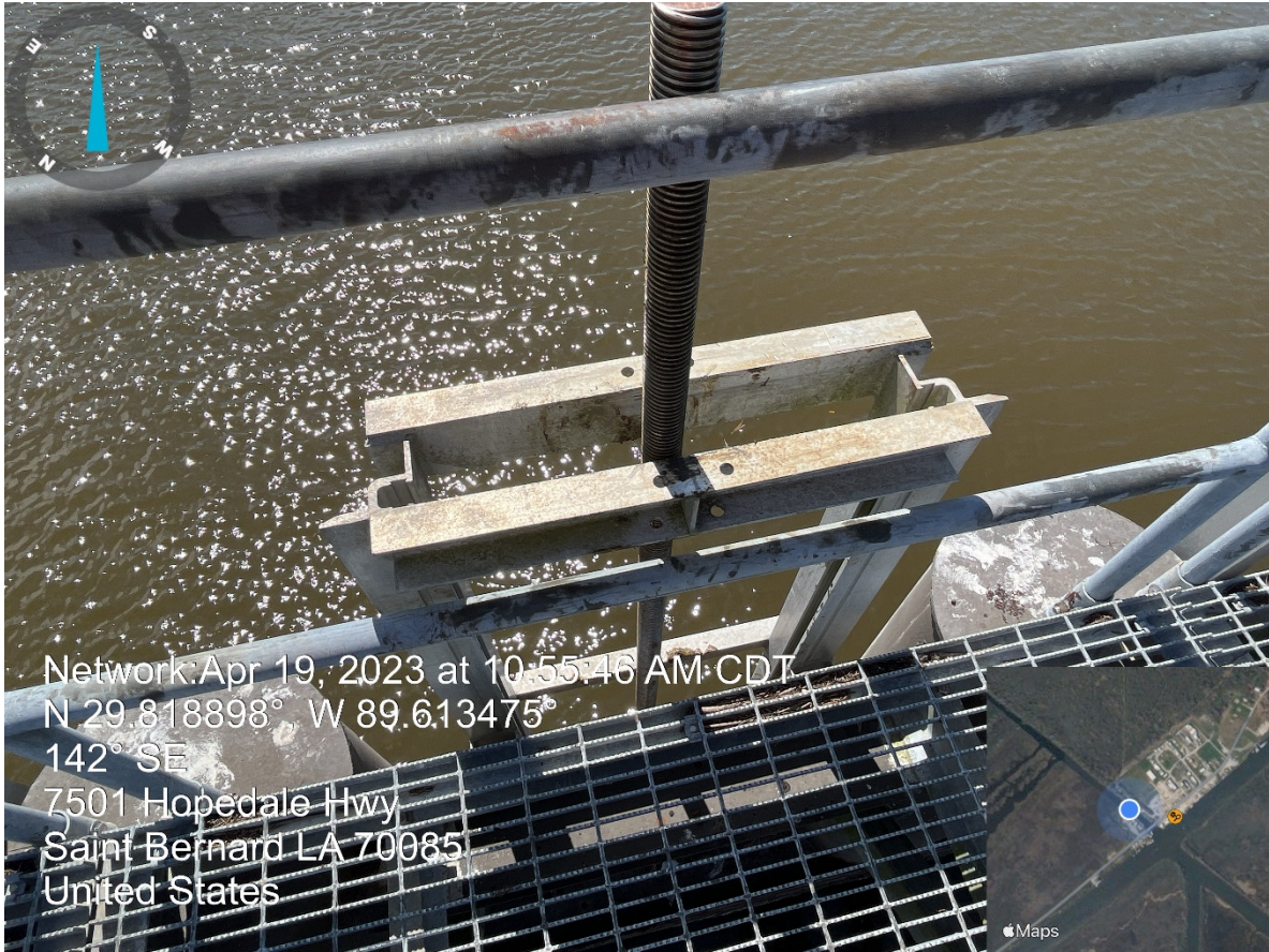
Photo 3: Fish gate viewed from atop the structure. (Gearbox removed for repairs).
