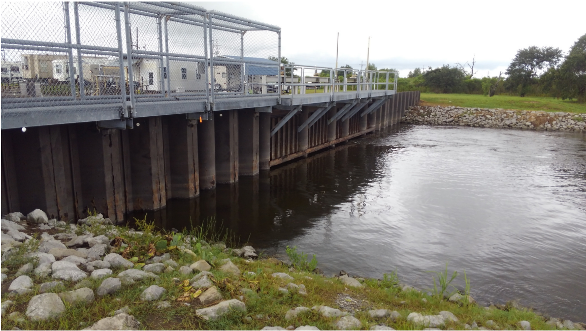
Photo 1: Structure taken from Upstream Northeast Bank looking south
