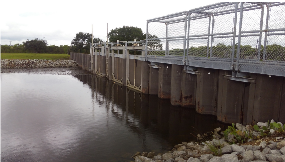
Photo 2: Gates taken from Downstream Northeast Bank looking west
