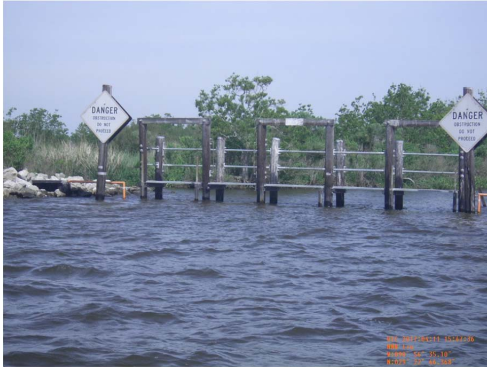
Photo No.23 – view of the variable crest weir Structure 21.
