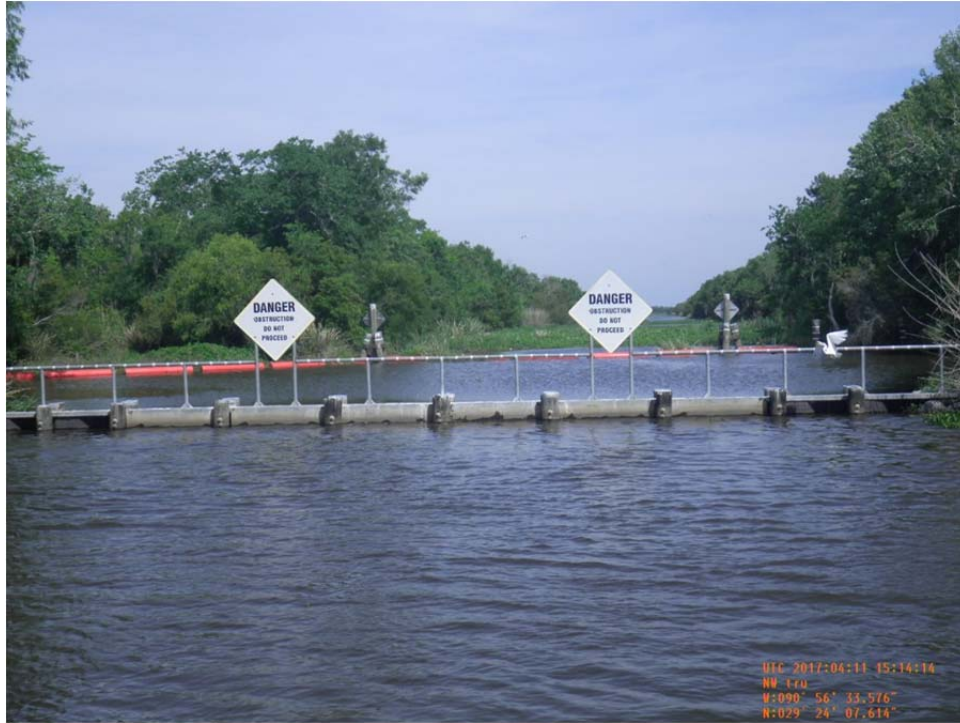
Photo No.21 – view of the Superior Canal Structure from the south side looking north.
