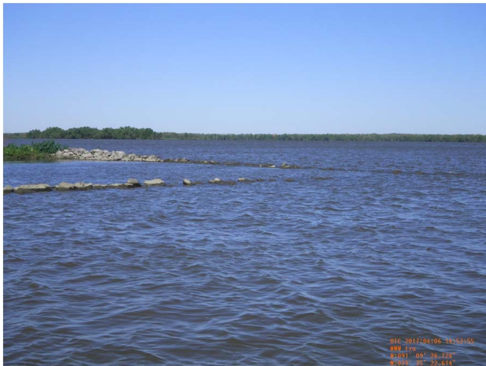
Photo No.8 – view of rock dike and marsh creation site on west side of Bayou Penchant at the intersection of Bayou Chene.
