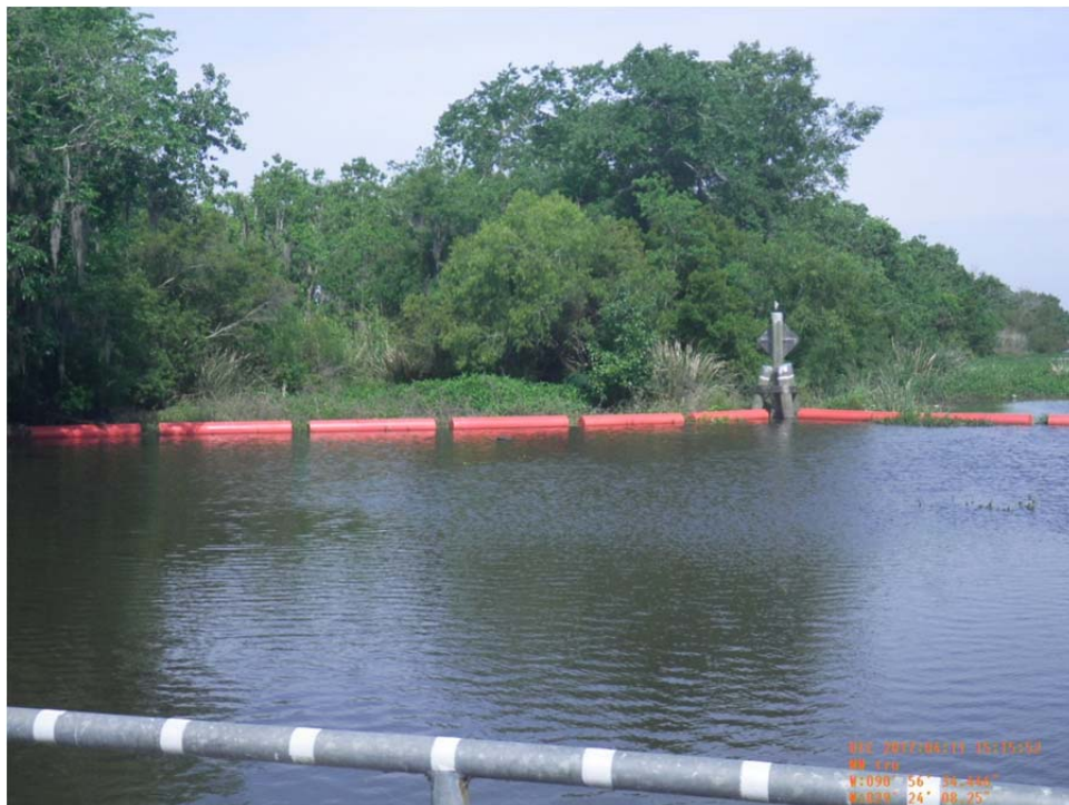
Photo No.22 – view of the floating debris barrier on the north side of the Superior Canal Structure.
