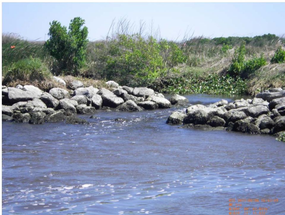
Photo 38- view of cut in rock dike tie-in on the north side steel sheetpile Weir No.5 along west bank of Bayou de Cade.
