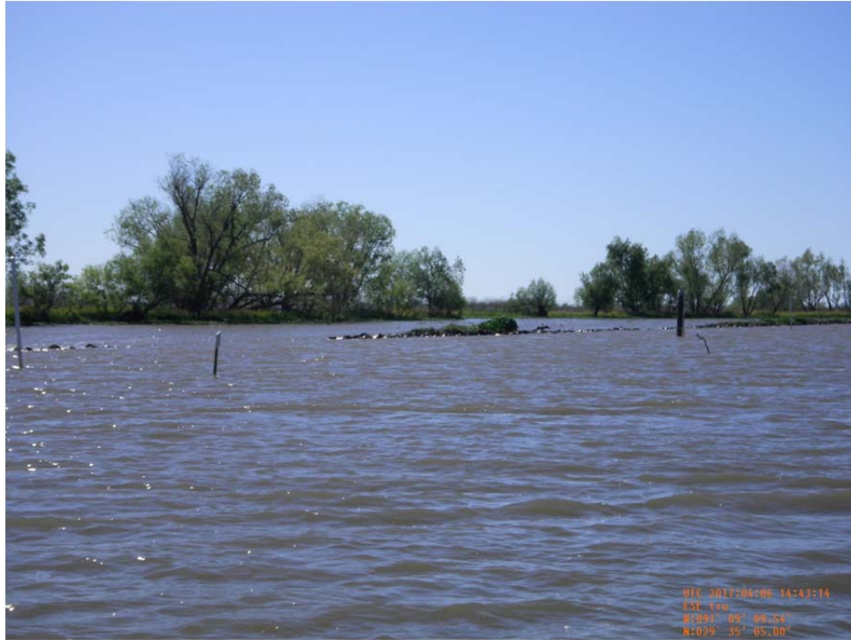
Photo No.3 – view of rock dike and marsh creation site along east bank of Bayou Penchant.
