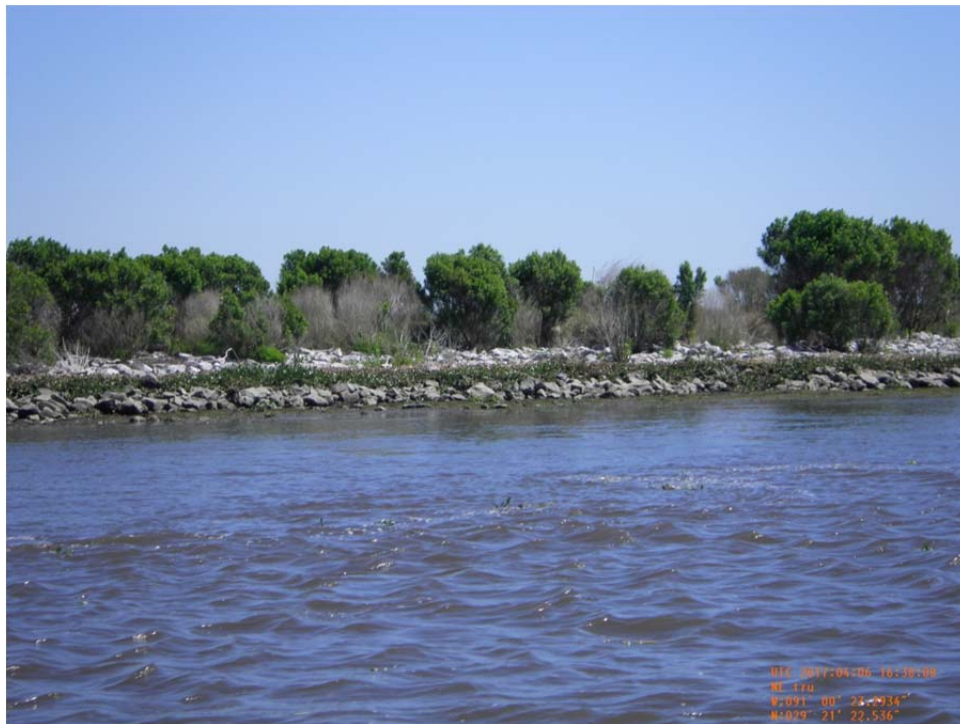
Photo 32- view of rock revetment (Reach 2) along west bank of Bayou de Cade.
