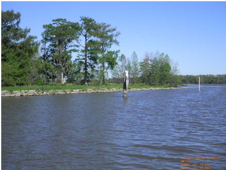
Photo No.6 – view of rock dike and marsh creation site on the west side of Bayou Penchant.
