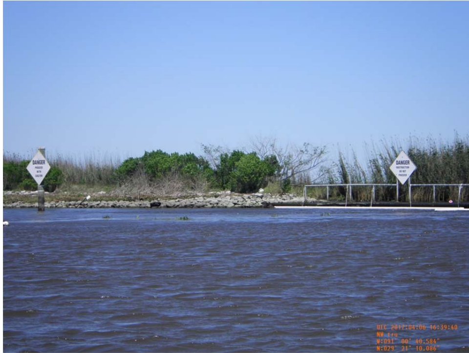
Photo 35- view of south bank tie-in of steel sheetpile Weir No.5 along west bank of Bayou de Cade.
