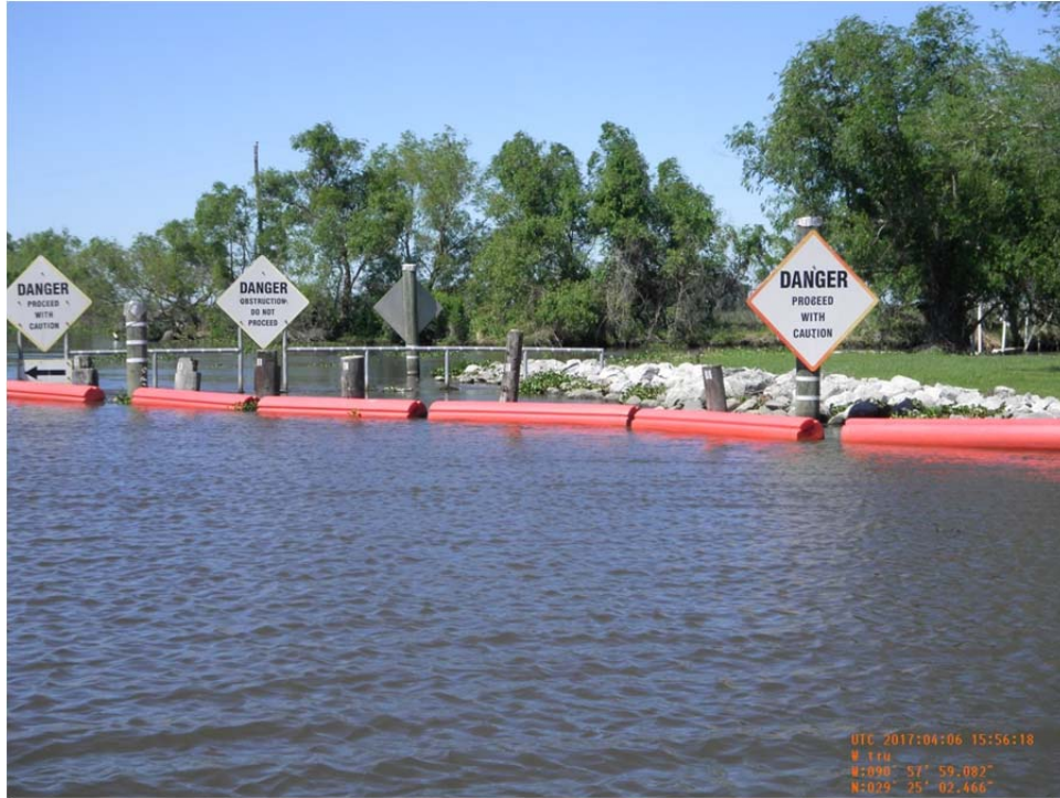
Photo No.15 – view of Brady Canal Structure, debris buoys and warning signs on northwest side of structure.
