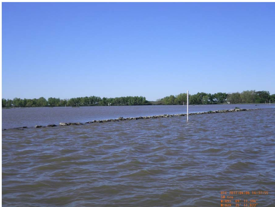
Photo No.2 – view of rock dike and marsh creation site on east side of Bayou Penchant along Bayou Chene.
