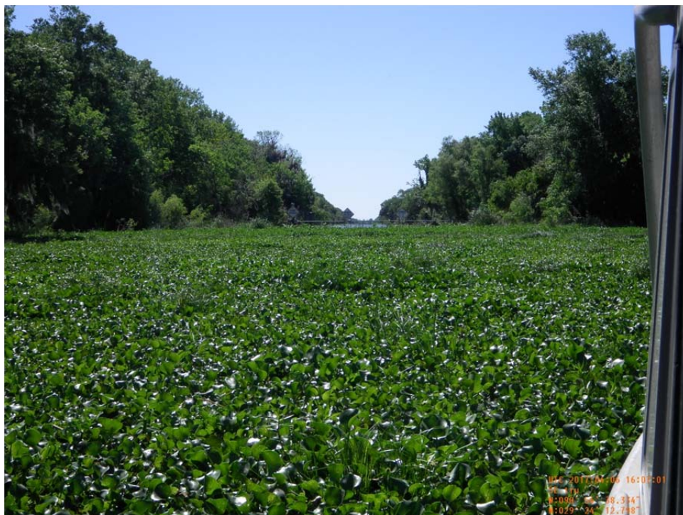
Photo No.18 – view of Superior Canal on the north side of the Superior Canal structure showing vegetation that is being held back by the floating debris barrier.
