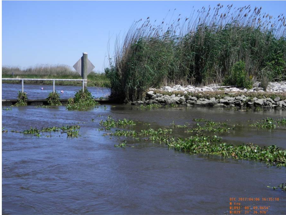
Photo 31- view of north bank tie-in of steel sheetpile Weir No.4 along west bank of Bayou de Cade.
