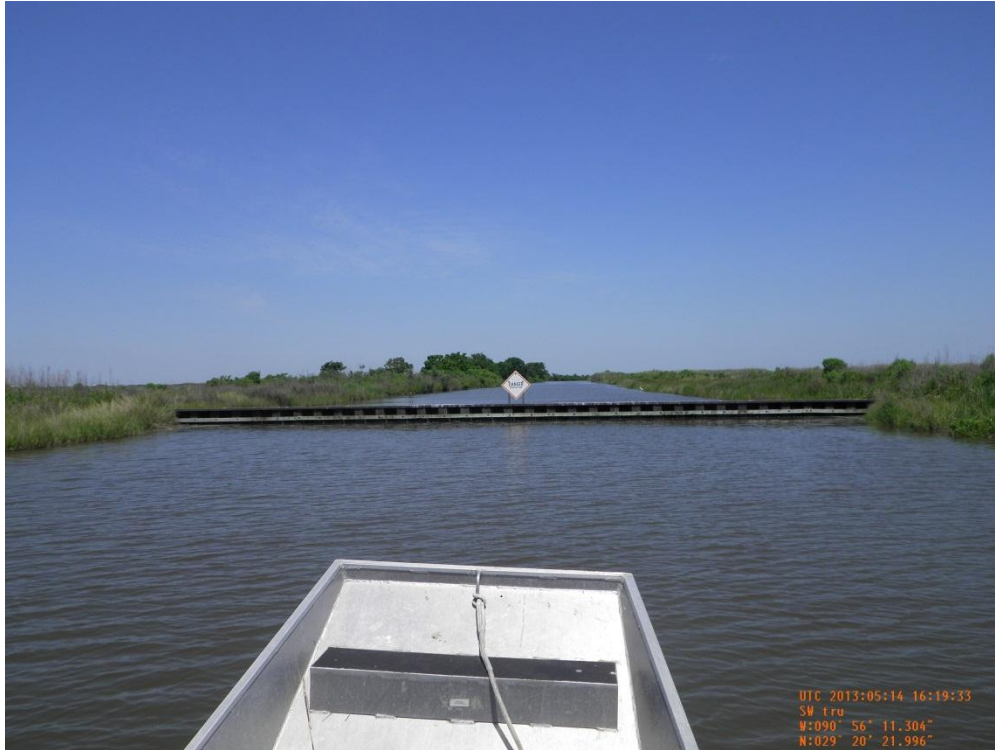
Photo 13: Overall view of Sheetpile Plug 3, looking northwest
