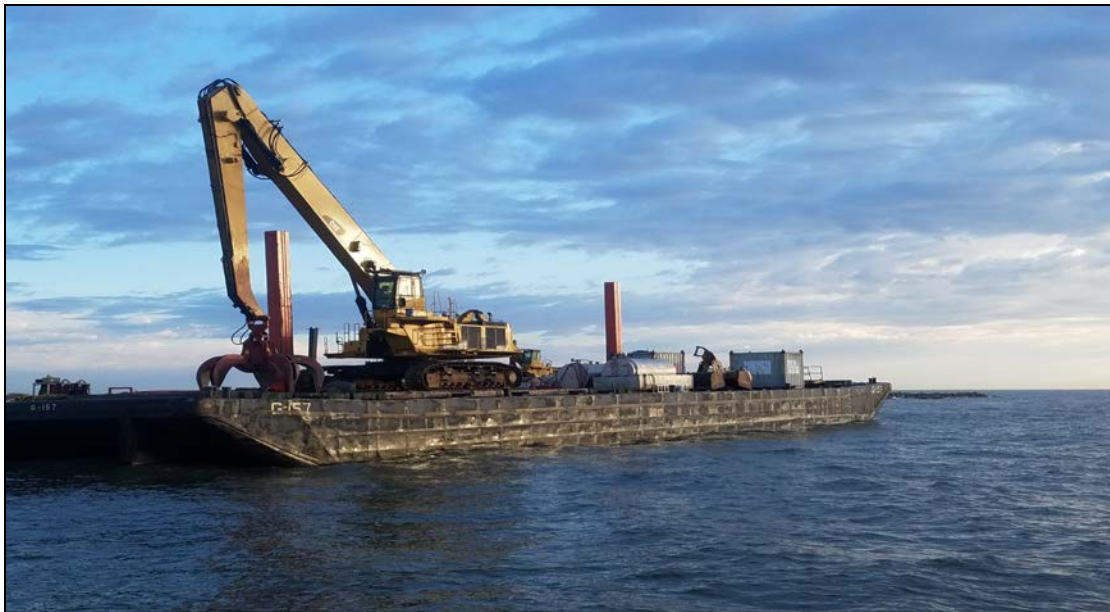
Figure 2: Major equipment mobilized to the project site
