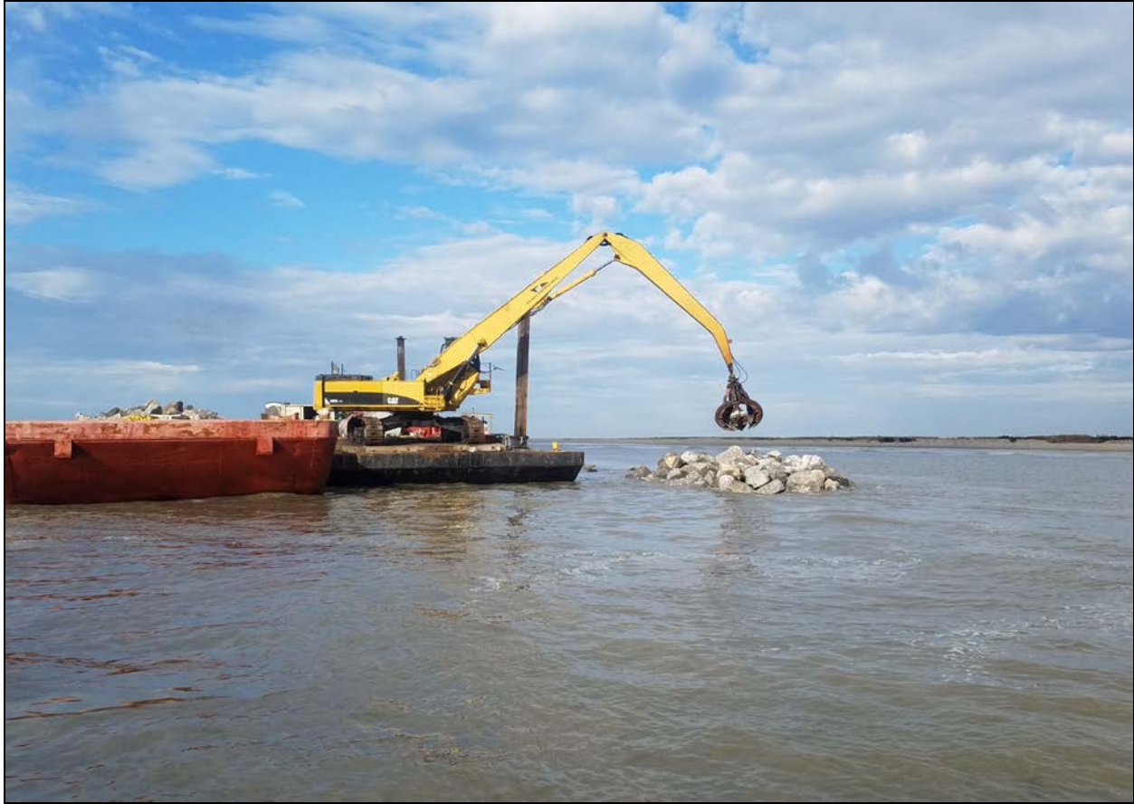
Figure 4: Typical Armor Stone Installation
