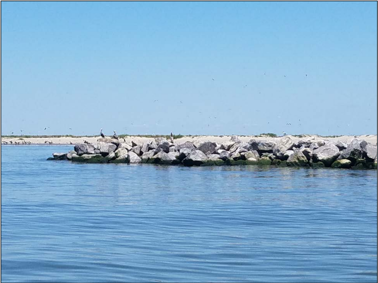
Figure 6: View of Breakwater 2 – Post-Construction
