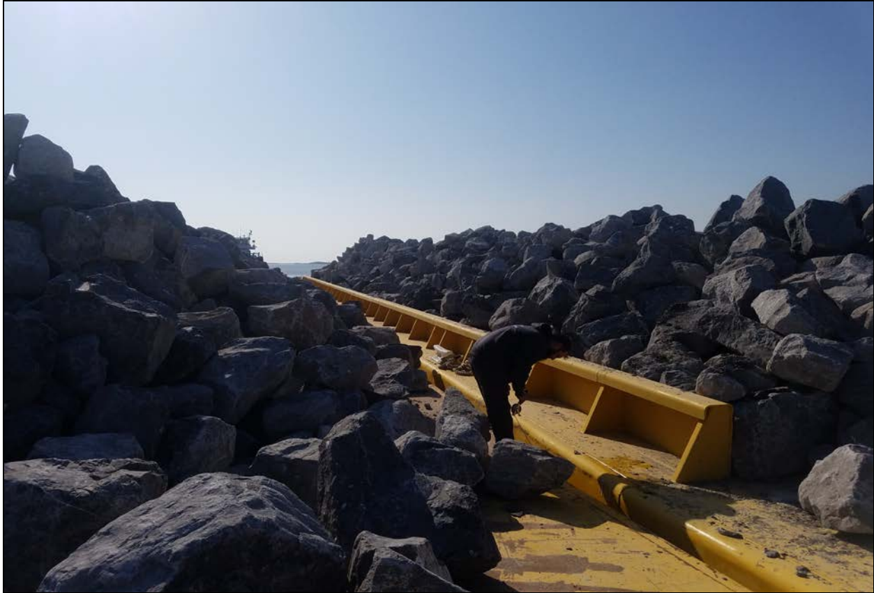
Figure 5: Draft Surveys on Fully Loaded Rock Barges
